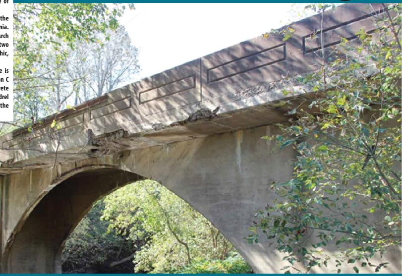
**Location:** Kanawha County Route 52 (New Hope Road) over Blue Creek **Type:** A Spandrel Braced Arch Bridge with Arch Ribs Supporting the Deck
