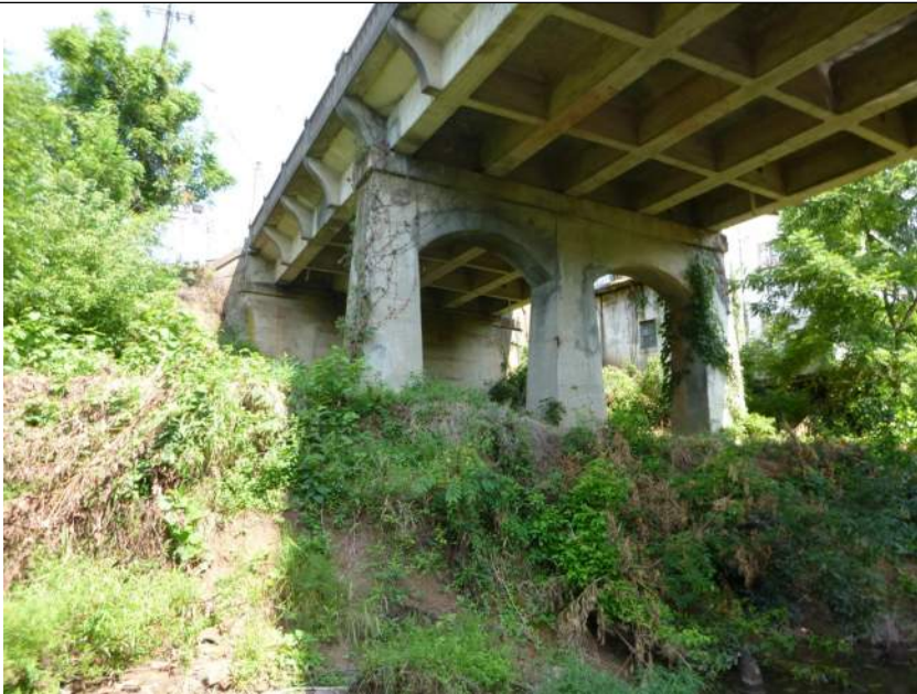
Photo #11 - View of underneath the bridge at abutment 1 & pier 4
