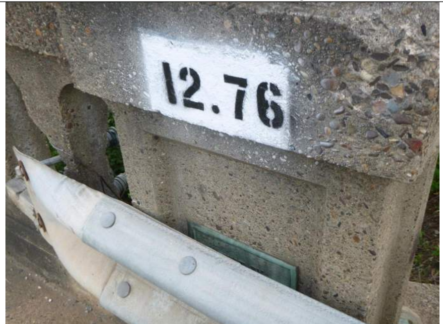
Photo #8 - Bridge milepost and builder plaque
