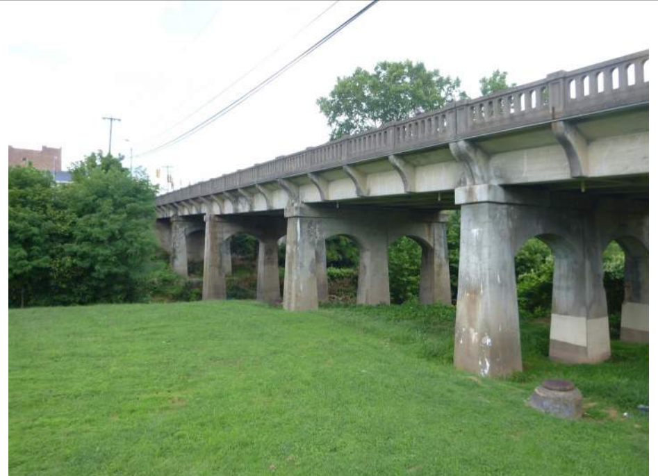
Photo #6 - Elevation view looking downstream
