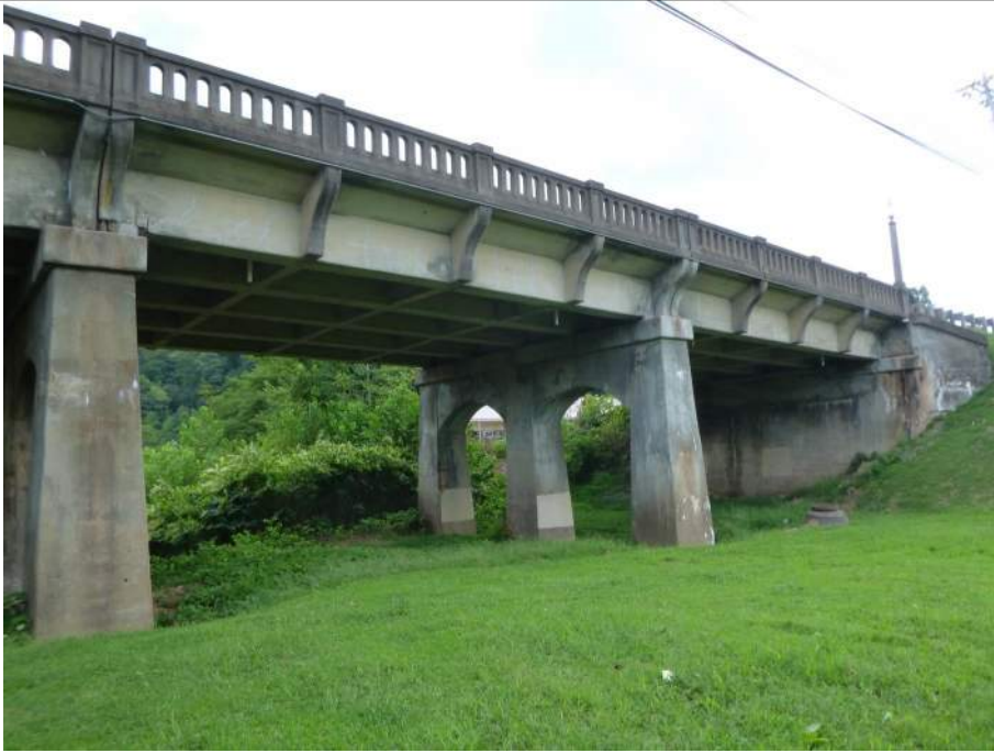
Photo #5 - Elevation view looking upstream
