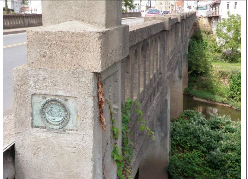
Photo #10 - Bridge plaque at abutment two
