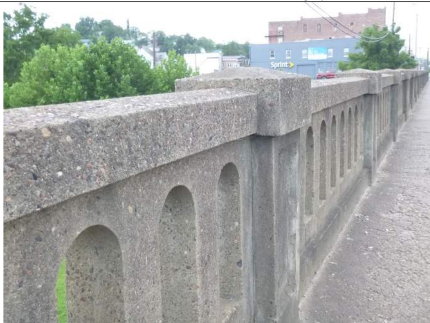
Photo #7 - Concrete parapet railing
