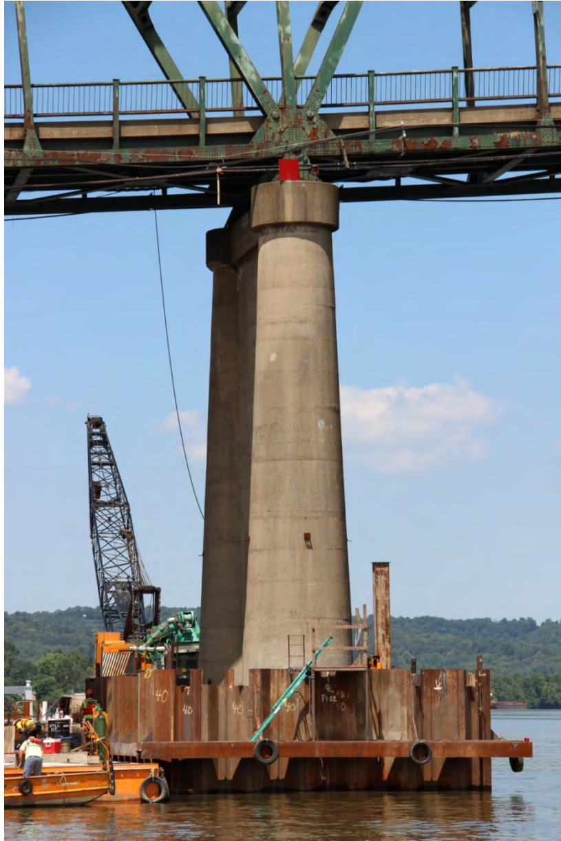
PHOTO 13 SOUTHEAST ELEVATION OF BRIDGE PIER NO. 2 SHOWING BRIDGE SHOE OF CANTILEVER TRUSS SPAN NOS. 6 AND 7, FACING NORTHWEST.
