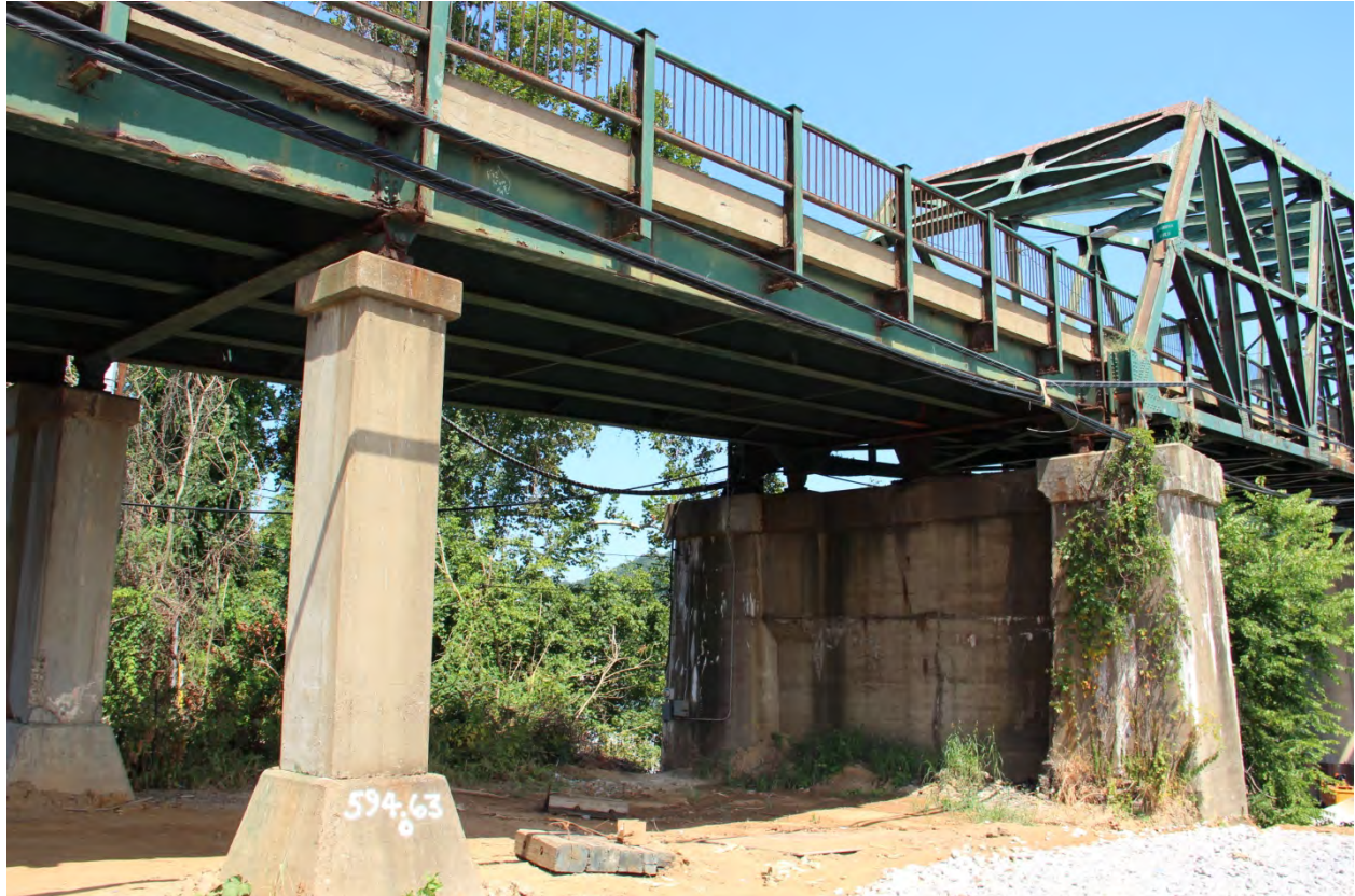
PHOTO 9 SOUTHEAST ELEVATION OF SOUTHWEST VIADUCT SPAN NO. 5 SHOWING VIADUCT PEDESTAL NO. 4 AND BRIDGE PIER NO. 1, FACING NORTH.
