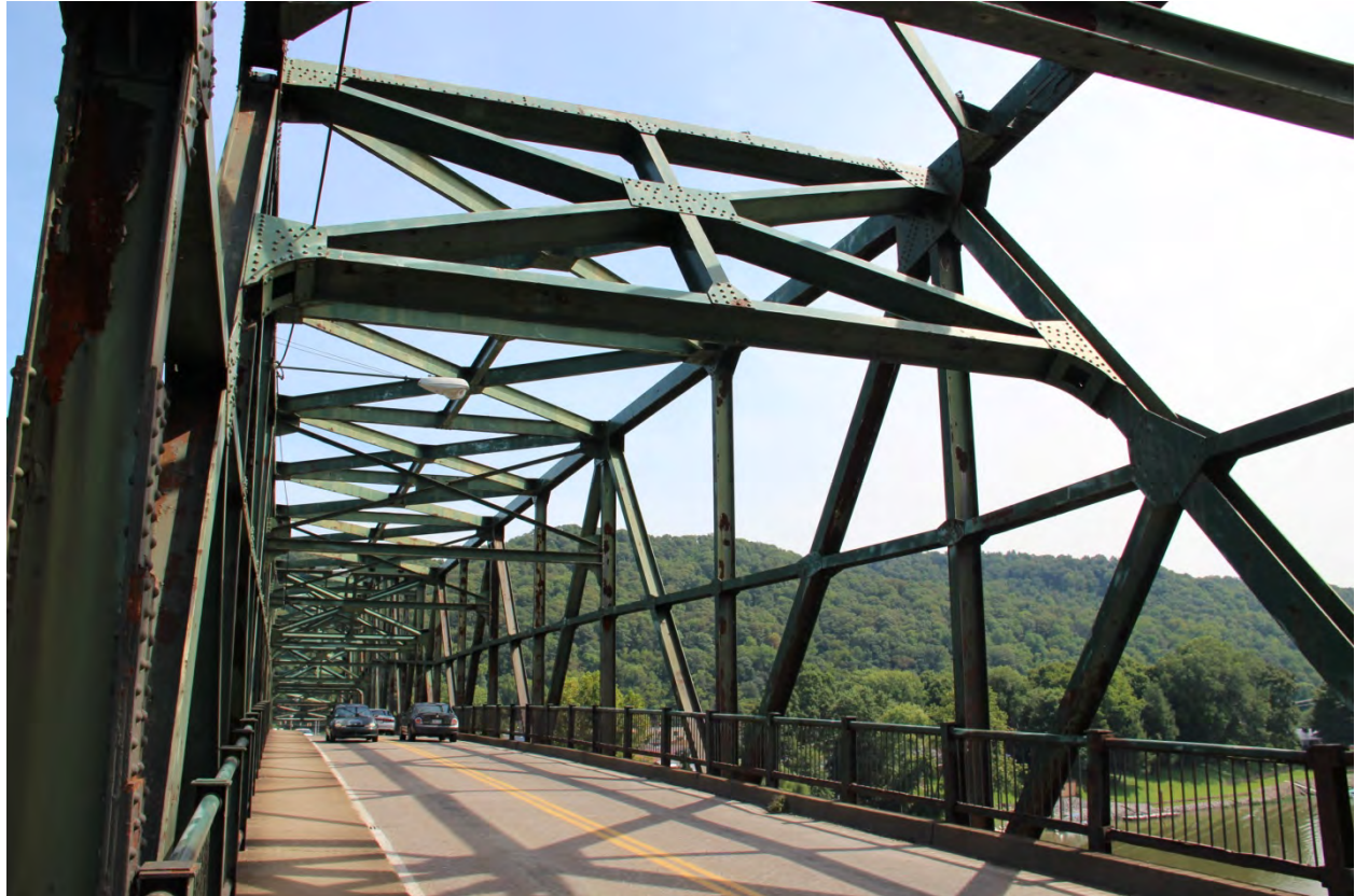
PHOTO 34 INTERIOR VIEW FROM DECK OF CENTER SUSPENDED PORTION OF TRUSS SPAN NO. 7 SHOWING BRIDGE DECK, VERTICAL AND DIAGONAL TRUSS MEMBERS, RIVETED CONNECTIONS, SWAY FRAMES, TOP CHORD, AND TOP LATERAL BRACING, FACING NORTHEAST.
