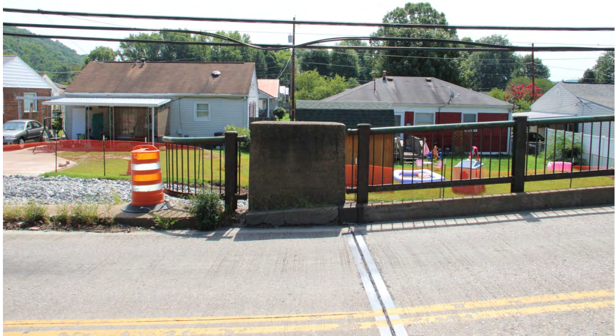
PHOTO 46 DETAIL OF HANDRAILING, POSTS, AND CONCRETE END POST ASSEMBLY ALONG SOUTHEAST ELEVATION OF NORTHWEST APPROACH, FACING SOUTHEAST.
