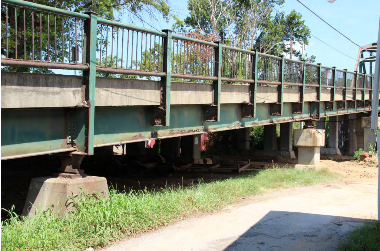
PHOTO 6 SOUTHEAST ELEVATION OF SOUTHWEST VIADUCT SPAN NO. 2 SHOWING VIADUCT PEDESTAL NOS. 1 AND 2, FACING NORTH.
