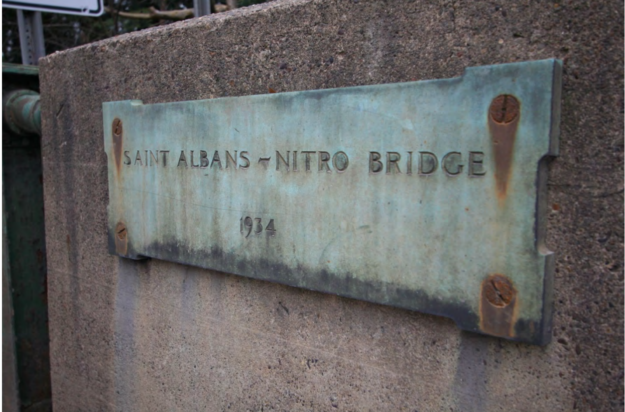
PHOTO 44 DETAIL OF CONCRETE END POST WITH BRIDGE PLAQUE ALONG NORTHWEST ELEVATION OF NORTHEAST APPROACH, FACING WEST.
