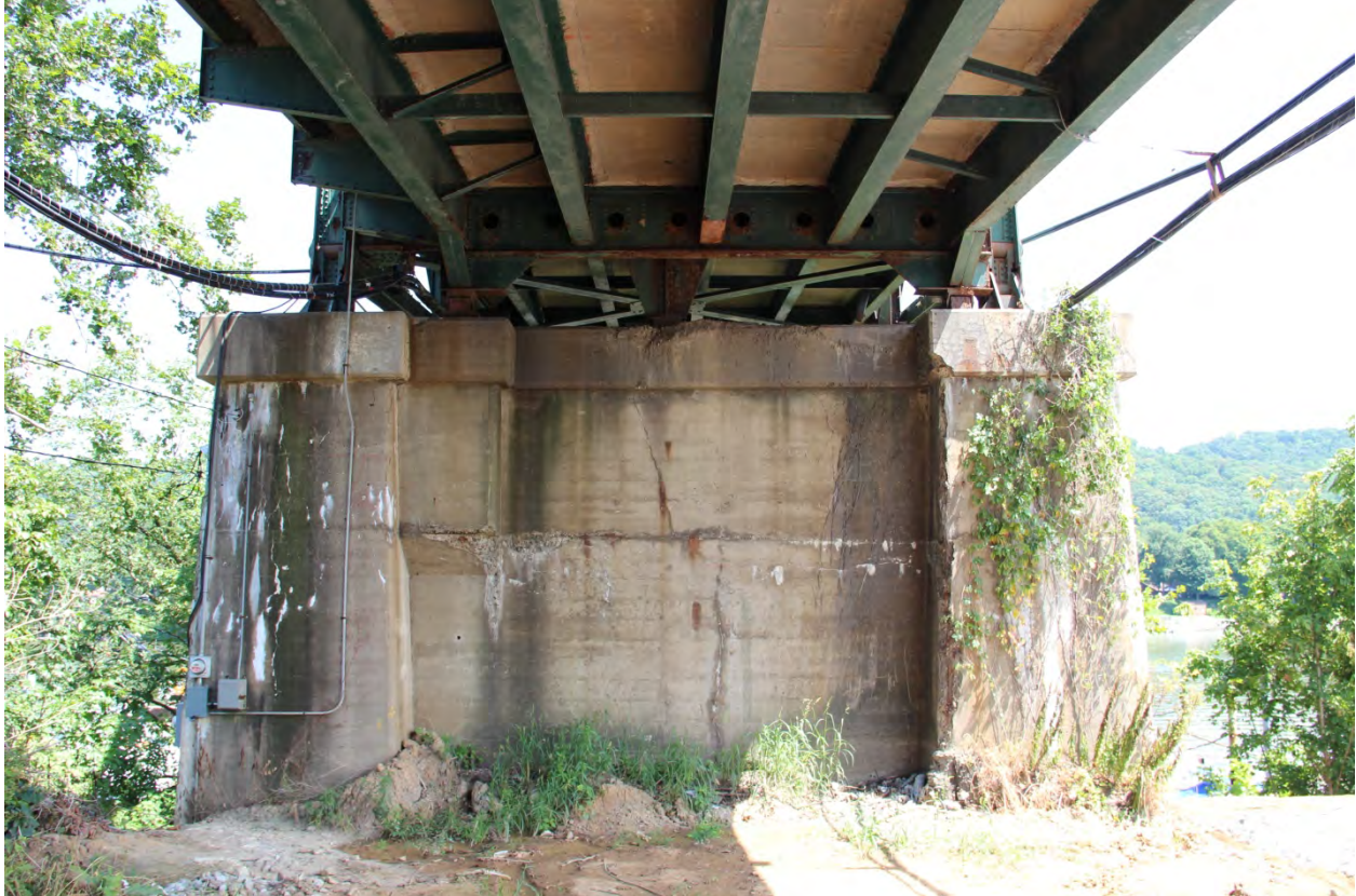
PHOTO 11 SOUTHWEST ELEVATION OF BRIDGE PIER NO. 1 SHOWING FLOORBEAMS, STRINGERS, AND ROCKER SHOES OF VIADUCT SPAN NO. 5 AND SHOES AND ANCHORAGE OF CANTILEVER TRUSS SPAN NO. 6, FACING NORTHEAST.
