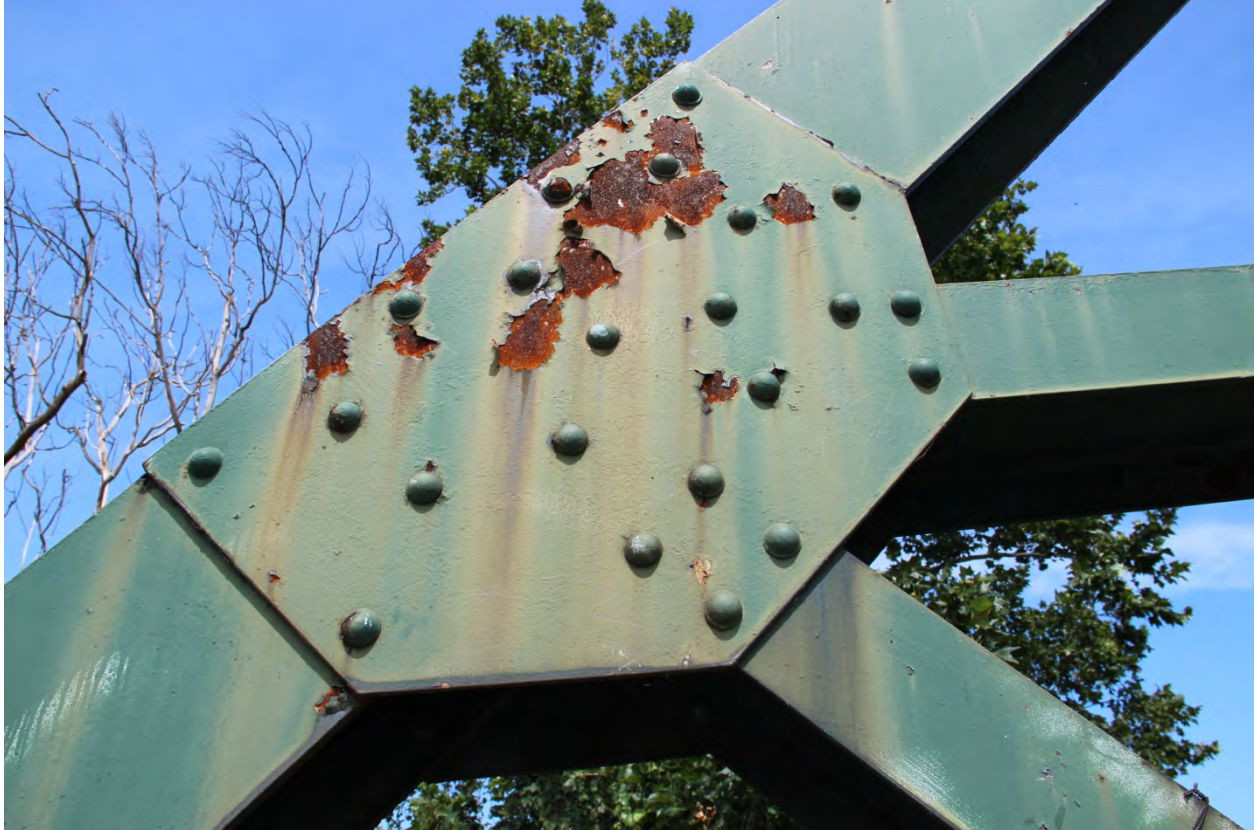
PHOTO 29 DETAIL OF RIVETED GUSSET PLATE ON INTERIOR OF NORTHWEST ELEVATION OF CANTILEVER TRUSS SPAN NO. 6 AT SOUTHWEST PORTAL.
