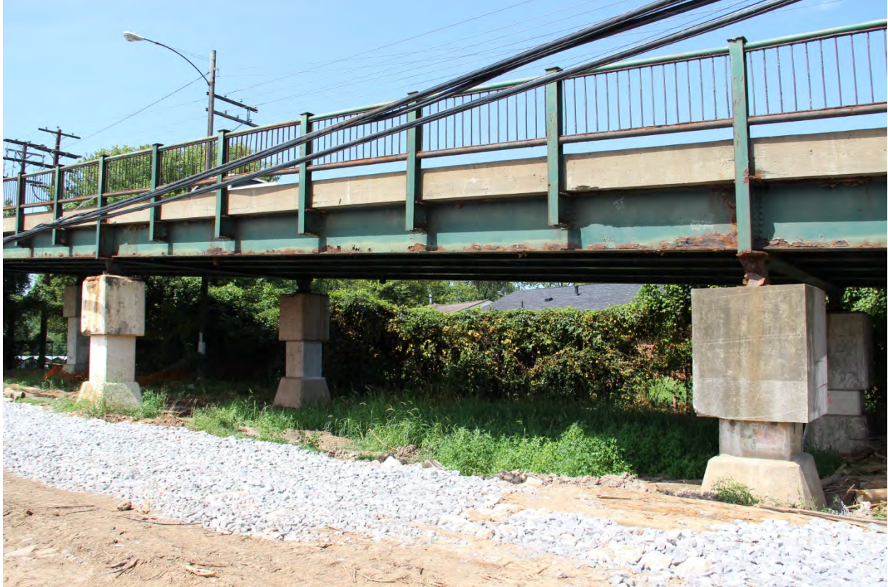
PHOTO 22 SOUTHEAST ELEVATION OF NORTHEAST VIADUCT SPAN NO. 12 SHOWING VIADUCT PEDESTAL NOS. 7 AND 8, FACING SOUTHWEST.
