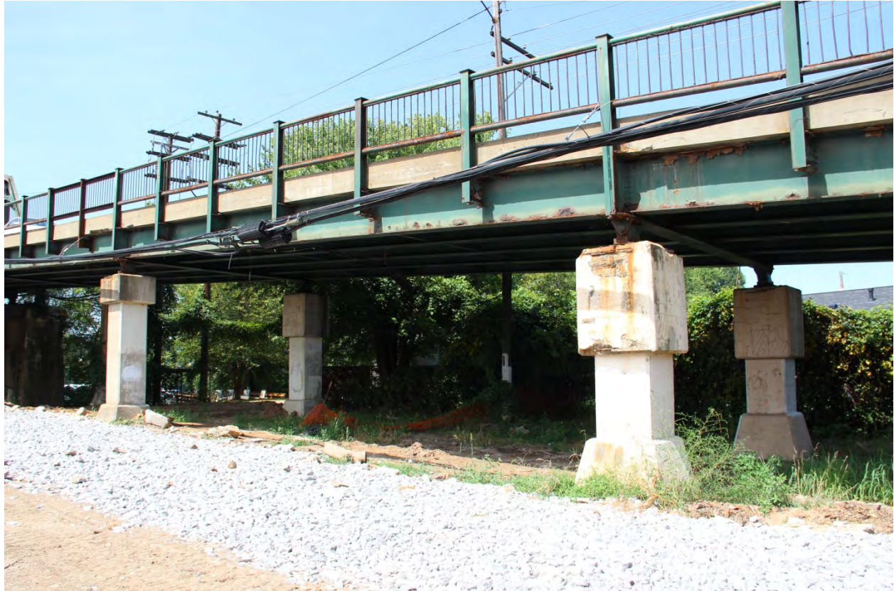
PHOTO 21 SOUTHEAST ELEVATION OF NORTHEAST VIADUCT SPAN NO. 11 SHOWING VIADUCT PEDESTAL NOS. 6 AND 7, FACING SOUTHWEST.
