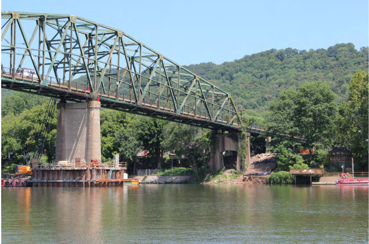
PHOTO 36 SOUTHEAST ELEVATION OF CANTILEVERED TRUSS SPAN NO. 8 BETWEEN BRIDGE PIER NOS. 3 AND 4 SHOWING BOTTOM CHORD, VERTICAL AND DIAGONAL MEMBERS, SWAY FRAMES, TOP CHORD, AND TOP LATERAL BRACING, FACING NORTHWEST.
