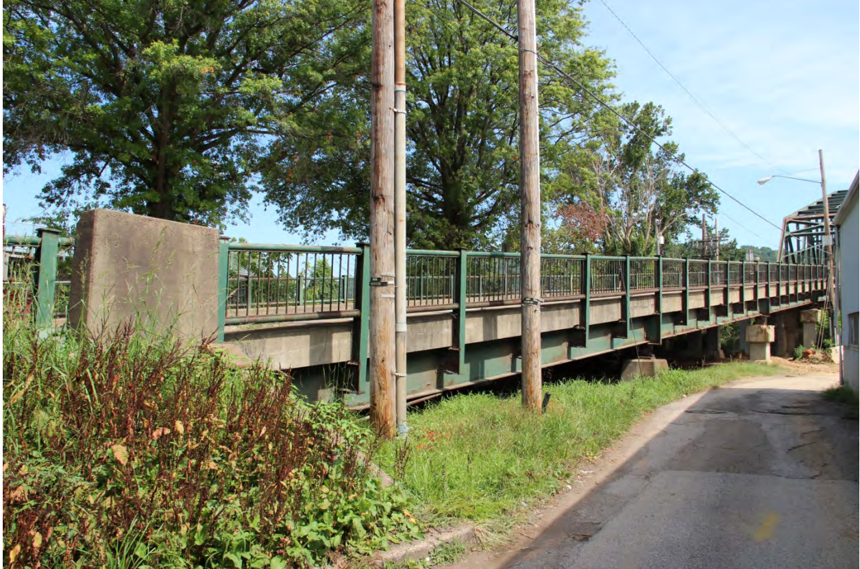
PHOTO 45 DETAIL OF HANDRAILING, POSTS, CONCRETE END POSTS, AND HANDRAIL SUPPORT BRACKETS ALONG SOUTHEAST ELEVATION OF SOUTHWEST APPROACH, FACING NORTH.
