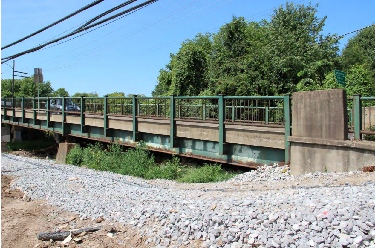
PHOTO 25 SOUTHEAST ELEVATION OF NORTHEAST VIADUCT SPAN NO. 14 SHOWING VIADUCT PEDESTAL NO. 9 AND NORTHEAST ABUTMENT, FACING SOUTHWEST.
