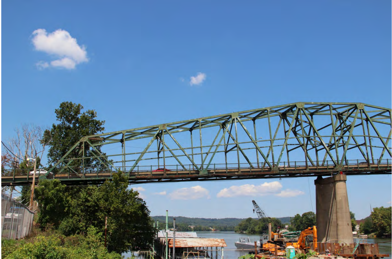
PHOTO 26 SOUTHEAST ELEVATION OF CANTILEVER TRUSS SPAN NO. 6 SHOWING BOTTOM CHORD, VERTICAL AND DIAGONAL MEMBERS, SWAY FRAMES, TOP LATERAL BRACING, AND TOP CHORD, FACING NORTHWEST.
