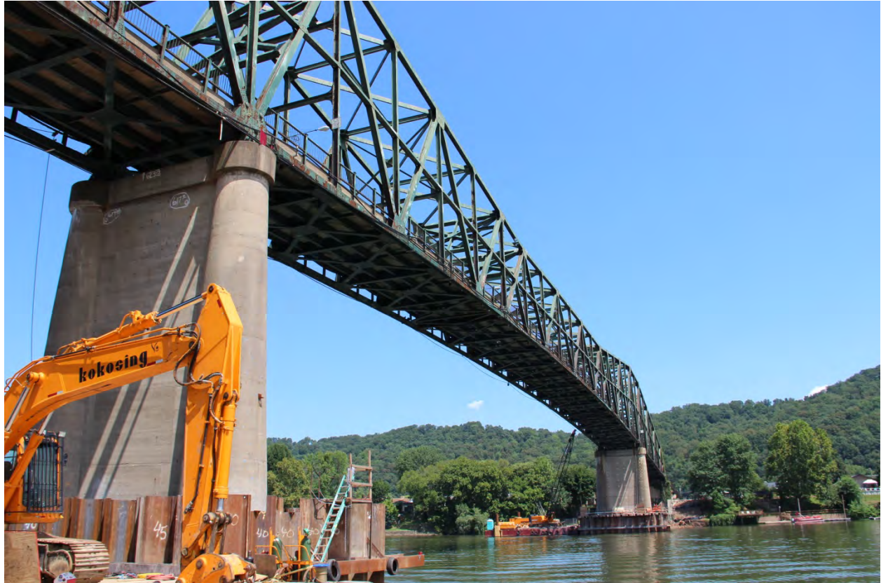
PHOTO 33 SOUTHEAST ELEVATION AND UNDERSIDE OF CANTILEVERED AND SUSPENDED TRUSS SPAN NO. 7 BETWEEN BRIDGE PIER NOS. 2 AND 3 SHOWING FLOOR SYSTEM, BOTTOM CHORD, VERTICAL AND DIAGONAL MEMBERS, SWAY FRAMES, TOP LATERAL BRACING, AND TOP CHORD, FACING NORTH.
