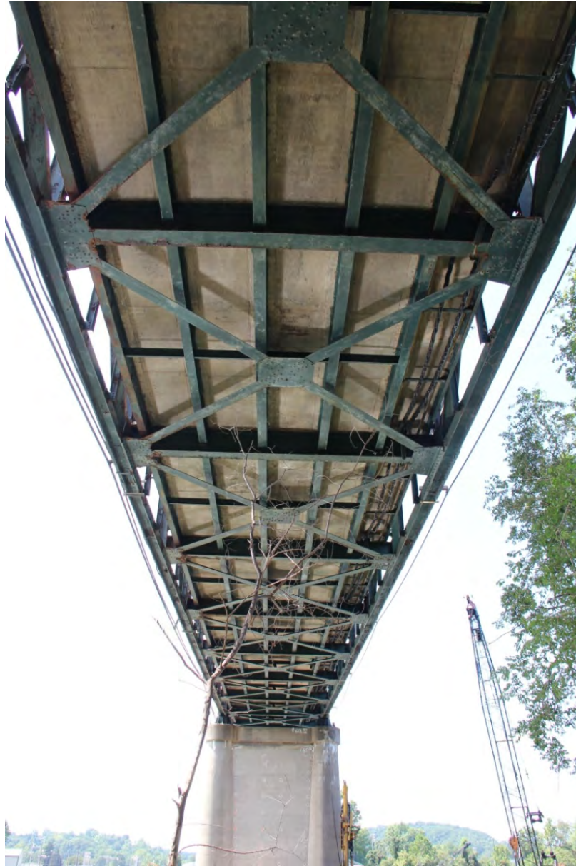
PHOTO 15 UNDERSIDE OF CANTILEVER TRUSS SPAN NO.8 SHOWING BOTTOM CHORD AND FLOOR SYSTEM CONSISTING FLOOR BEAMS, STRINGERS, AND BOTTOM LATERAL BRACING WITH BRIDGE PIER NO. 3 IN BACKGROUND, FACING SOUTHWEST.
