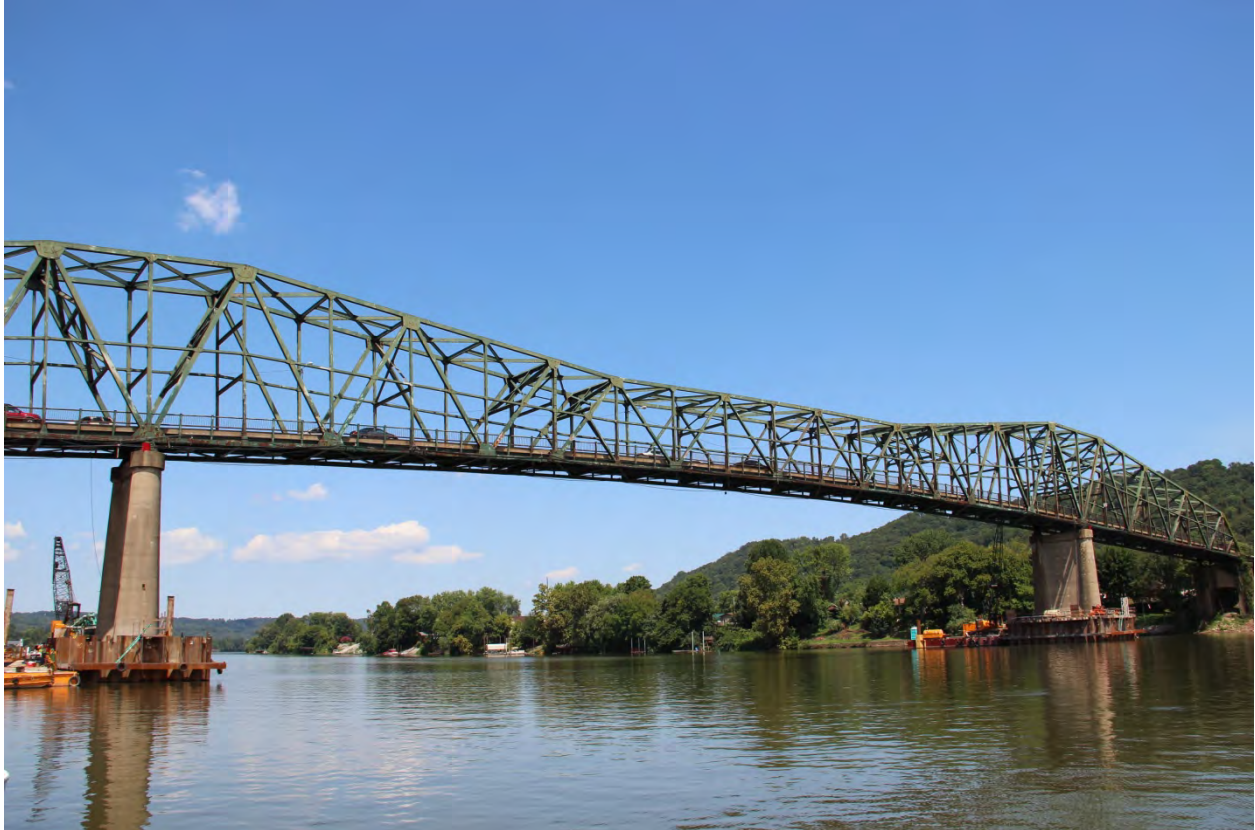
PHOTO 32 SOUTHEAST ELEVATION OF CANTILEVERED AND SUSPENDED TRUSS SPAN NO. 7 BETWEEN BRIDGE PIER NOS. 2 AND 3 SHOWING BOTTOM CHORD, VERTICAL AND DIAGONAL MEMBERS, SWAY FRAMES, TOP LATERAL BRACING, AND TOP CHORD, FACING NORTHWEST.
