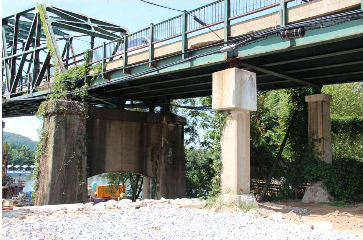
PHOTO 18 SOUTHEAST ELEVATION OF NORTHEAST VIADUCT SPAN NO. 9 SHOWING BRIDGE PIER NO. 4 AND VIADUCT PEDESTAL NO. 5, FACING SOUTHWEST.
