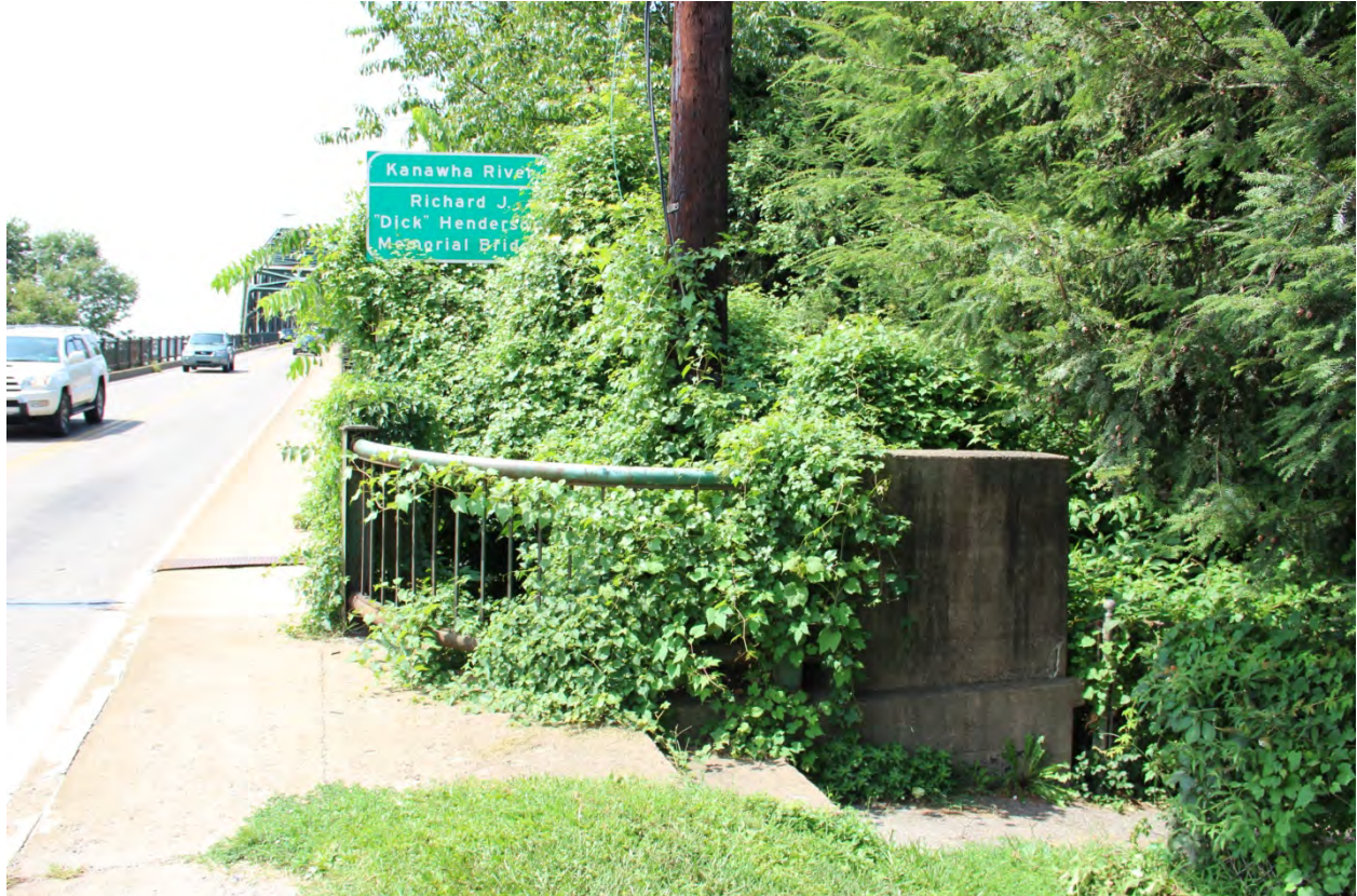
PHOTO 47 DETAIL OF SIDEWALK AND CURVED HANDRAILING AND CONCRETE END POST ASSEMBLY ALONG NORTHWEST ELEVATION OF NORTHEAST APPROACH, FACING SOUTHWEST.
