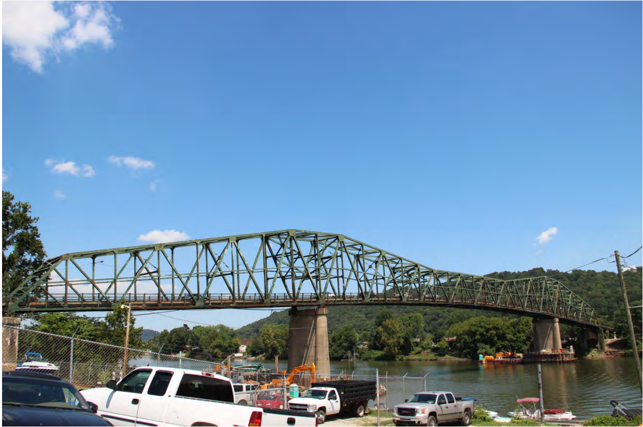
PHOTO 1 OVERVIEW SHOWING SOUTHEAST ELEVATION OF TRUSS SPANS (SPAN NOS. 6, 7, 8), FACING NORTHWEST.
