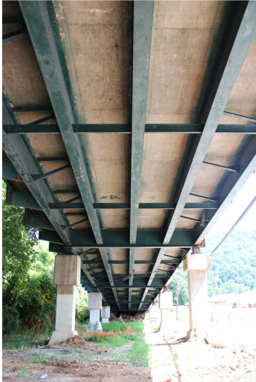
PHOTO 20 UNDERSIDE OF NORTHEAST VIADUCT SPAN NOS. 10 THROUGH 14 SHOWING VIADUCT PEDESTALS, ROCKER SHOES, FLOOR BEAMS, STRINGERS, AND INTERMEDIATE SIDEWALK AND RAIL POST BRACKETS, FACING NORTHEAST.
