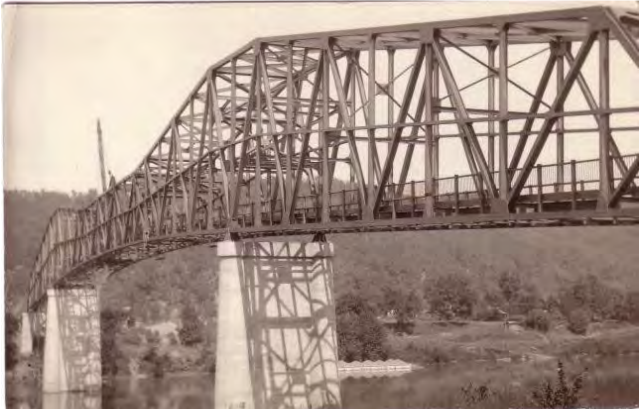
Figure 8: 1934 photograph of the St. Albans-Nitro Bridge under construction. Available from, Rich Hively, "St. Albans-Nitro Bridge," Nitro, West Virginia 25143, 2012.
