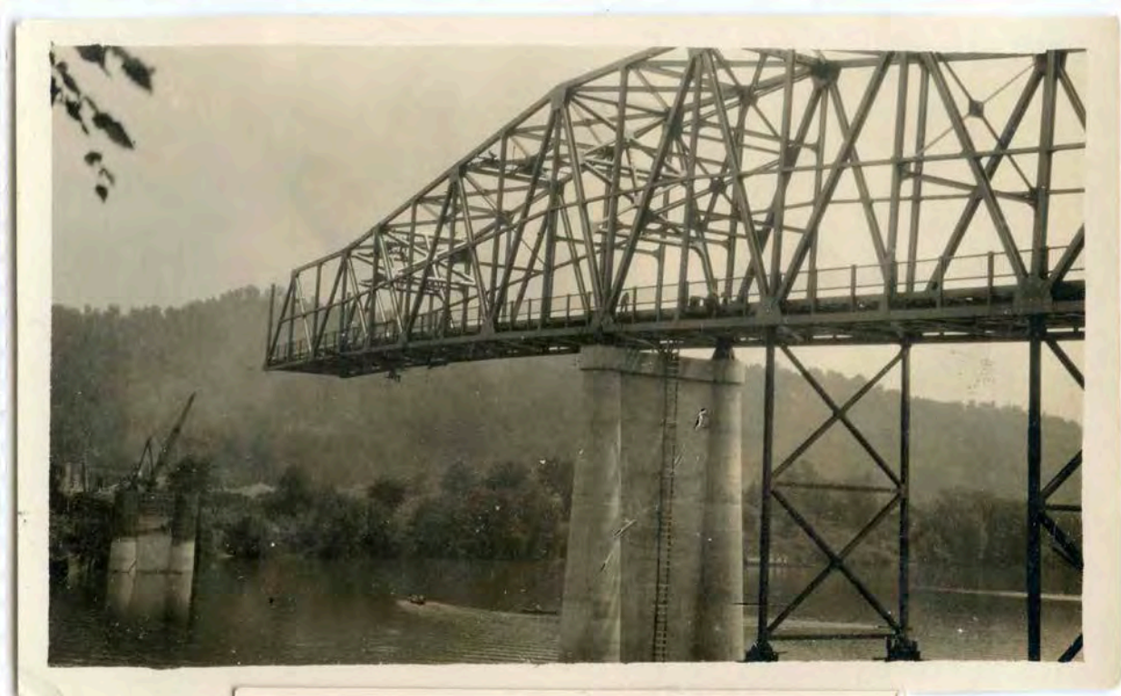
Figure 6: 1934 photograph of the St. Albans-Nitro Bridge under construction. Photograph available from St. Albans Historical Society.
