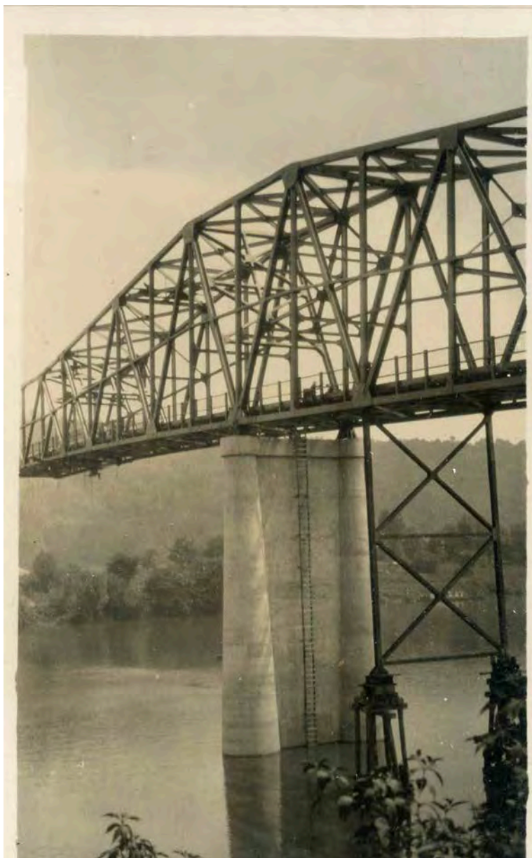
Figure 5: 1934 photograph of the St. Albans-Nitro Bridge under construction. Photograph available from St. Albans Historical Society.
