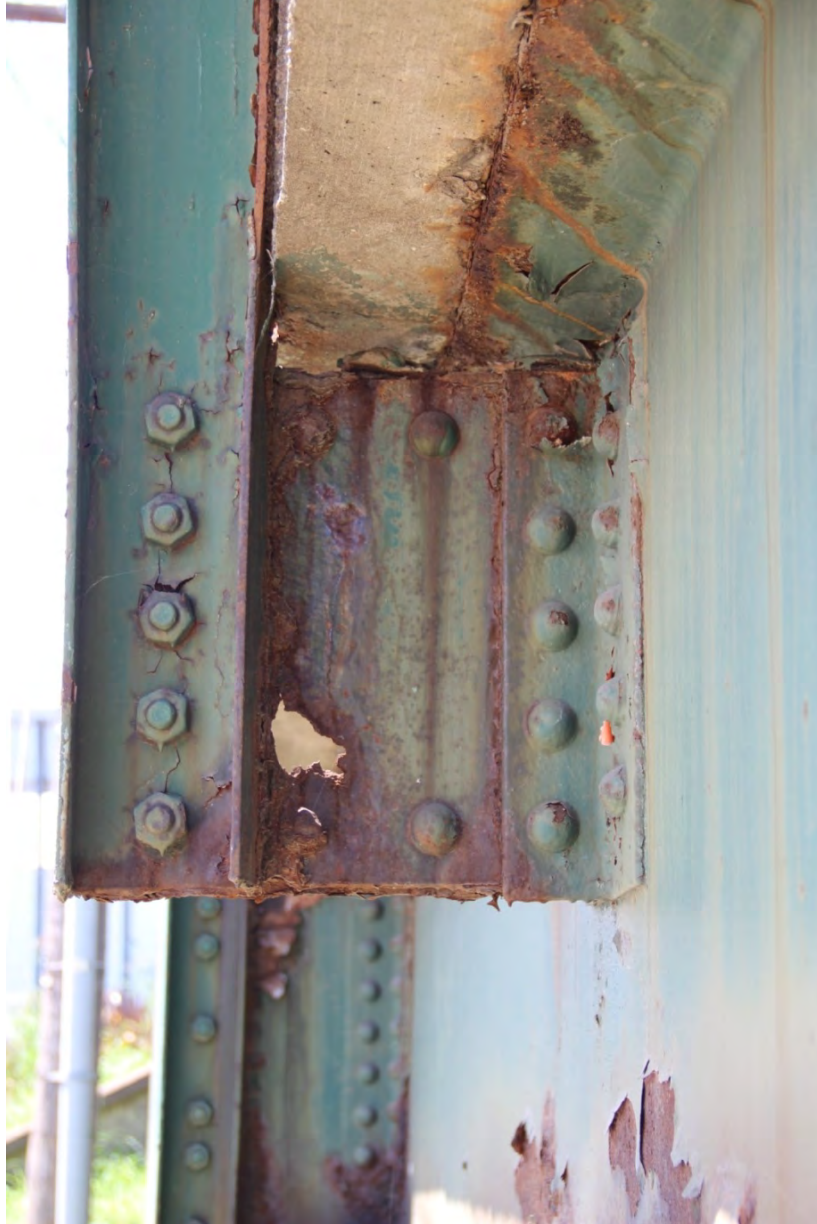
PHOTO 40 DETAIL OF AN INTERMEDIATE HANDRAIL SUPPORT BRACKET ALONG SOUTHEAST ELEVATION, FACING SOUTHWEST.
