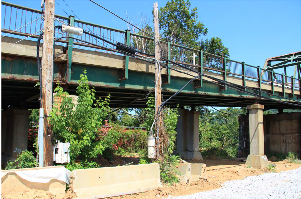
PHOTO 8 SOUTHEAST ELEVATION OF SOUTHWEST VIADUCT SPAN NO. 4 SHOWING VIADUCT PEDESTAL NOS. 3 AND 4, FACING NORTHWEST.
