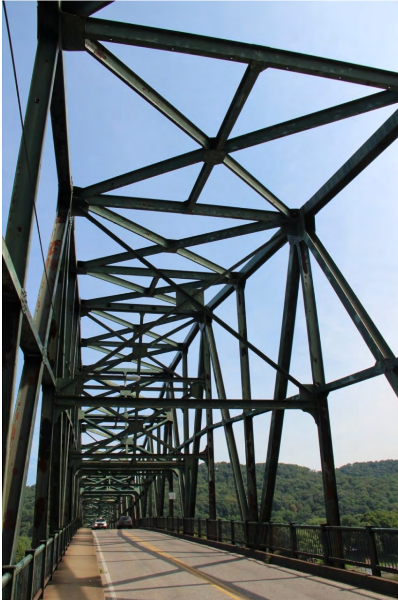
PHOTO 30 INTERIOR VIEW FROM DECK OF CANTILEVER TRUSS SPAN NOS. 6 AND 7 SHOWING BRIDGE DECK, VERTICAL AND DIAGONAL TRUSS MEMBERS, SWAY FRAMES, TOP CHORD, AND TOP LATERAL BRACING, FACING NORTHEAST.
