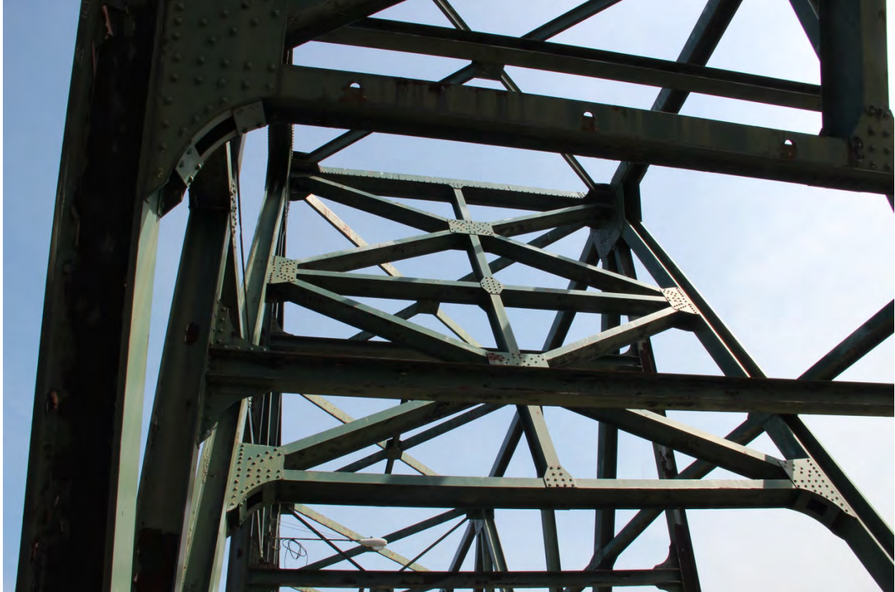
PHOTO 31 INTERIOR VIEW OF JUNCTION OF CANTILEVER TRUSS SPAN NOS. 6 AND 7 ABOVE BRIDGE PIER NO. 2 SHOWING VERTICAL, HORIZONTAL, AND DIAGONAL TRUSS MEMBERS, SWAY FRAMES, TOP CHORD, AND TOP LATERAL BRACING, FACING NORTHEAST.
