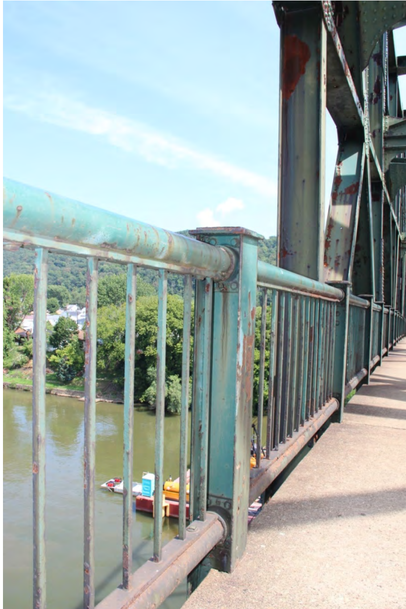
PHOTO 41 DETAIL OF SIDEWALK HANDRAILING AND POST ASSEMBLY ALONG NORTHWEST ELEVATION, FACING NORTH.
