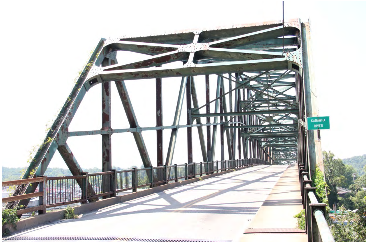
PHOTO 38 NORTHEAST PORTAL OF CANTILEVER TRUSS SPAN NO. 8 SHOWING BRIDGE DECK, EXPANSION JOINT, PORTAL BRACING, RIVETED CONNECTIONS, VERTICAL AND DIAGONAL TRUSS MEMBERS, AND SWAY FRAMES, FACING SOUTH.
