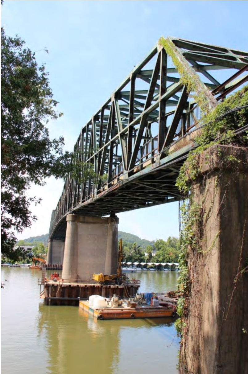
PHOTO 37 SOUTHEAST ELEVATION AND UNDERSIDE OF CANTILEVERED TRUSS SPAN NO. 8 BETWEEN BRIDGE PIER NOS. 3 AND 4 SHOWING FLOOR SYSTEM, BOTTOM CHORD, VERTICAL AND DIAGONAL MEMBERS, SWAY FRAMES, TOP CHORD, AND TOP LATERAL BRACING, FACING SOUTHWEST.
