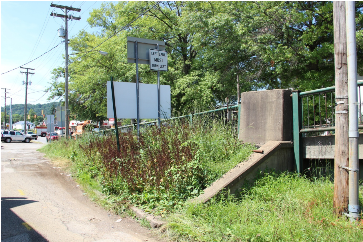
PHOTO 4 SOUTHEAST ELEVATION OF EARTHEN FILLED SOUTHWEST APPROACH AND SOUTHWEST ABUTMENT AND WINGWALL, FACING SOUTHWEST.
