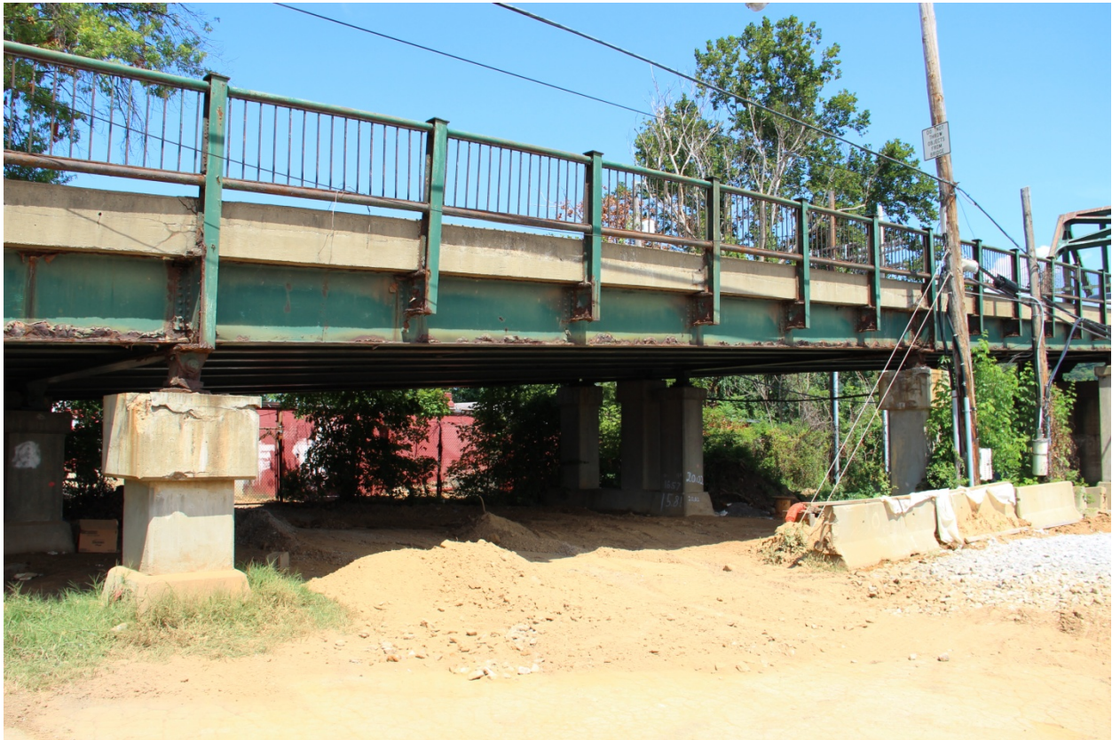
PHOTO 7 SOUTHEAST ELEVATION OF SOUTHWEST VIADUCT SPAN NO. 3 SHOWING VIADUCT PEDESTAL NOS. 2 AND 3, FACING NORTHWEST.
