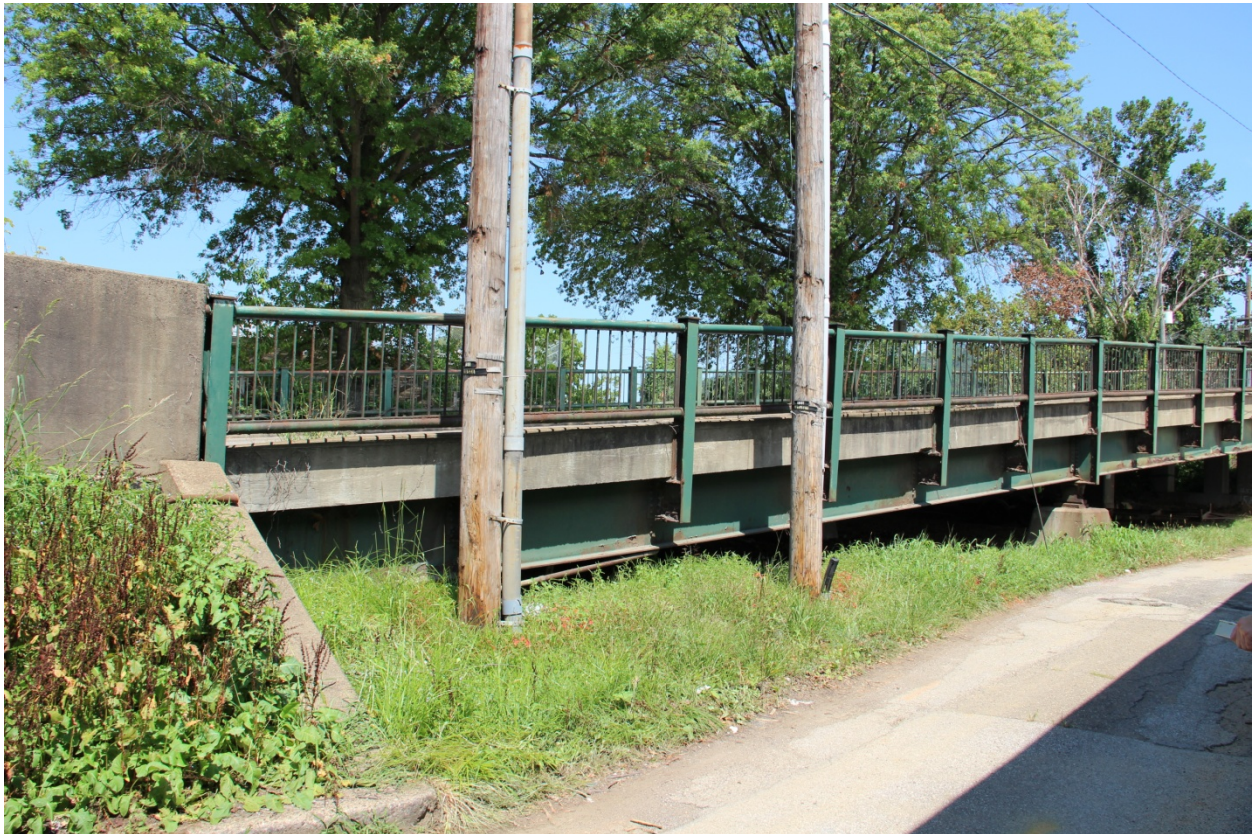
PHOTO 5 SOUTHEAST ELEVATION OF SOUTHWEST VIADUCT SPAN NO. 1 SHOWING SOUTHWEST ABUTMENT AND WINGWALL AND VIADUCT PEDESTAL NO.1, FACING NORTH.
