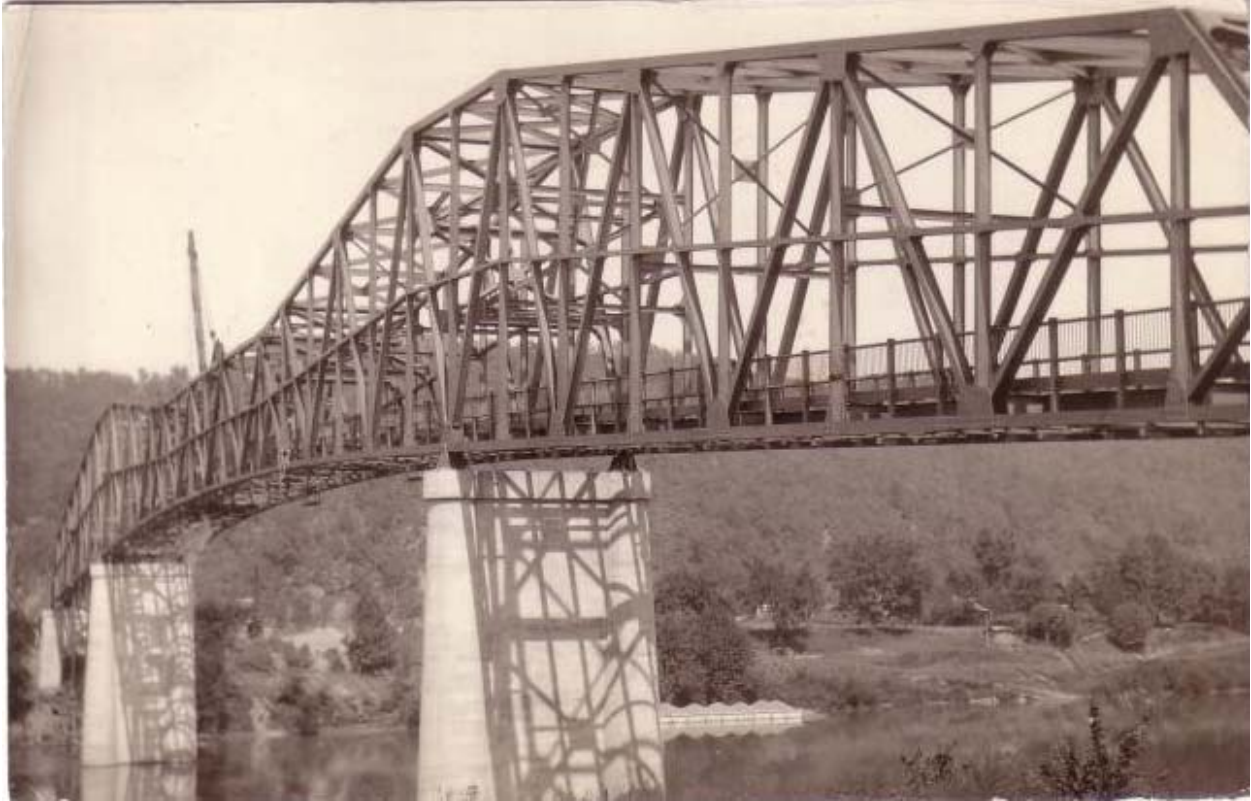
FIGURE 6: 1934 photograph of the St. Albans-Nitro Bridge under construction. Available from, Rich Hively, "St. Albans-Nitro Bridge," Nitro, West Virginia 25143, 2012.
