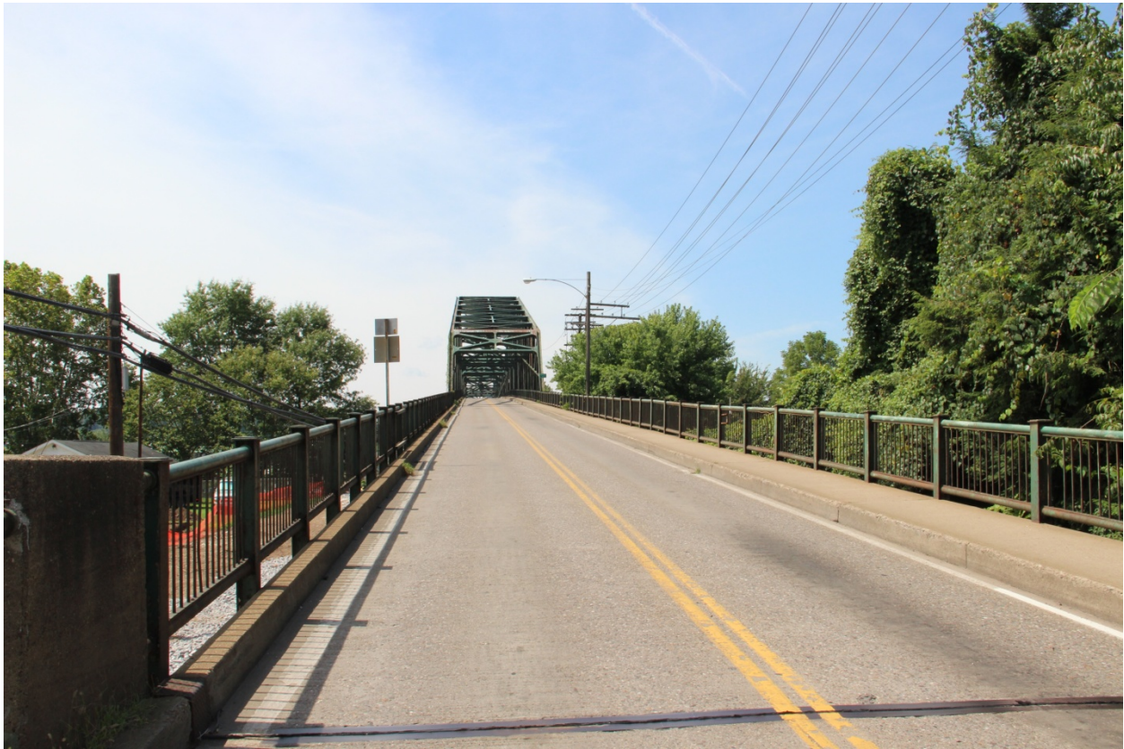
PHOTO 3 OVERVIEW SHOWING NORTHEAST VIADUCT SPANS (SPAN NOS. 9 THROUGH 14) AND PORTAL OF TRUSS SPAN (SPAN NO. 8), FACING SOUTHWEST.
