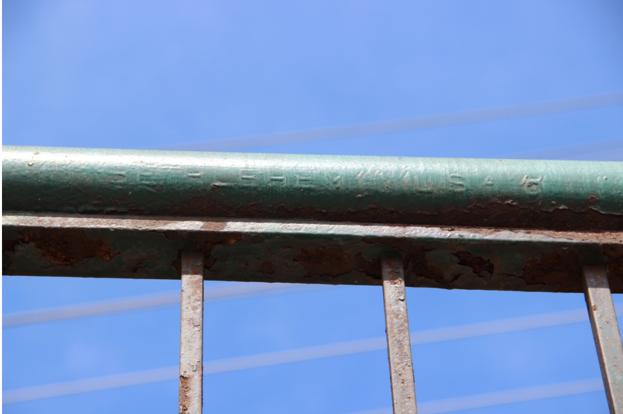
PHOTO 43 DETAIL OF HANDRAILING SHOWING EMBOSSED MANUFACTURER'S MARK "BETHLEHEM USA" ALONG SOUTHEAST ELEVATION, FACING NORTHWEST.
