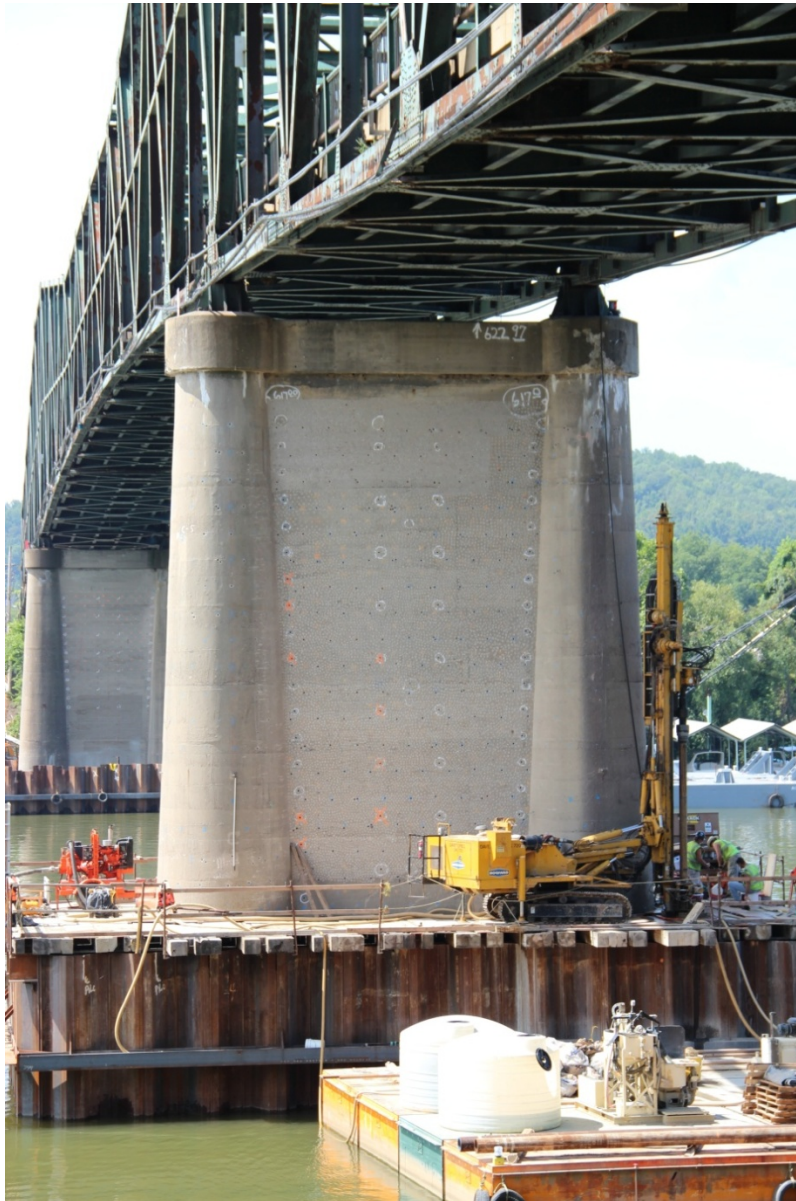
PHOTO 14 NORTHEAST ELEVATION OF BRIDGE PIER NO. 3 SHOWING BRIDGE SHOE AND UNDERSIDE OF CANTILEVER TRUSS SPAN NOS. 7 AND 8, FACING SOUTHWEST.
