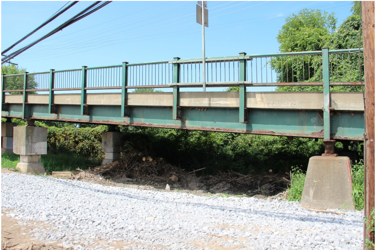
PHOTO 23 SOUTHEAST ELEVATION OF NORTHEAST VIADUCT SPAN NO. 13 SHOWING VIADUCT PEDESTAL NOS. 8 AND 9, FACING SOUTHWEST.
