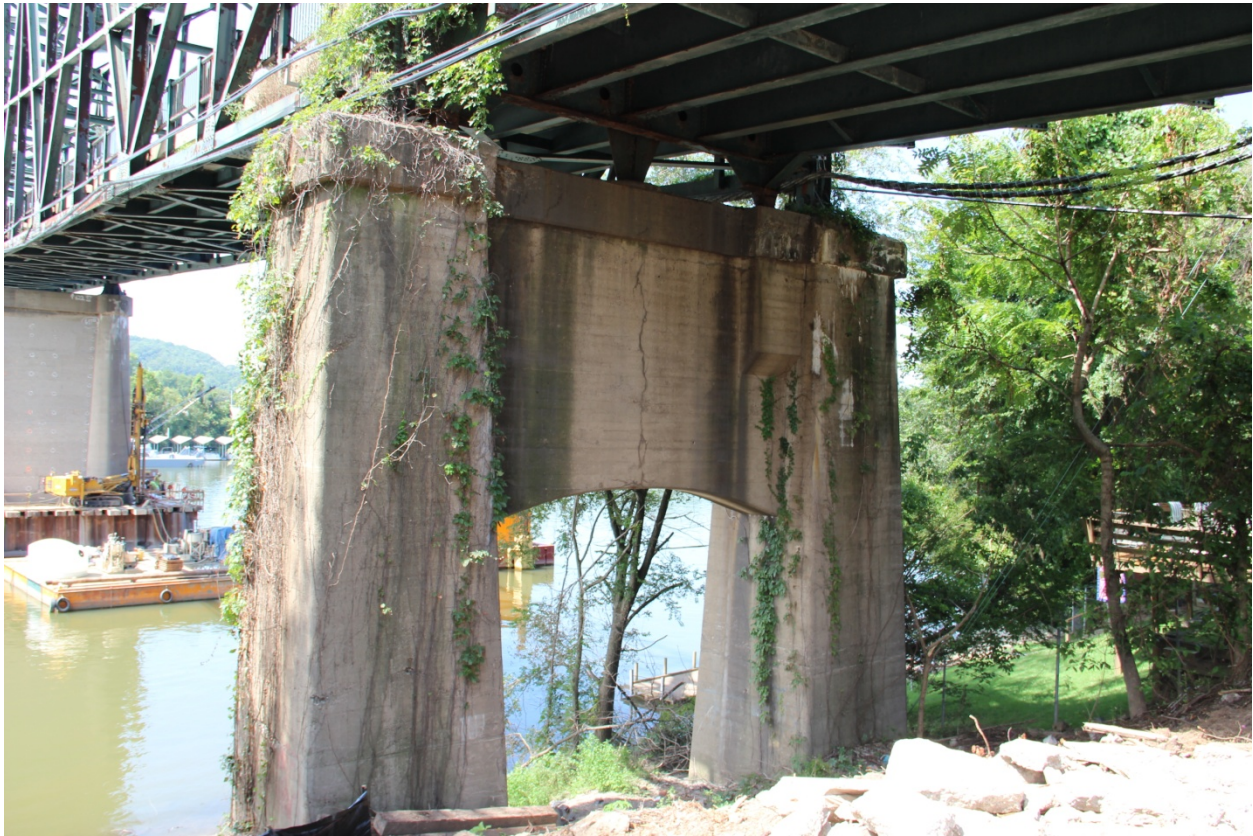
PHOTO 16 SOUTHEAST AND NORTHEAST ELEVATIONS OF BRIDGE PIER NO. 4, FACING SOUTHWEST.
