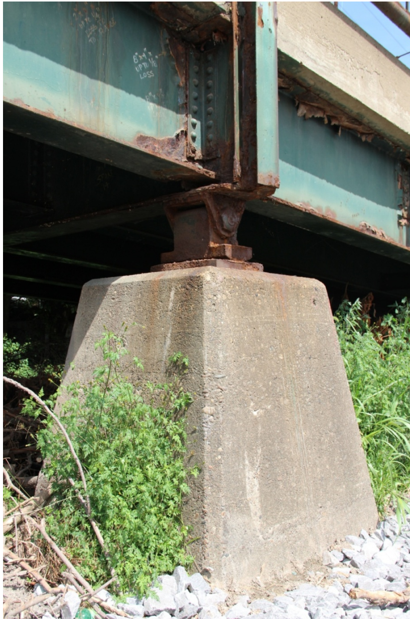
PHOTO 24 DETAIL OF VIADUCT PEDESTAL NO.9 AND ROCKER SHOE ALONG NORTHEAST ELEVATION, FACING NORTH.
