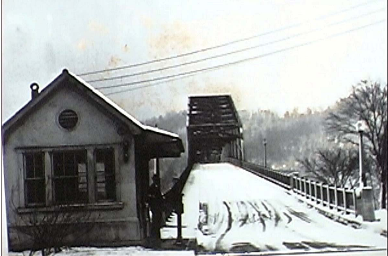
FIGURE 10: Ca. 1939 historic postcard depicting the St. Albans-Nitro Bridge, looking north toward the St. Albans approach and toward the toll house. Available from St. Albans Historical Society.
