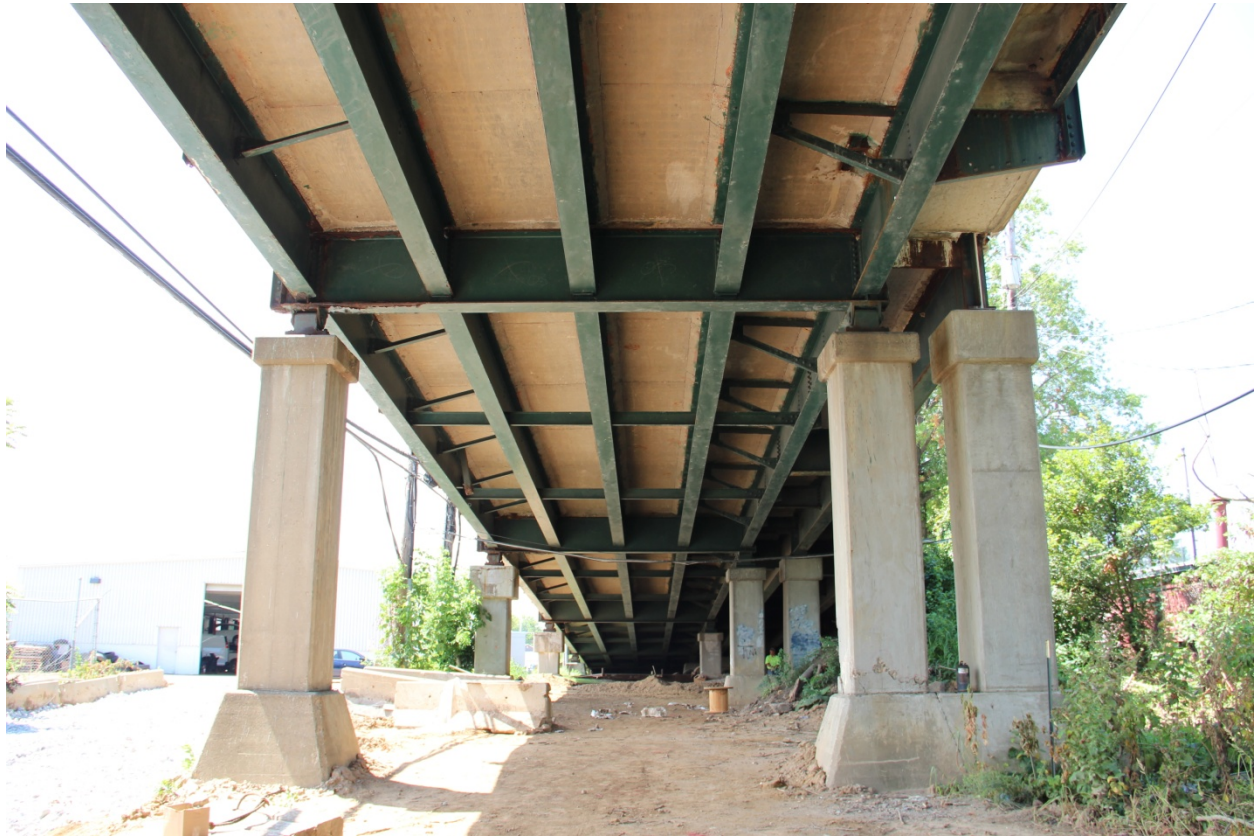
PHOTO 10 UNDERSIDE OF SOUTHWEST VIADUCT SPAN NOS. 5 THROUGH 1 SHOWING VIADUCT PEDESTALS, ROCKER SHOES, FLOOR BEAMS, STRINGERS, AND INTERMEDIATE SIDEWALK AND RAIL POST BRACKETS, FACING SOUTHWEST (NOTE NORTHWESTERN-MOST (RIGHT) PEDESTALS WERE ADDED FOR A TURN LANE IN 1977).
