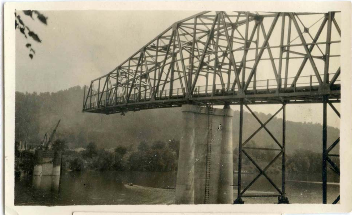
FIGURE 4: 1934 photograph of the St. Albans-Nitro Bridge under construction. Photograph available from St. Albans Historical Society.
