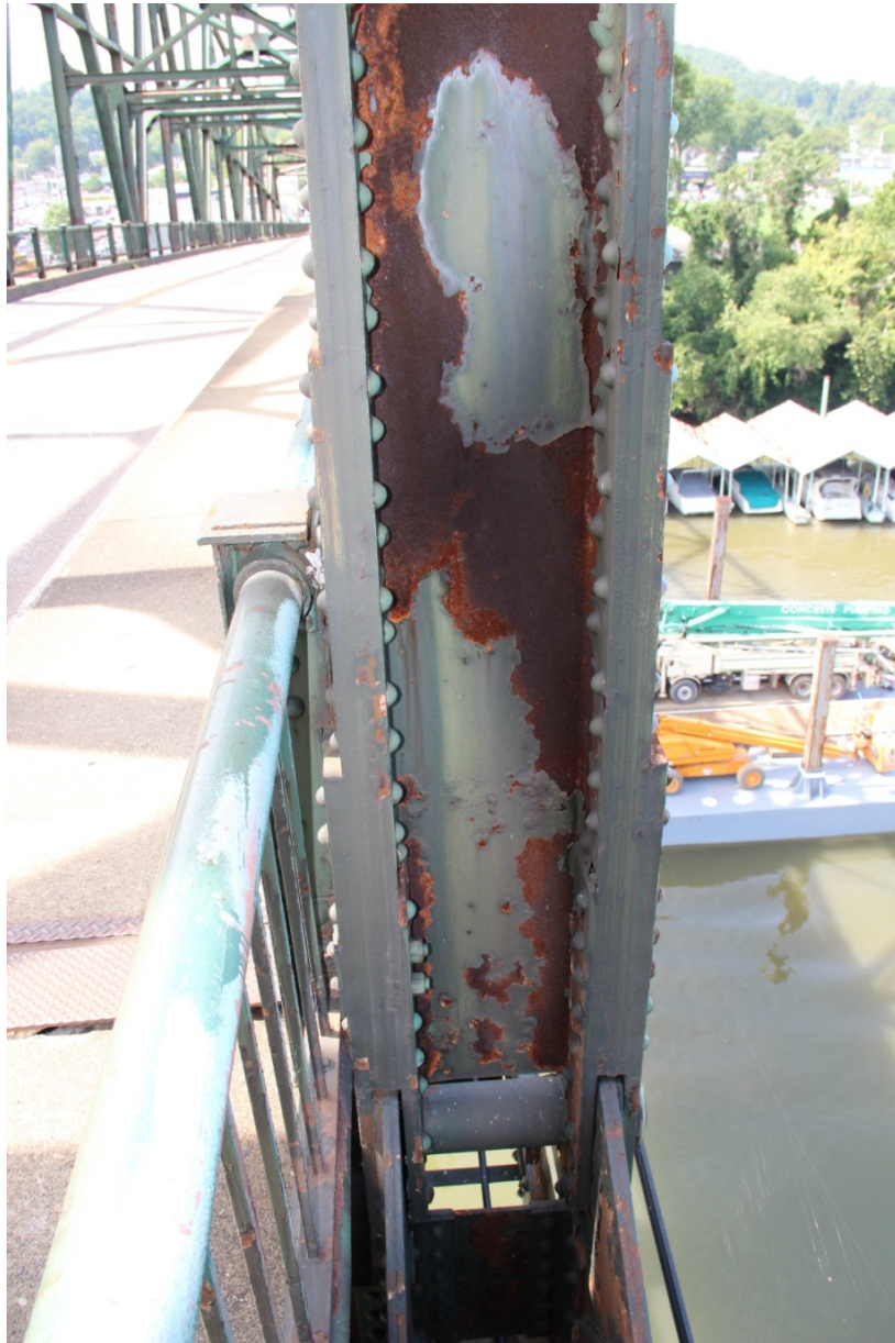
PHOTO 35 DETAIL OF BUILT-UP, RIVETED VERTICAL MEMBER OF TRUSS SPAN NO.7 AT JUNCTION OF CANTILEVERED AND SUSPENDED PORTION OF SPAN, FACING SOUTHWEST.
