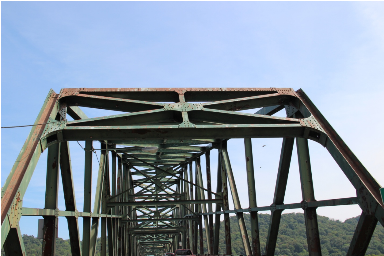
PHOTO 28 SOUTHWEST PORTAL OF CANTILEVER TRUSS SPAN NO. 6 SHOWING PORTAL BRACING, RIVETED CONNECTIONS, VERTICAL AND DIAGONAL TRUSS MEMBERS, SWAY FRAMES, TOP CHORD, AND TOP LATERAL BRACING, FACING NORTHEAST.
