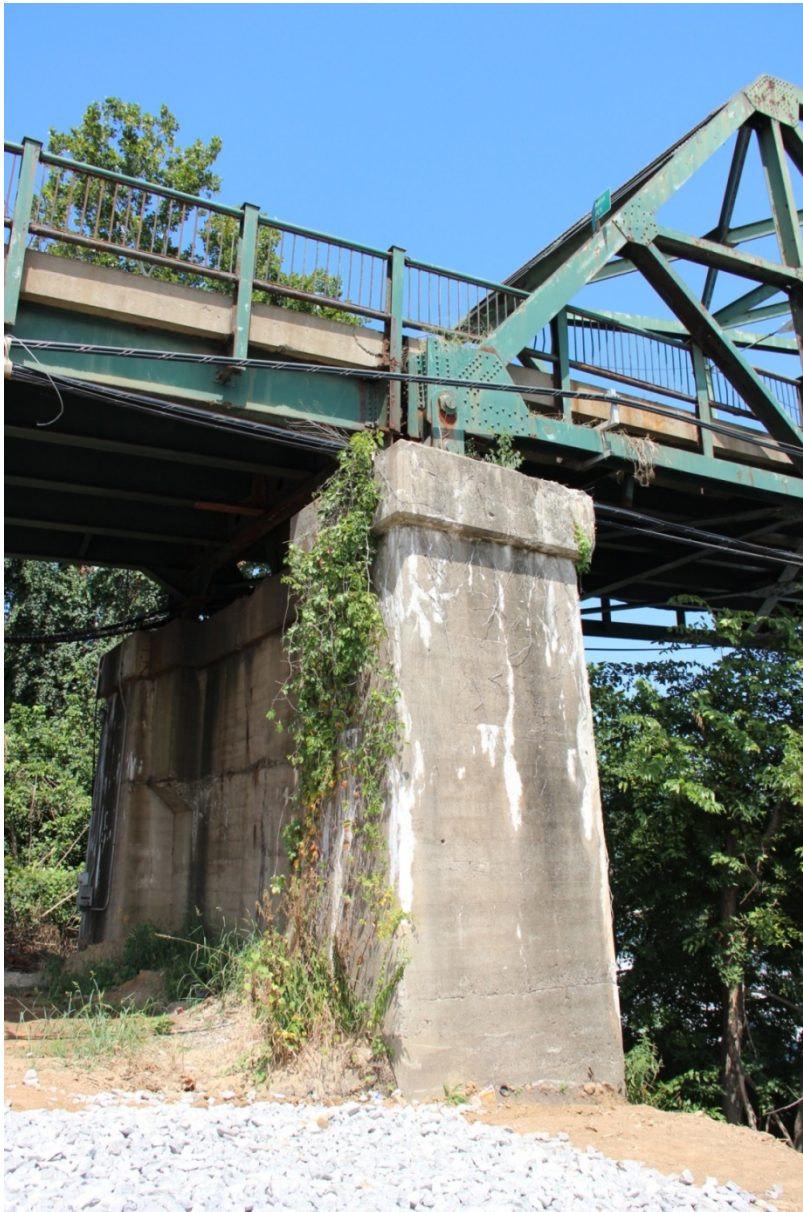
PHOTO 12 SOUTHWEST AND SOUTHEAST ELEVATION OF BRIDGE PIER NO. 1 SHOWING BRIDGE SHOE AND ANCHORAGE ASSEMBLY OF CANTILEVER TRUSS SPAN NO. 6, FACING NORTHWEST.
