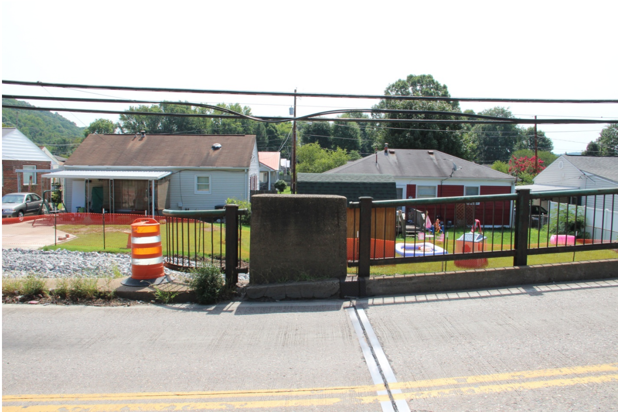
PHOTO 46 DETAIL OF HANDRAILING, POSTS, AND CONCRETE END POST ASSEMBLY ALONG SOUTHEAST ELEVATION OF NORTHWEST APPROACH, FACING SOUTHEAST.
