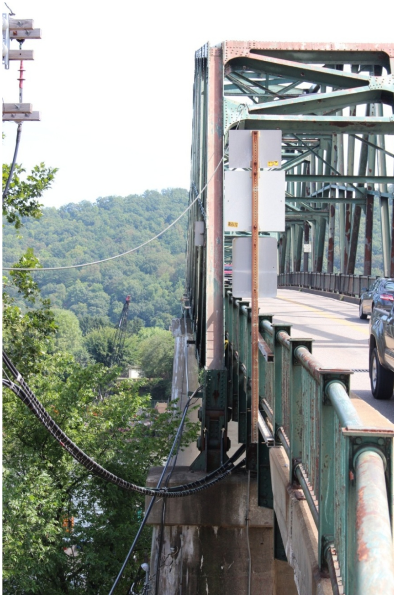
PHOTO 27 NORTHWEST ELEVATION OF BRIDGE SHOWING BRIDGE SHOE AND ANCHORAGE ASSEMBLY OF CANTILEVER TRUSS SPAN NO. 6 ATOP BRIDGE PIER NO. 1, FACING NORTHEAST.
