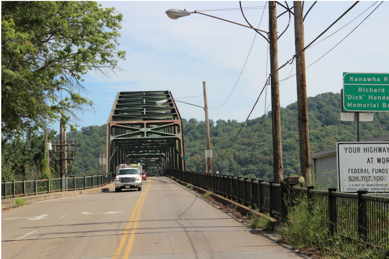
PHOTO 2 OVERVIEW SHOWING SOUTHWEST VIADUCT SPANS (SPAN NOS. 1 THROUGH 5) AND PORTAL OF TRUSS SPAN (SPAN NO. 6), FACING NORTHEAST.
