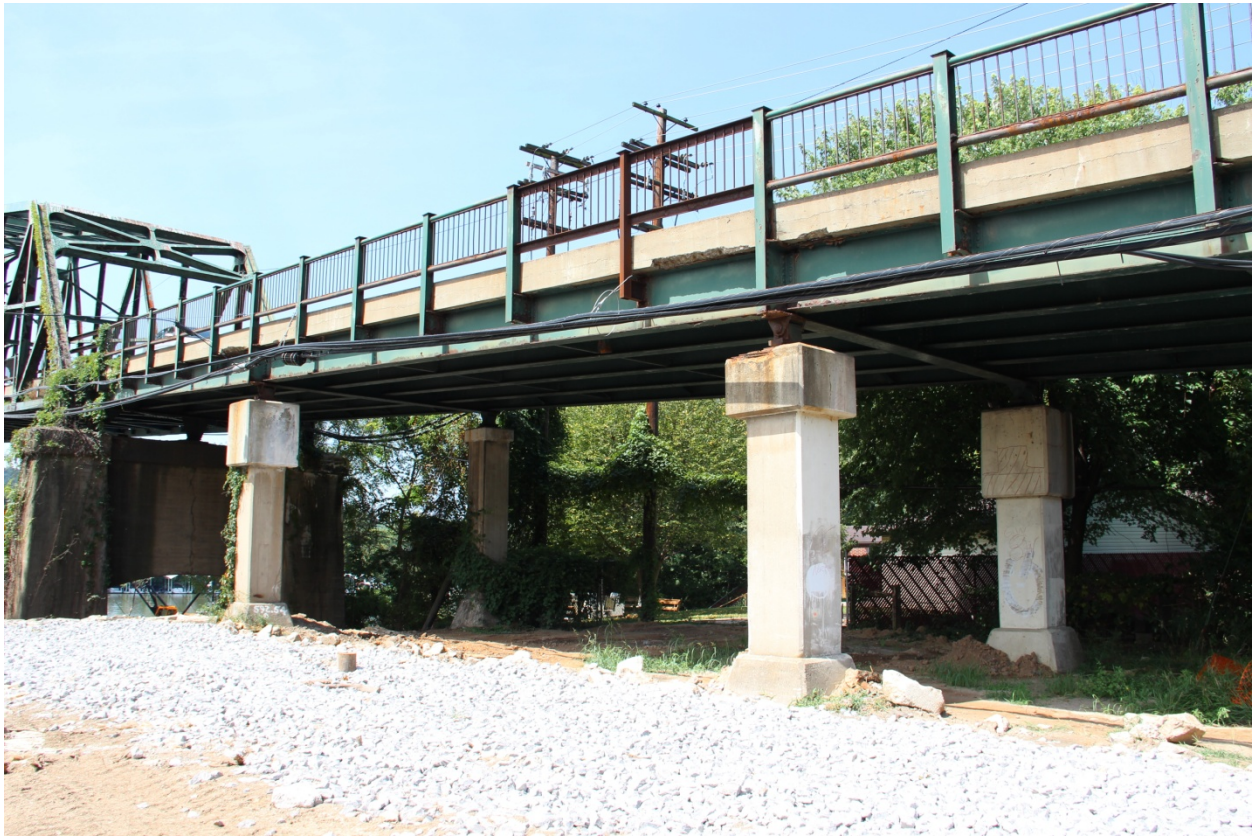
PHOTO 19 SOUTHEAST ELEVATION OF NORTHEAST VIADUCT SPAN NO. 10 SHOWING VIADUCT PEDESTAL NOS. 5 AND 6, FACING SOUTHWEST.
