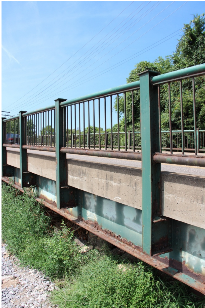
PHOTO 42 DETAIL OF HANDRAIL, POSTS, INTERMEDIATE HANDRAIL SUPPORTS, AND CONNECTING BRACKETS ALONG SOUTHEAST ELEVATION OF SPAN 14, FACING SOUTHWEST.
