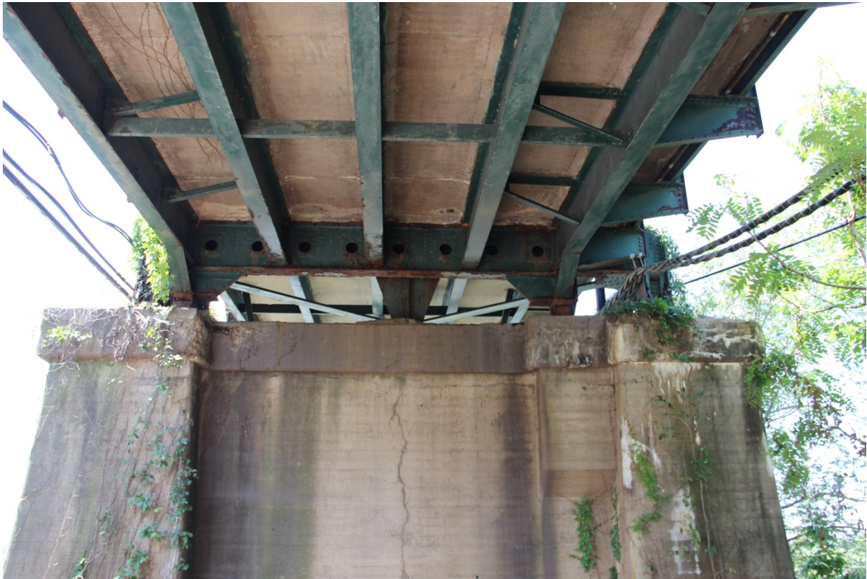
PHOTO 17 NORTHEAST ELEVATION OF BRIDGE PIER NO. 4 SHOWING FLOORBEAMS, STRINGERS, AND ROCKER SHOES OF NORTHEAST VIADUCT SPAN NO. 9 AND SHOES AND ANCHORAGE OF CANTILEVER TRUSS SPAN NO. 8, FACING SOUTHWEST.
