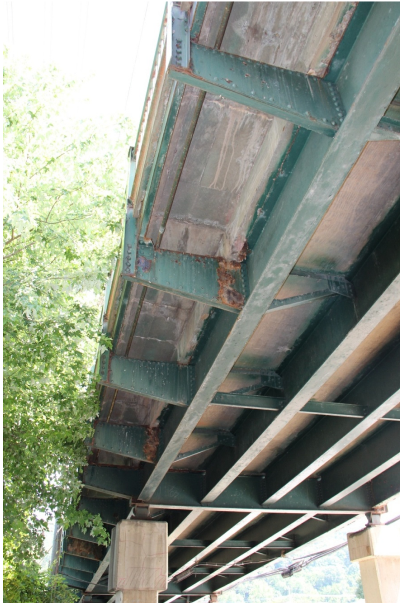
PHOTO 39 UNDERSIDE OF NORTHWEST APPROACH SPAN NO. 10 SHOWING INTERMEDIATE SIDEWALK AND HANDRAIL SUPPORT BRACKETS ALONG NORTHWEST ELEVATION, FACING NORTHEAST.
