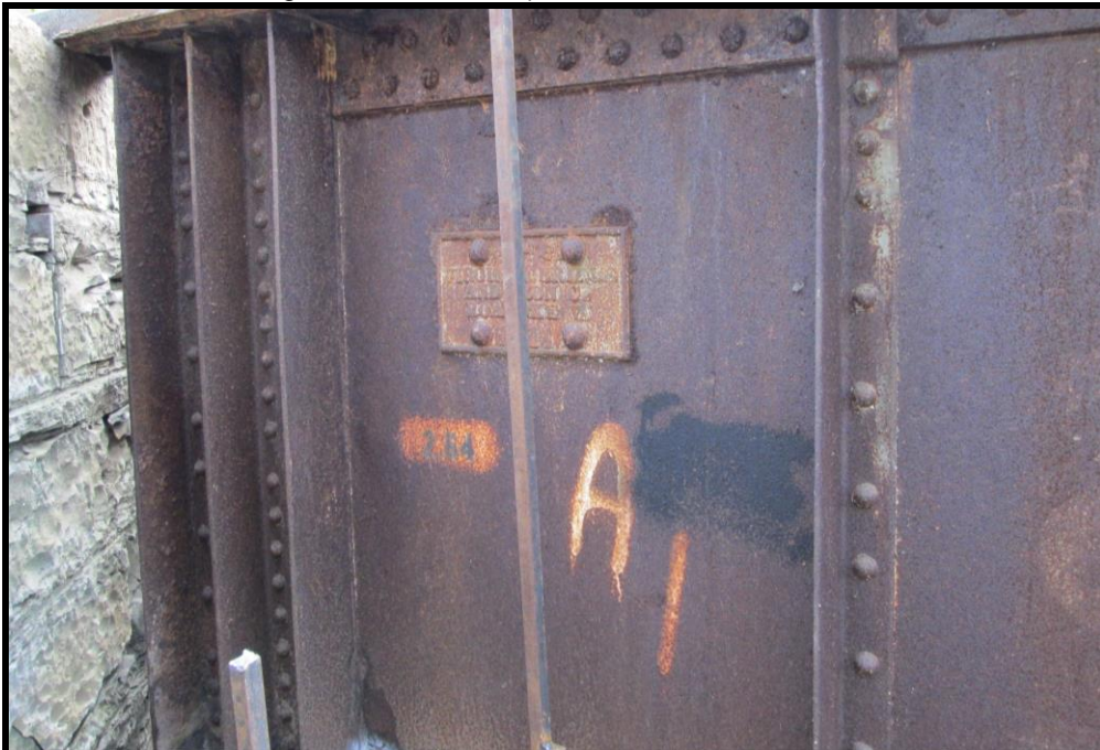
Plaque (same as in top photo) at North End West Girder of Bridge. Photo courtesy of WVDOH District 2 Engineers, Nov. 2013).
