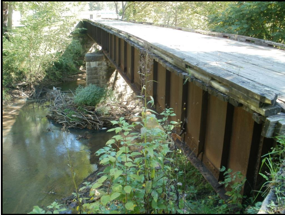
West (Upstream) Side of Fleming Deck Girder Bridge. View East/Northeast (WVDOH 2013)
