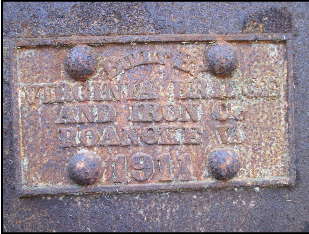
Plaque on West (Upstream) Side Girder on Fleming Bridge, as north end. Reads "BUILT BY / VIRGINIA BRIDGE / AND IRON CO. / ROANOKE VA / 1911. Photo courtesy of WVDOH District 2 Engineers, Nov. 2013)
