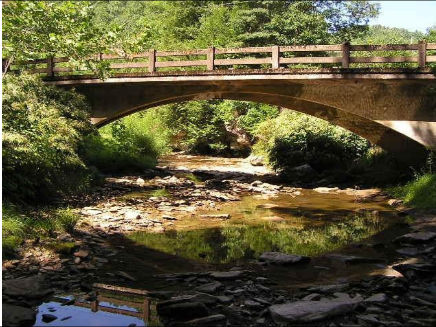
1. East Elevation Looking Upstream, View West
