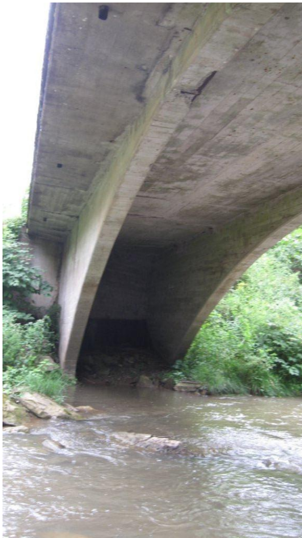
9. North End of Bridge, Exhibiting West Side Deck Overhang and Terminus of Arched Spandrels at North Abutment, View Northeast
