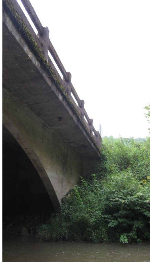
10. North End of Bridge, Exhibiting East Side Deck Overhang, Railing and Terminus of Arched Spandrel at North Abutment, View North/NW
