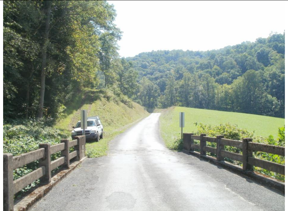
6. South Portion of Bridge Deck, View Southwest Along County Route 12
