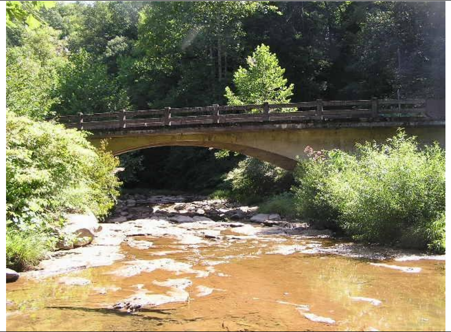
2. West Elevation Looking Downstream, View East
