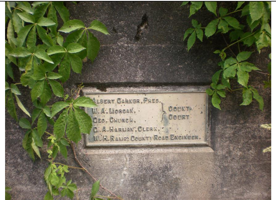
8. Bridge Plate on South End of East Railing, View Southeast
