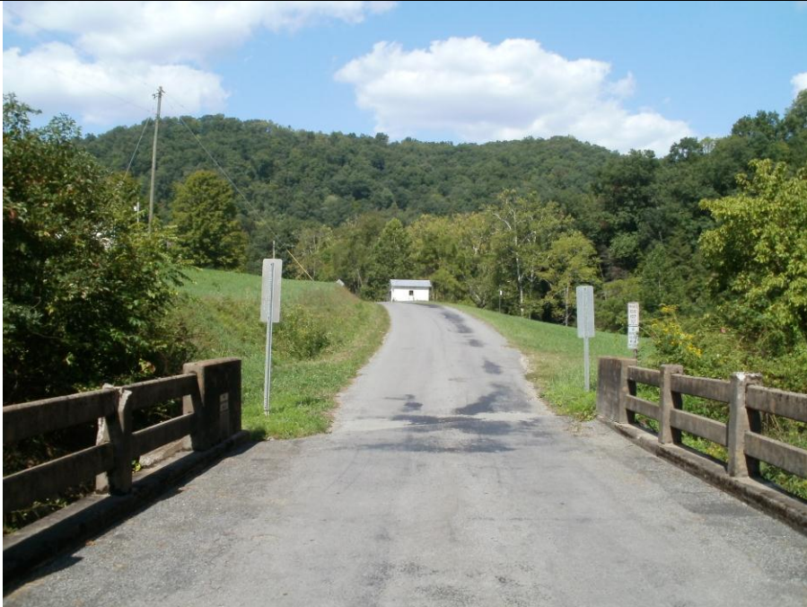
5. North Portion of Bridge Deck, View Northeast Along County Route 12
