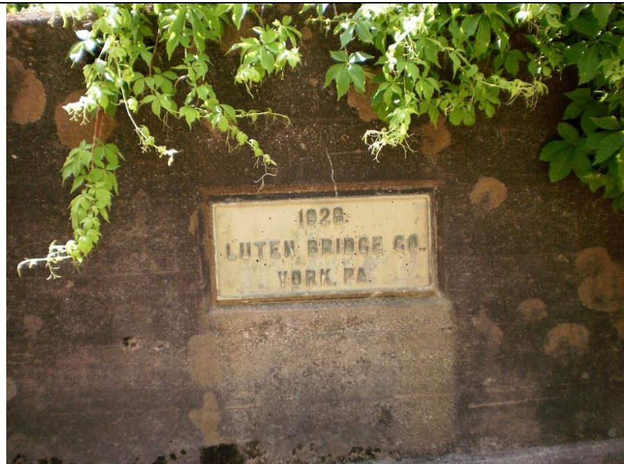
7. Bridge Plate on North End of West Railing, View Northwest
