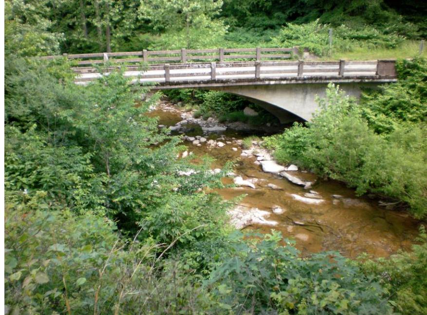
3. Overview, West Side of Bridge in Forefront, View Southeast
