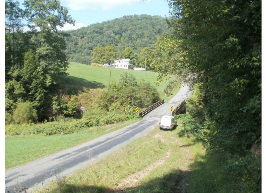
4. Overview of County Route 12 Looking Toward Bridge and Nearby Residence, View North/Northwest
