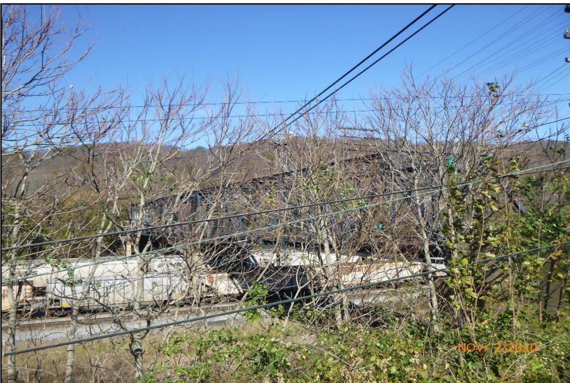
West elevation, obscured by vegetation. (Photo: WVDOH November 2020).
