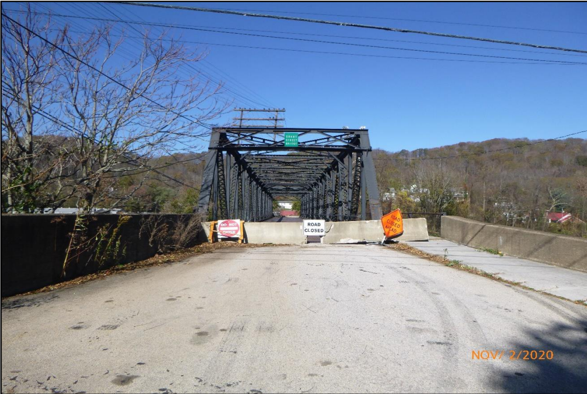
South approach. (Photo: WVDOH November 2020).
