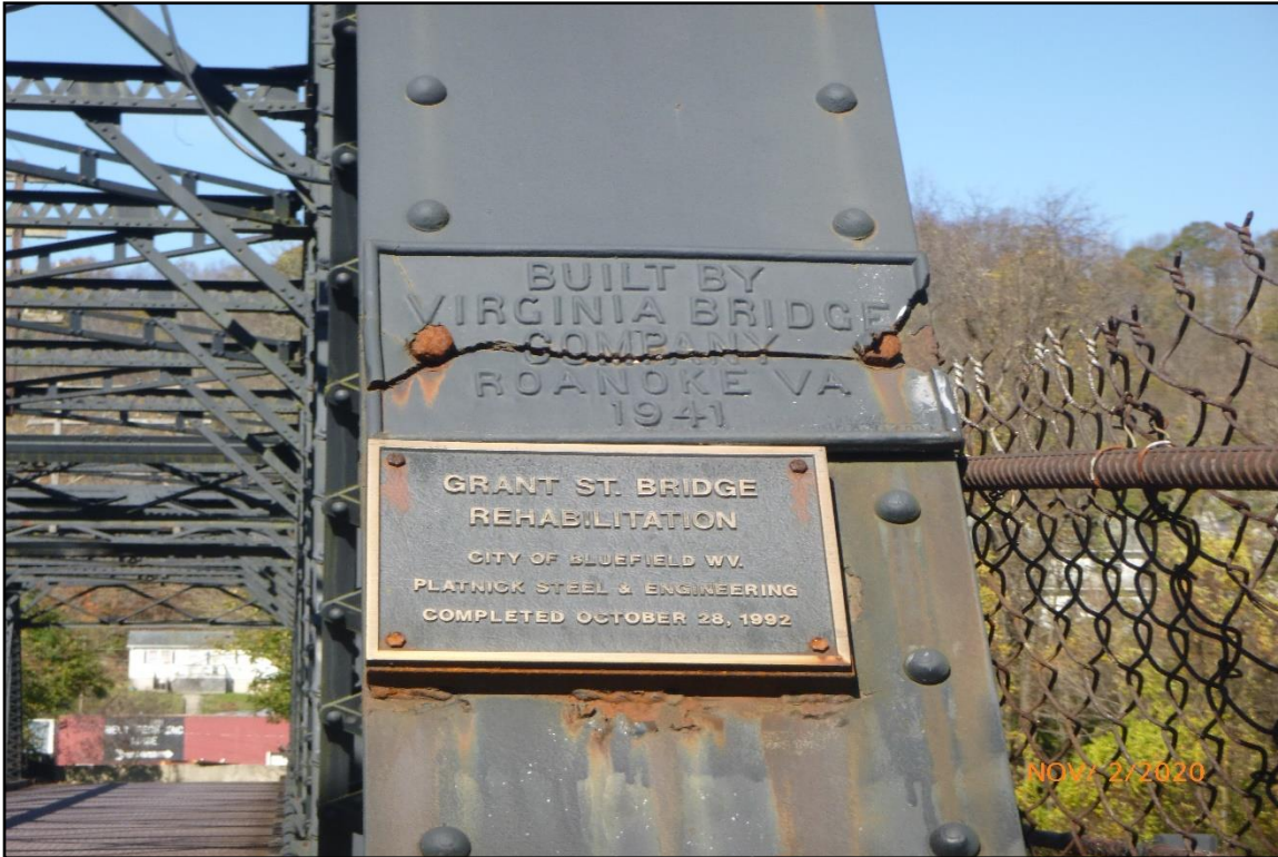
Detail of bridge plaques. (Photo: WVDOH November 2020).
