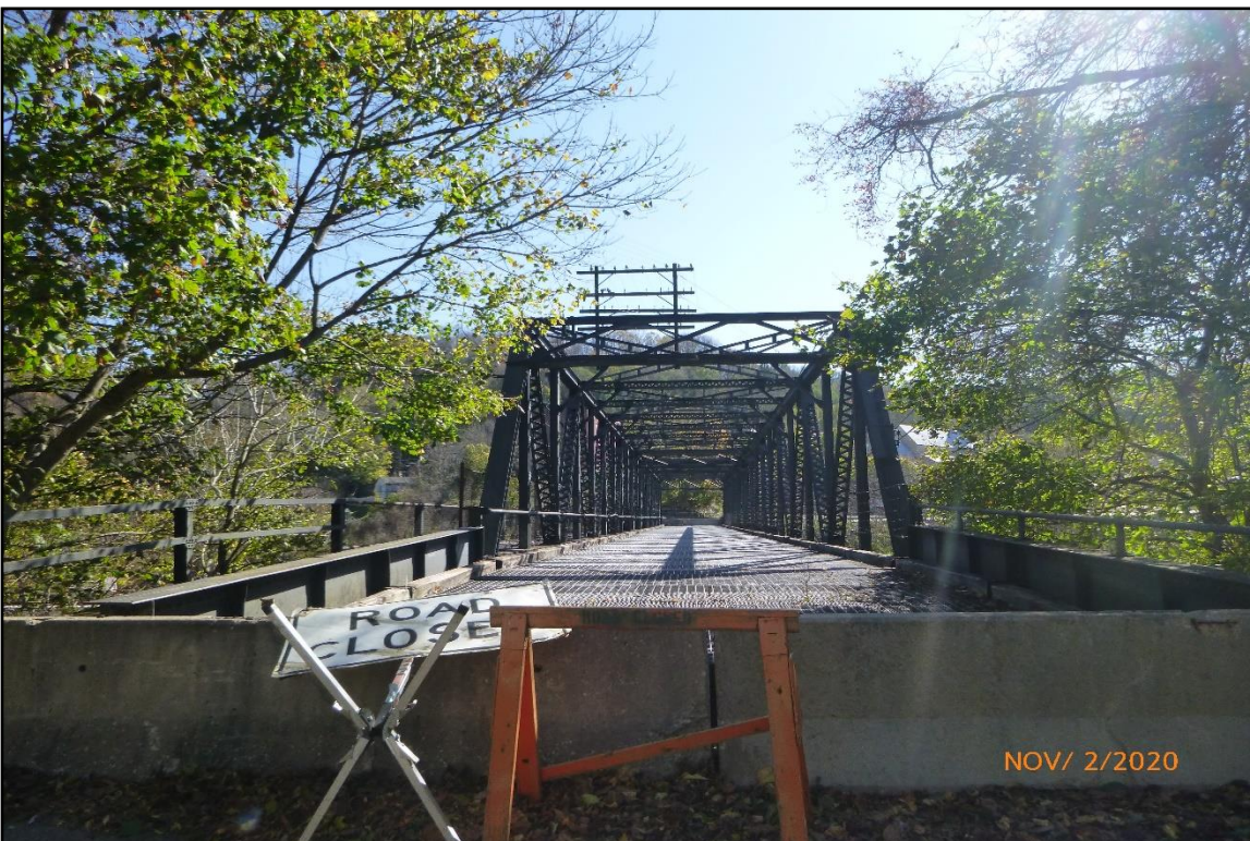
North approach. (Photo: WVDOH November 2020).
