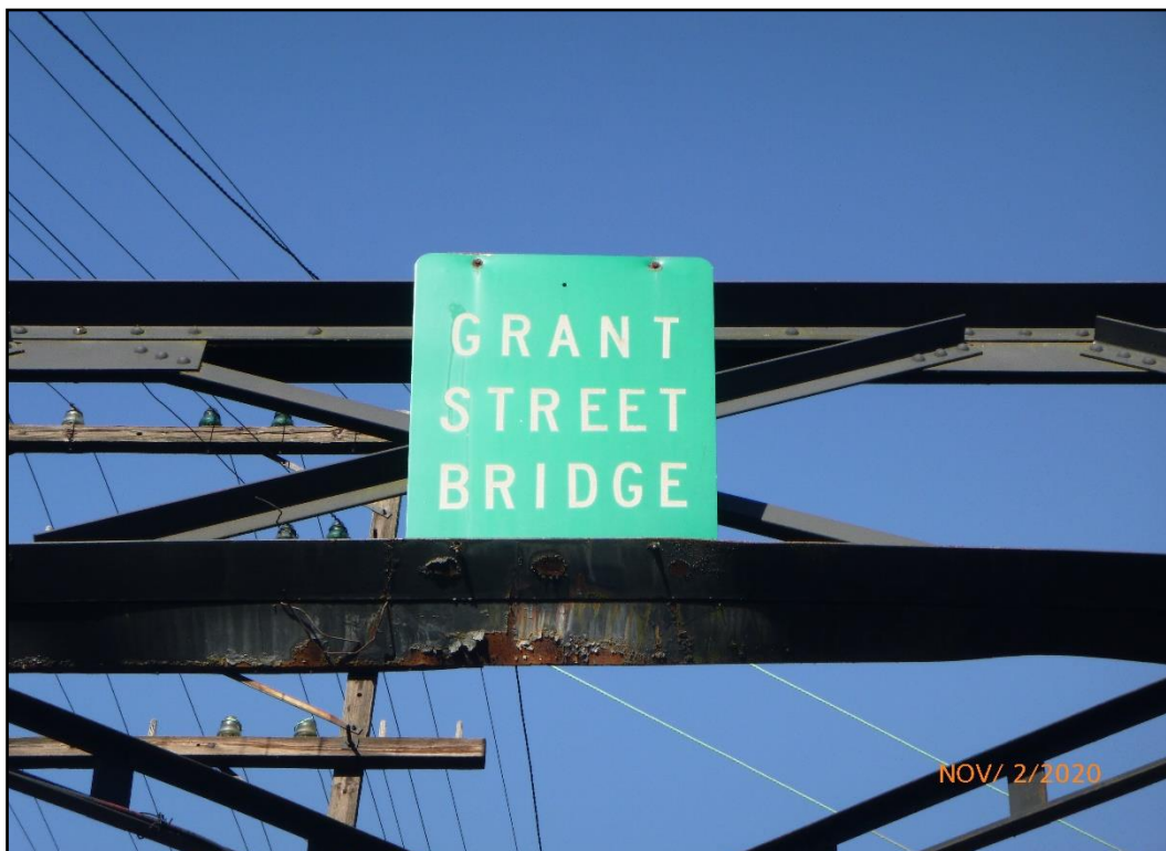
6. Bridge sign and upper laterals. Photo: WVDOH November 2020.
