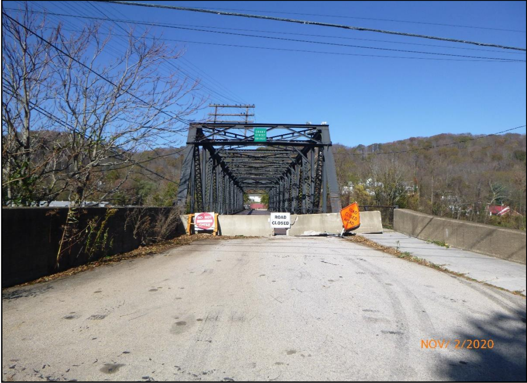
1. South approach. Photo: WVDOH November 2020.
