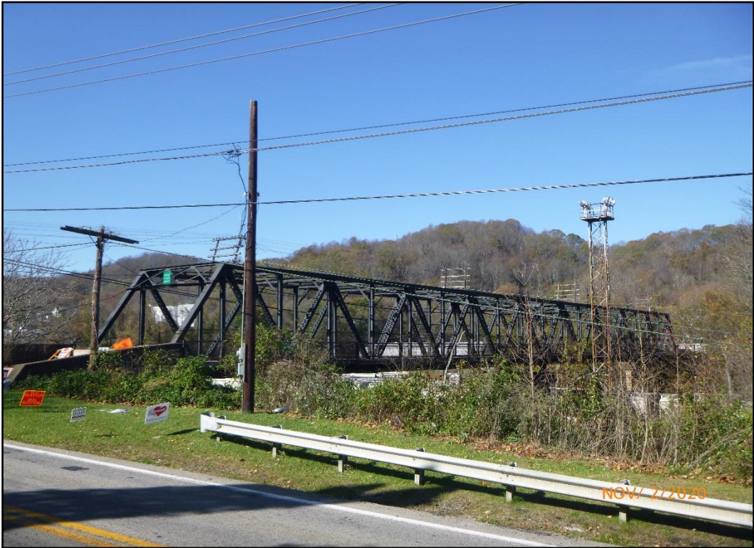
4. East elevation. Photo: WVDOH November 2020.
