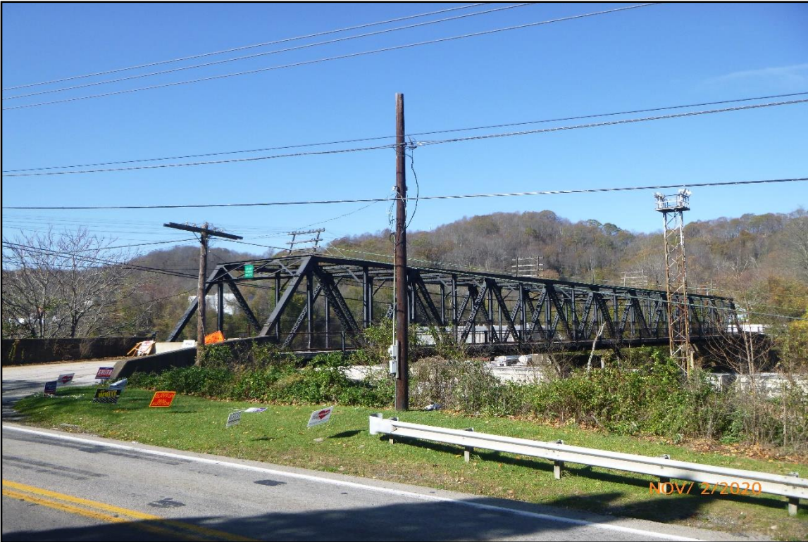
East elevation. (Photo: WVDOH November 2020).
