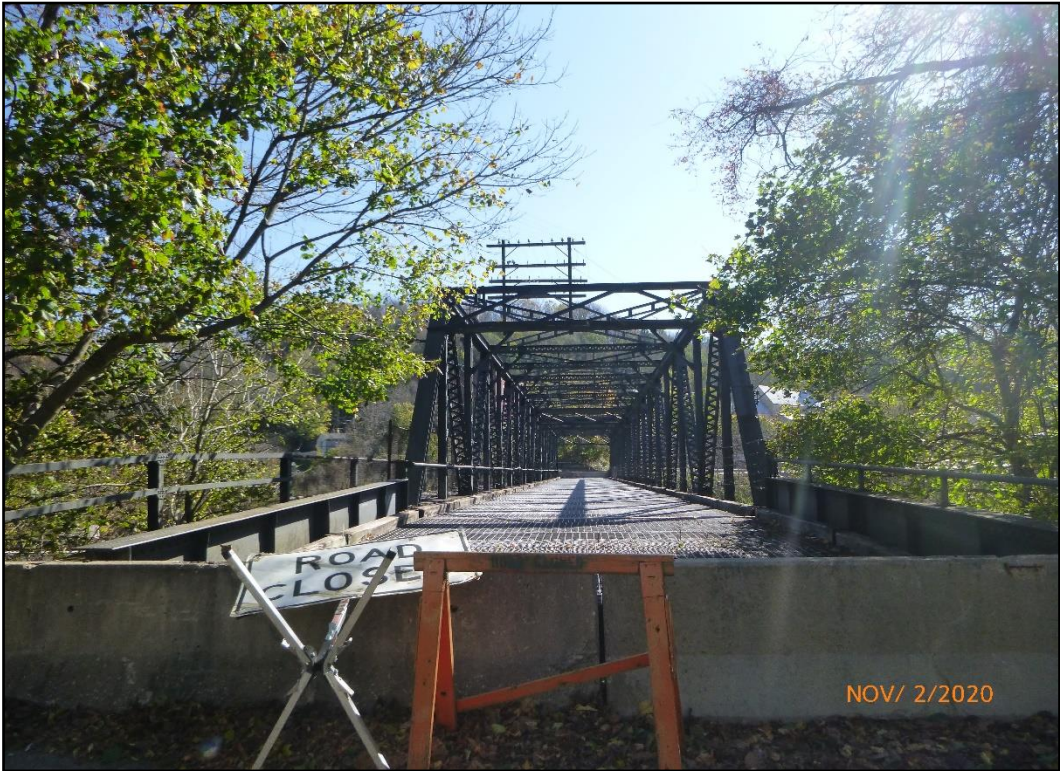
2. North approach. Photo: WVDOH November 2020.
