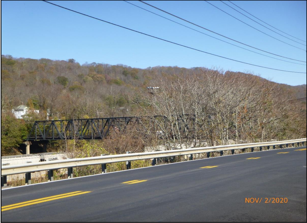
3. West elevation. Photo: WVDOH November 2020.
