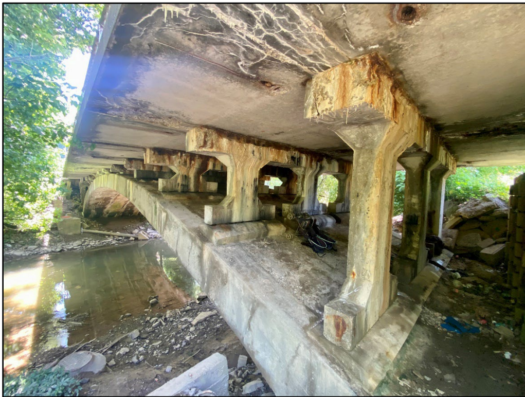
Photo 2: North (Upstream) Elevation. View South
