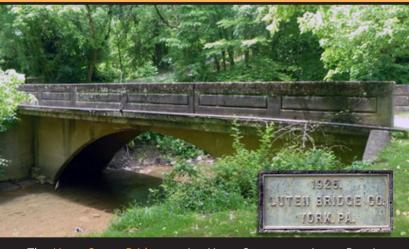
The Hope Street Bridge carries Hope Street over Jones Run in Harrison County. It is a single span spandrel-braced concrete arch with a total length of 49.2 feet total width of 16.2 feet. The arch rings feature flat beveled edges and are supported by concrete spread footers. The deck ends are supported by concrete abutments and wingwalls. The concrete parapets feature ornamentally incised rectangular panels on their inner and outer sides.
