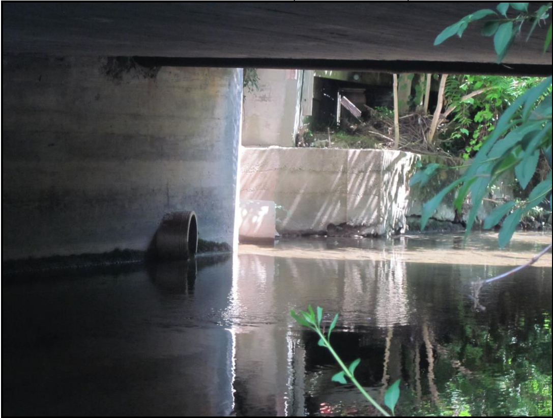
West Abutment, North End, with lower concrete retaining walls beyond. View N (WVDOH 6-28-2018)
