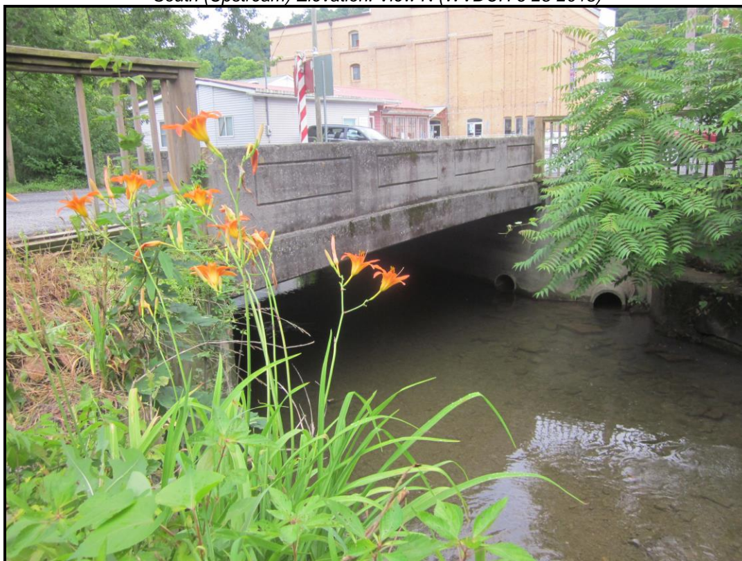
North (Downstream) Elevation. View SW (WVDOH 6-28-2018).
