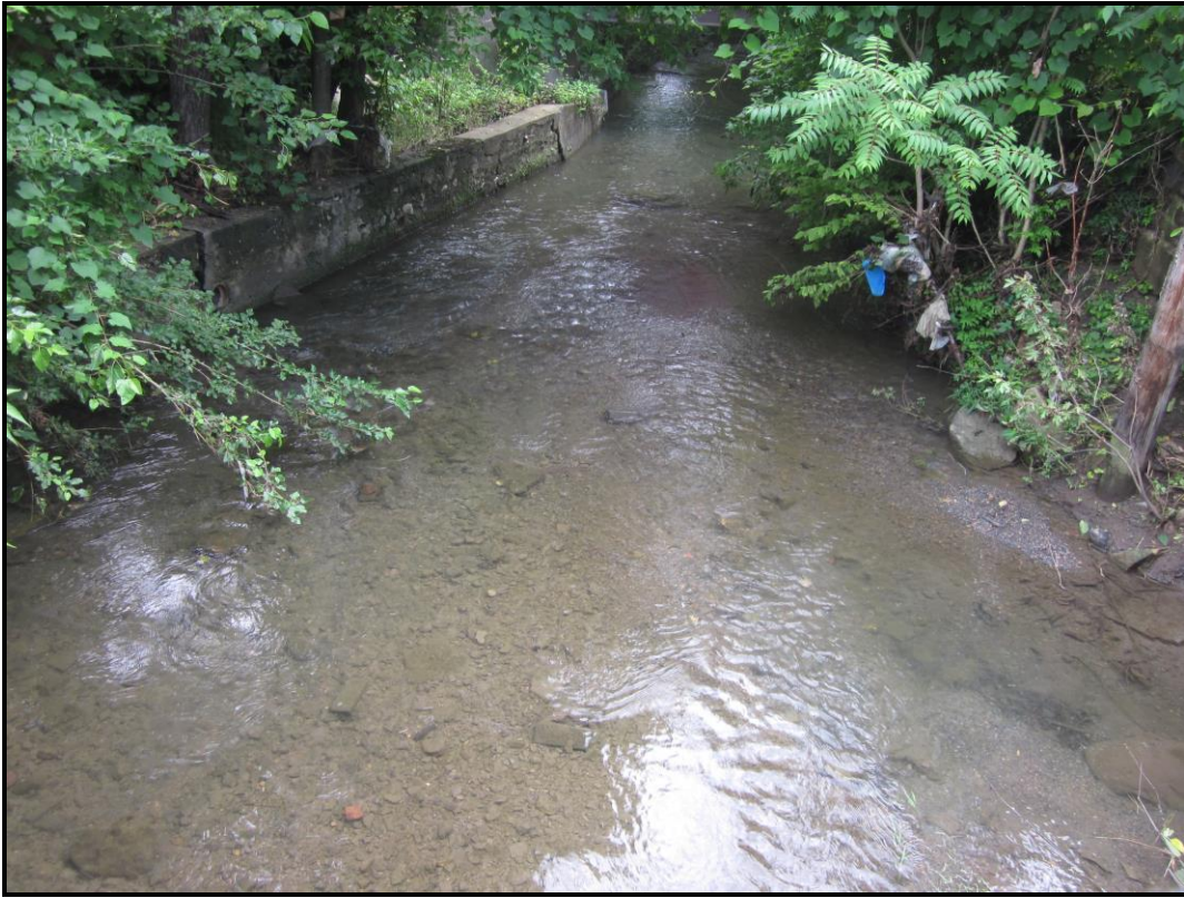
Warm Spring Run, North of Bridge/Abutments; the old Victor Products Plant is just north of this view. View NE (WVDOH 6-28-2018)
