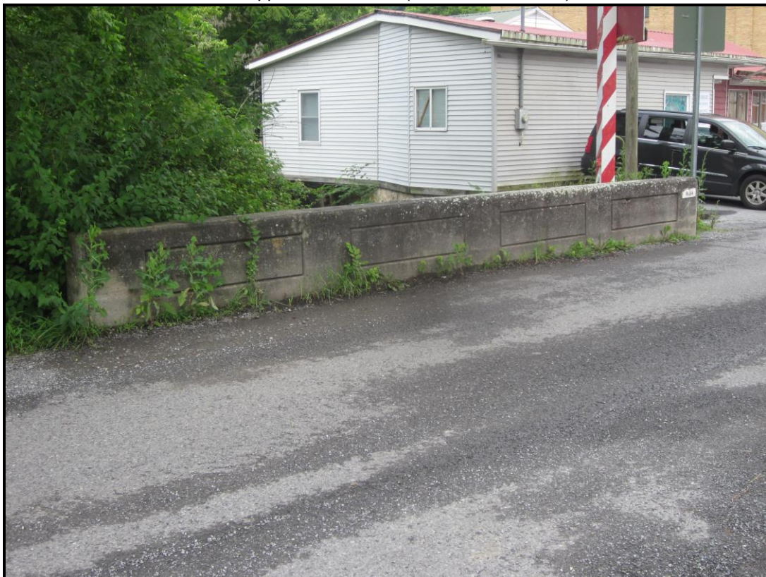
South (Upstream) Railing. View W (WVDOH 6-28-2018).
