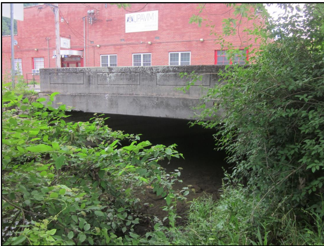
South (Upstream) Elevation. View N (WVDOH 6-28-2018)
