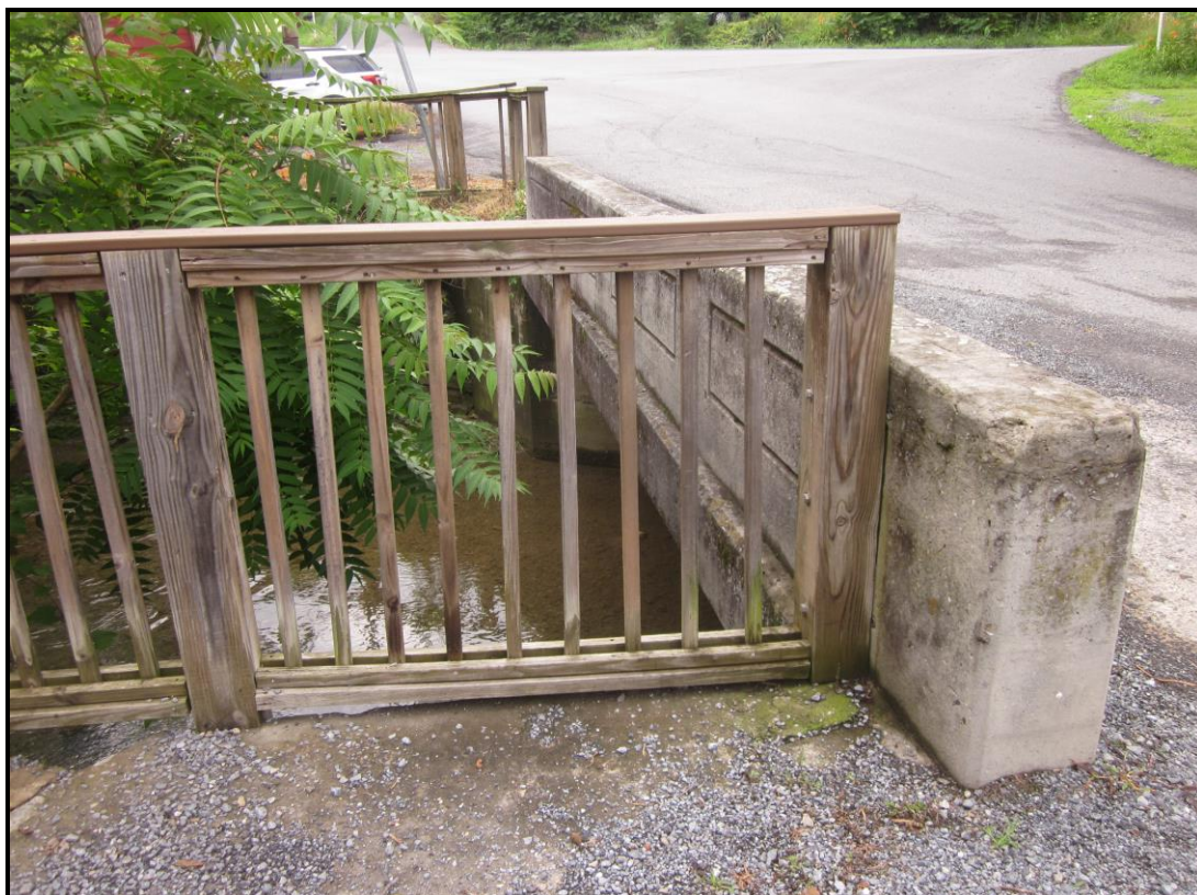
North (Downstream) Elevation. View SE (WVDOH 6-28-2018)
