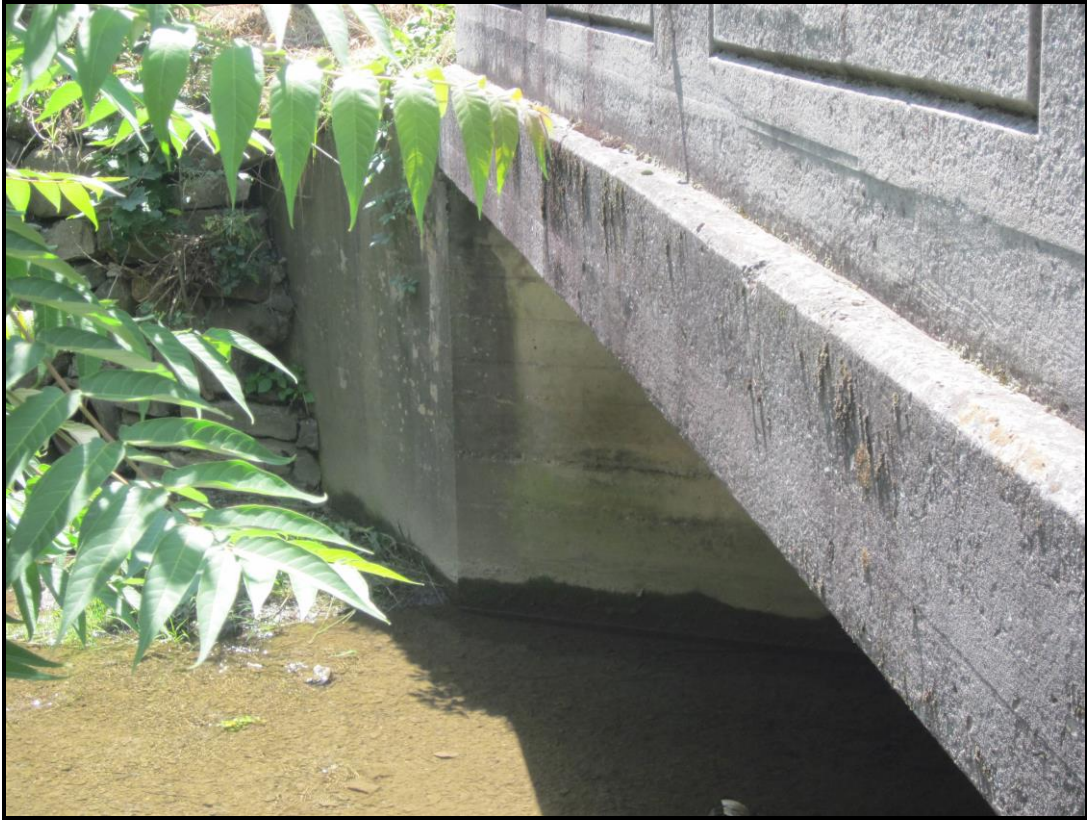
East Abutment, North Wingwall. View NE (WVDOH 6-29-2018)
