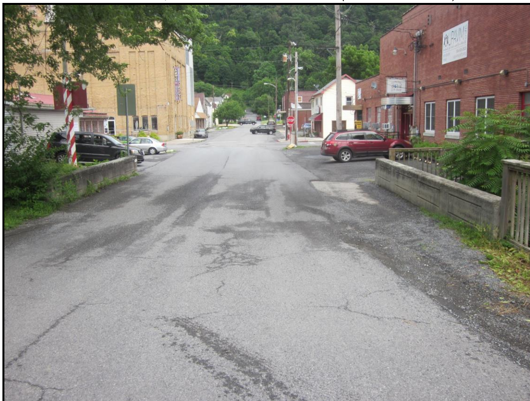
East Approach. View NW (WVDOH 6-28-2018).
