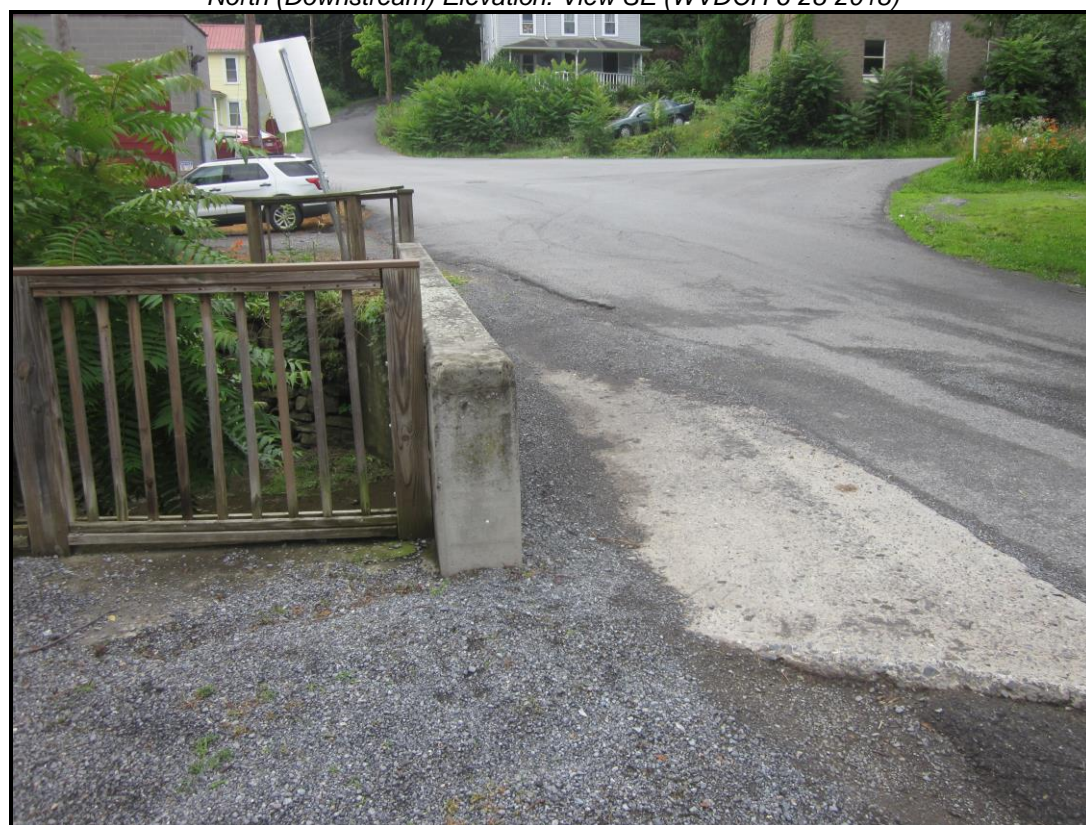
North (Downstream) Railing and Sidewalk. View SE (WVDOH 6-28-2018).
