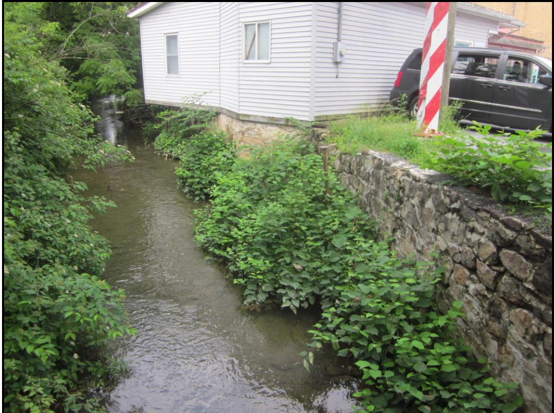
South Bank Stone Retaining Wall, Looking Southward from Bridge. View SW (WVDOH 5-28-2018)
