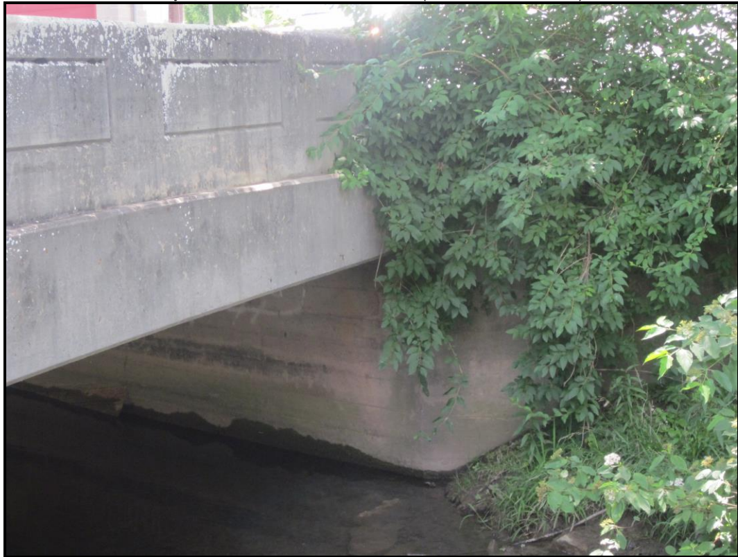
East Abutment, South Wingwall (stone). View East (WVDOH 6-29-2018)
