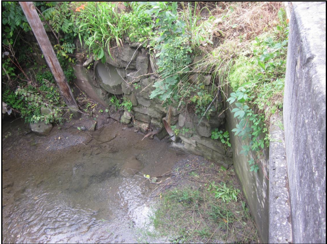
Stone Retaining Wall (with two pipe outlets), Next to North Wingwall of East Abutment. View East (WVDOH 6-29-2018)
