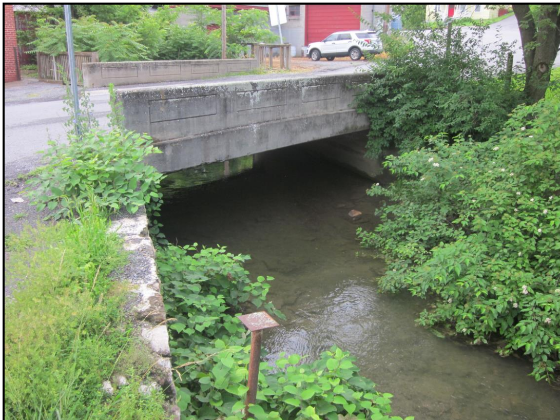
South (Upstream) Elevation. View NE (WVDOH 6-28-2018).
