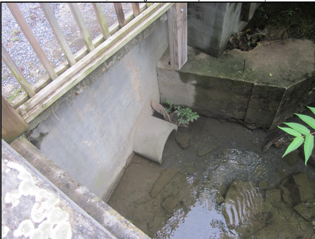
North Wingwall of West Abutment; lower concrete retaining wall in upper right corner head toward the old Victor Products Corp Plant. View NW (WVDOH 6-29-2018).
