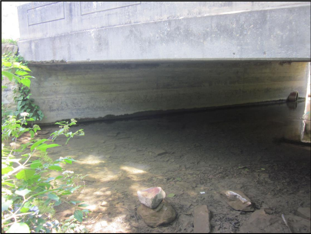
West Abutment. View NW (WVDOH 6-29-2018).
