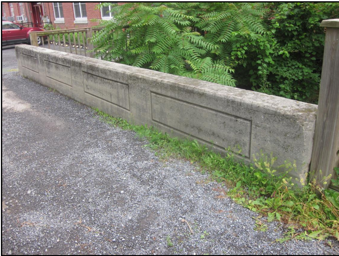
North (Downstream) Railing. View WNW (WVDOH 6-28-2018)
