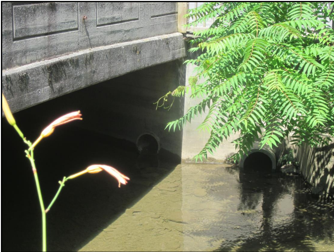
West Abutment, North Wingwall. View NW (WVDOH 6-29-2018)
