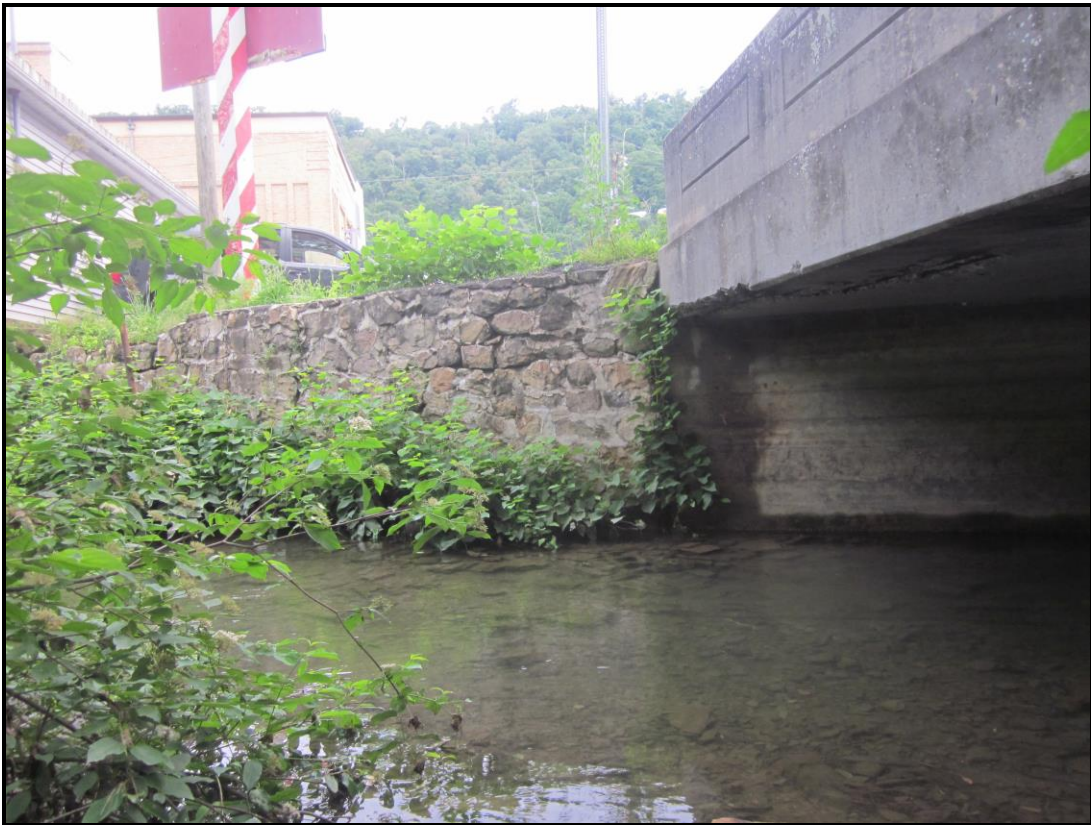
West Abutment and South Bank Stone Retaining Wall. View NW (WVDOH 6-29-2018)
