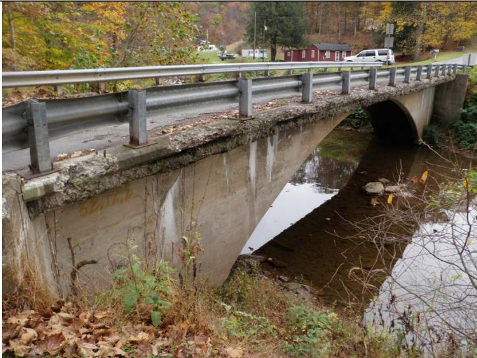
3. Concrete deterioration along downstream side of deck
