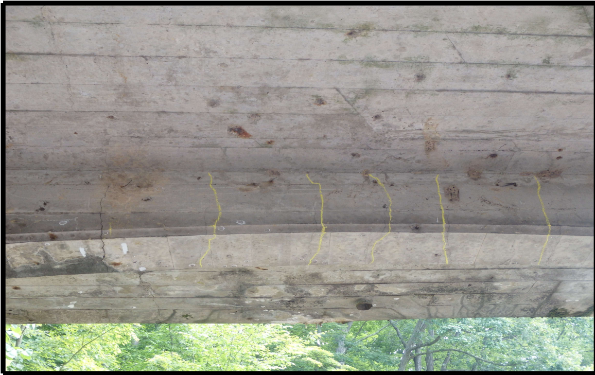
PHOTO NO. 1 - HAIRLINE TO 1/8" CRACKS I THE UPSTREAM GIRDER
