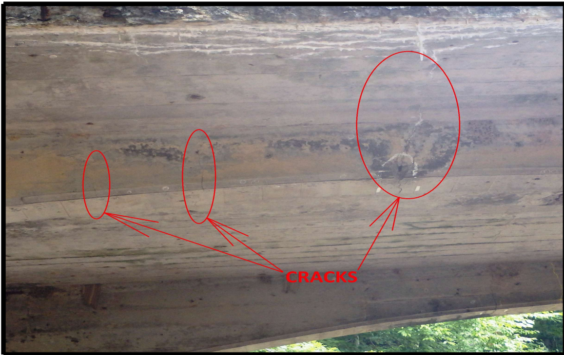
PHOTO NO. 3 - HAIRLINE TO 18" CRACKS IN THE DOWNSTREAM GIRDER
