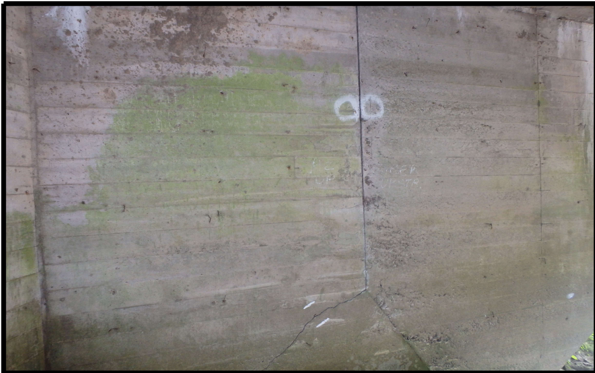
PHOTO NO. 6 - UP TO 1/4" SEPERATION IN UPSTREAM GIRDER AT ABUTMENT NO. 2
