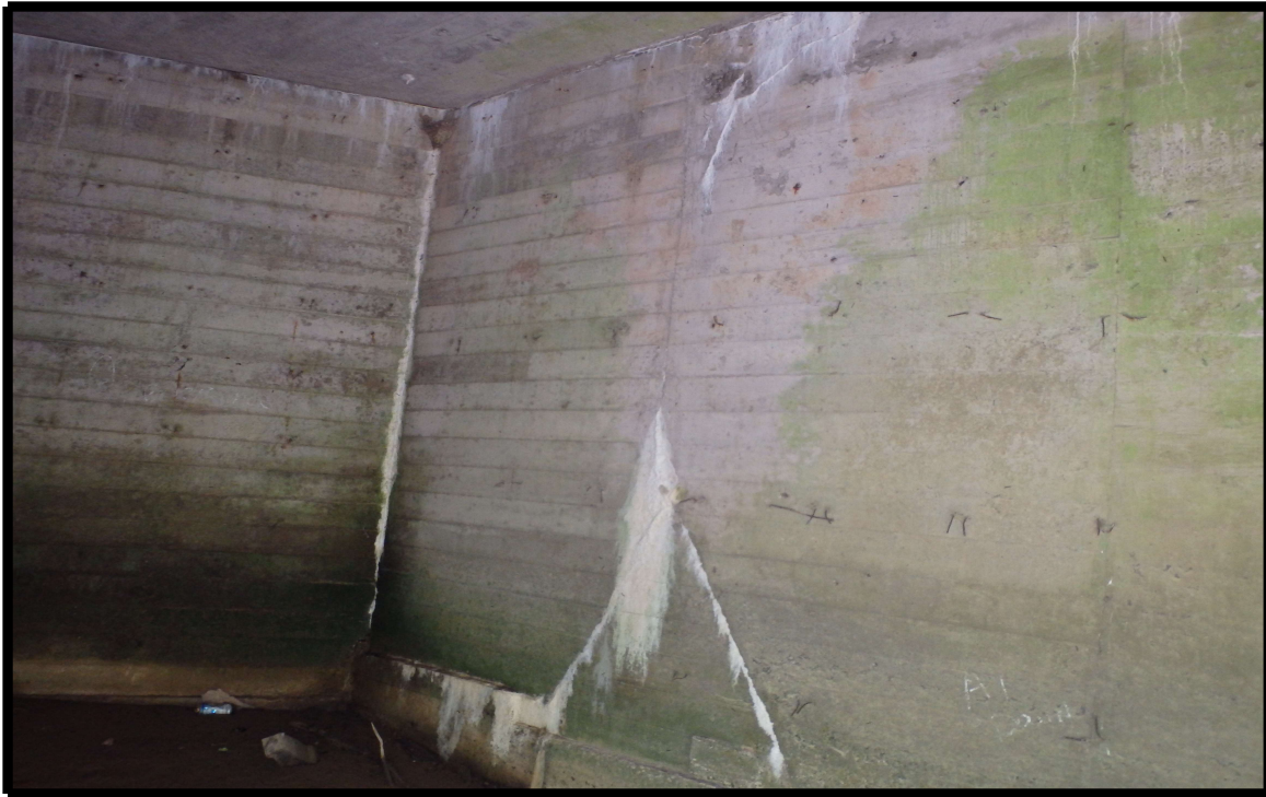
PHOTO NO. 5 - CRACKS WITH EFFLORESCENCE DOWNSTREAM GIRDER NEAR ABUTMENT NO. 1
