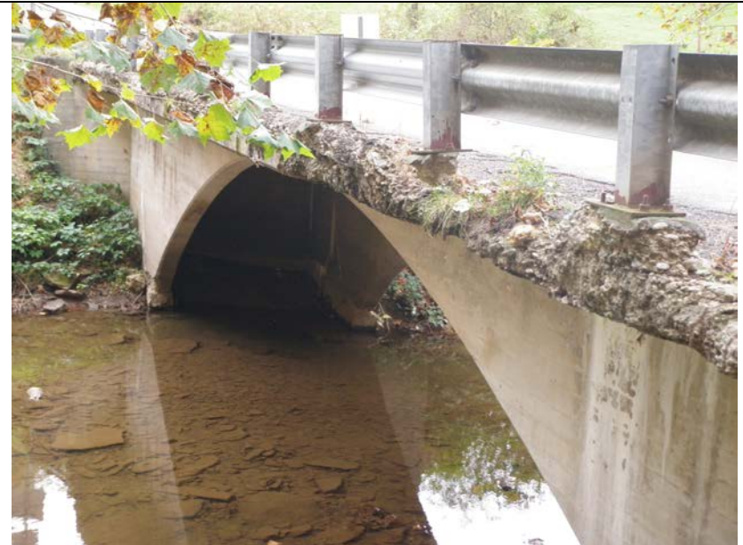
8. Looking inside arch at Abutment #1
