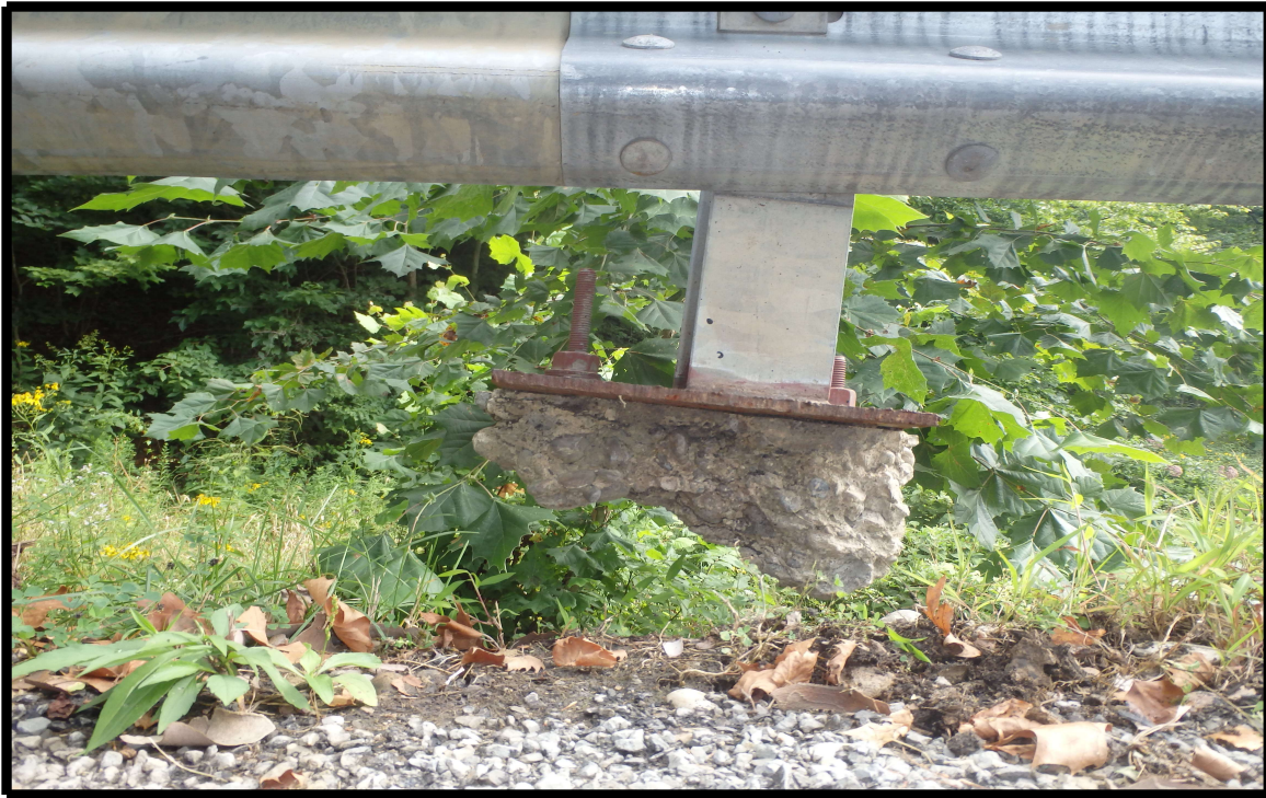
PHOTO NO. 7 - DETACHED GUARDRAIL POST
