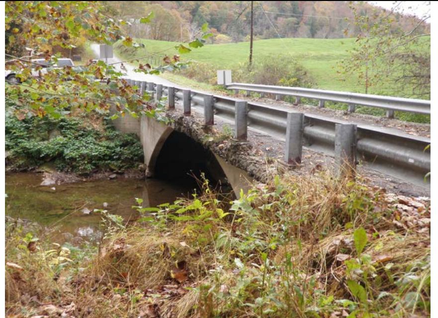
2. End view looking southwest
