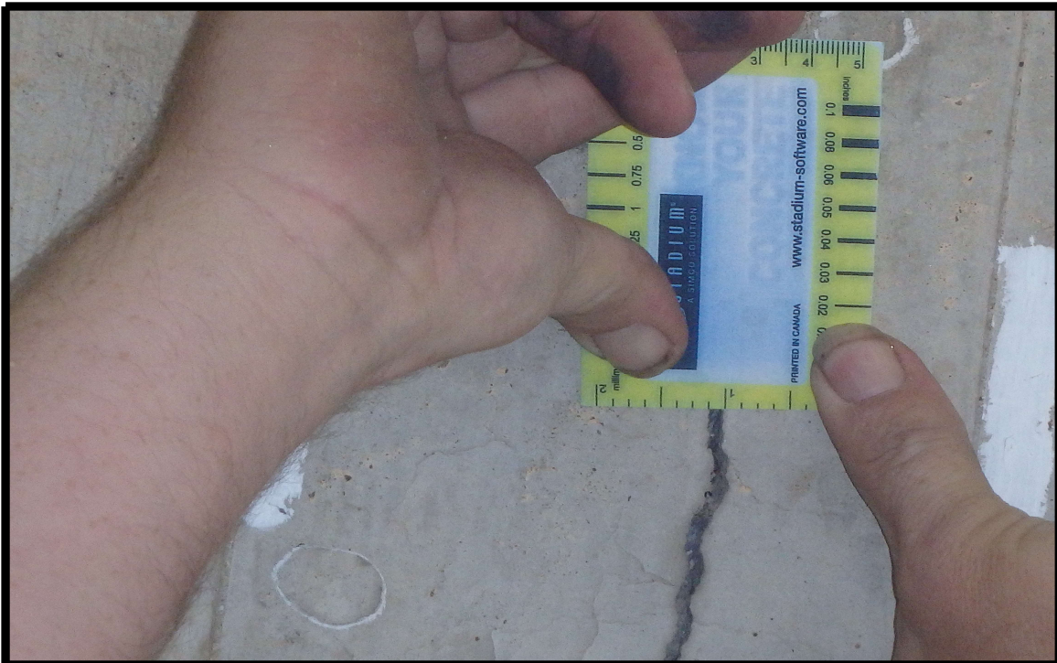
PHOTO NO. 2 - 1/8" CRACK IN THE UPSTREAM GIRDER
