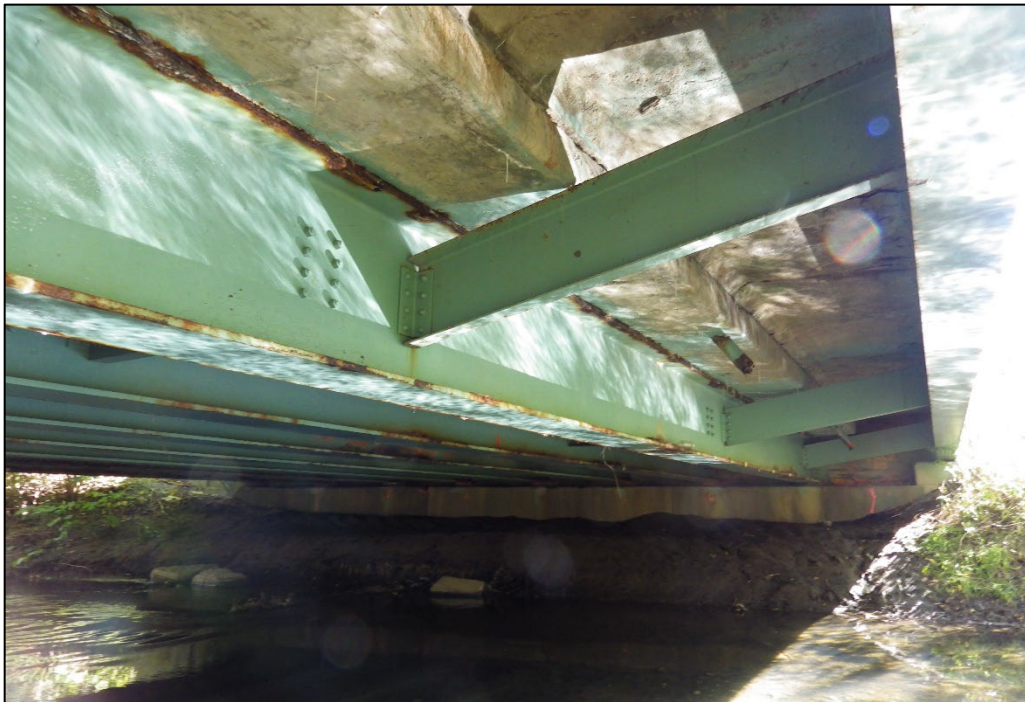
Photograph 10. Matoaka Bridge No. 1, view of steel stringers and south abutment, facing south.
