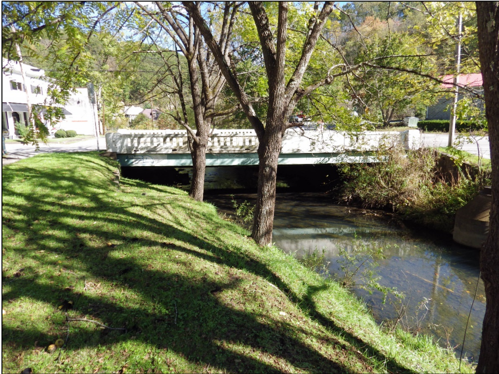
Photograph 3. Matoaka Bridge No. 1, upstream elevation, facing east.
