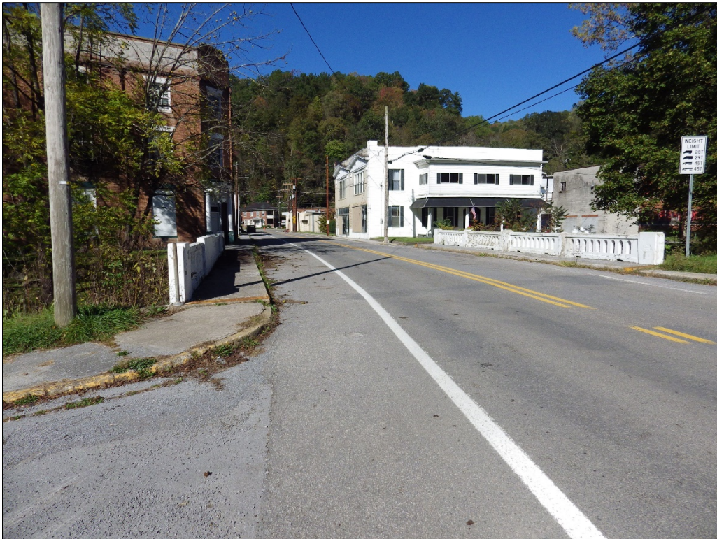
Photograph 6. Matoaka Bridge No. 1, through view of travel lanes, facing north.
