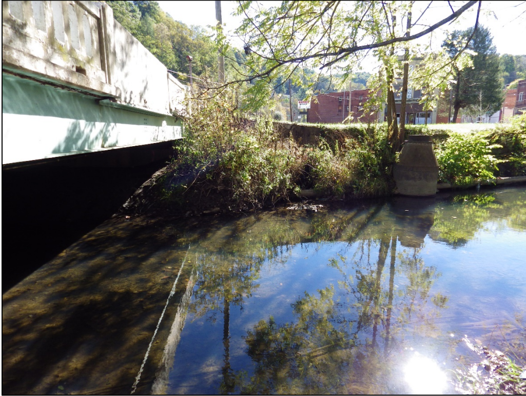
Photograph 5. Matoaka Bridge No. 1, west elevation, upstream view, facing south.
