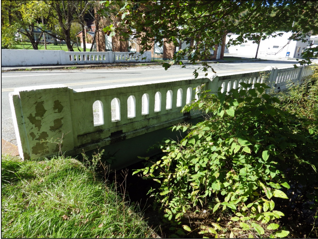
Photograph 1. Matoaka Bridge No. 1, parapet wall, downstream elevation, facing northwest.
