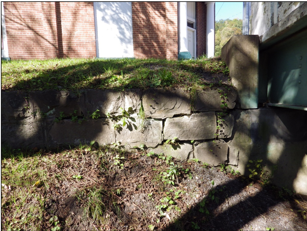
Photograph 8. Matoaka Bridge No. 1, view of north abutment, facing north.
