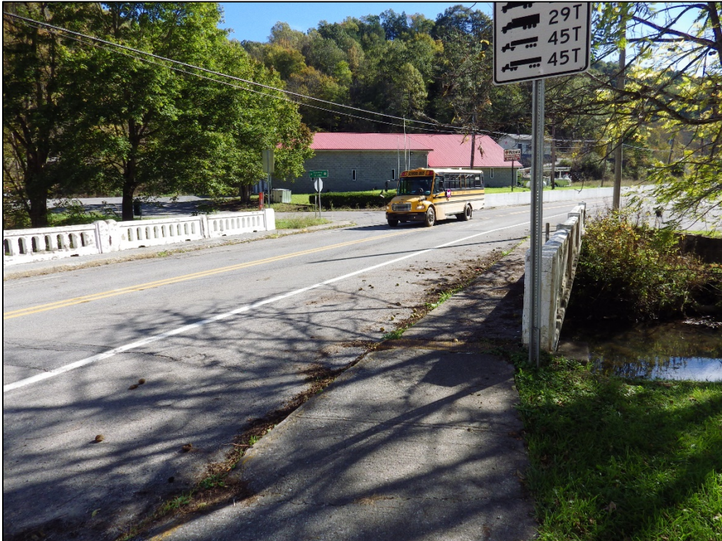
Photograph 4. Matoaka Bridge No. 1, travel lanes and parapets facing south.
