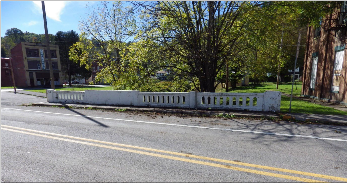
Photograph 11. Matoaka Bridge No. 1, general view, facing southwest.
