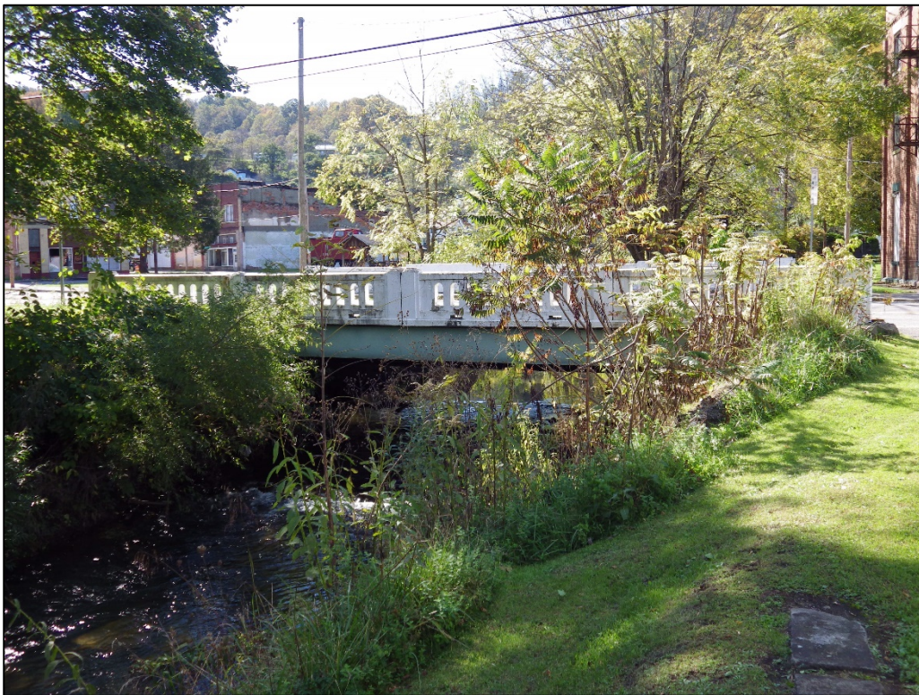
Photograph 2. Matoaka Bridge No. 1, downstream elevation, parapet wall and steel stinger, facing west.
