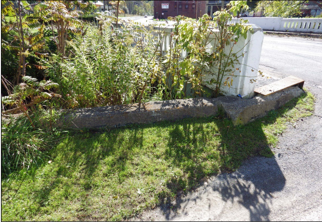
Photograph 7. Matoaka Bridge No. 1, view of breast wall, abutment, newel, and parapet, facing southwest.
