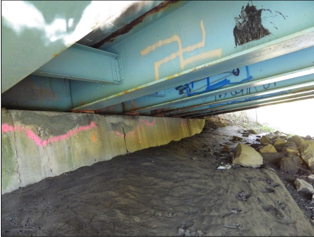
Photograph 9. Matoaka Bridge No. 1, view of steel stringers, bearings, and braces of north abutment, facing northeast.
