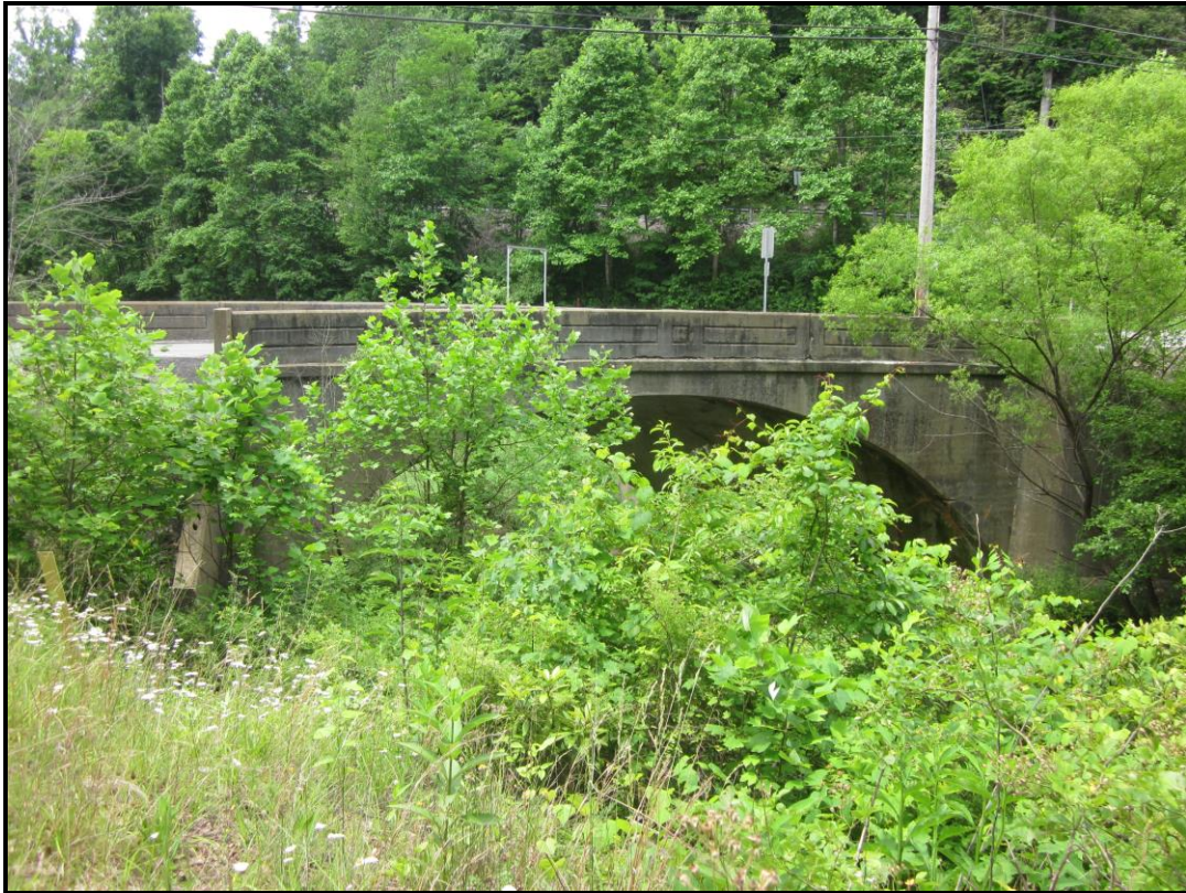
Milam Arch Bridge – North (Upstream) Elevation. View SW (WVDOH 6-12-2017).
