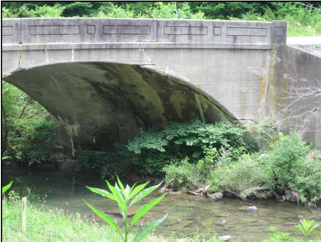
Milam Arch Bridge – South (Downstream) Elevation – Abutment Detail. View NE (WVDOH 6-12-2017).
