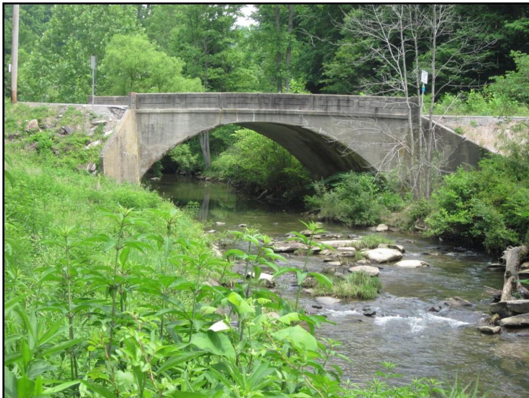
Milam Arch Bridge, built 1925. South (Downstream) Elevation. View NNE (WVDOH 6-12-2017)
