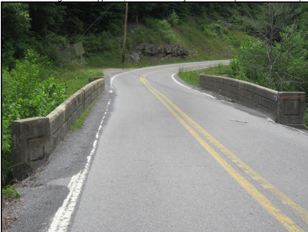
Milam Arch Bridge – North (Upstream) Elevation & East Approach. View Southwest (WVDOH 6-12-2017).
