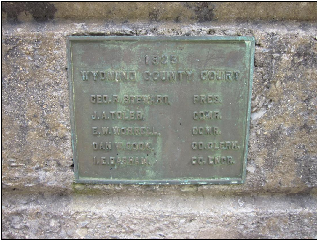
Milam Arch Bridge – Plaque at West End of South Railing. View SW (WVDOH 6-12-2017).
