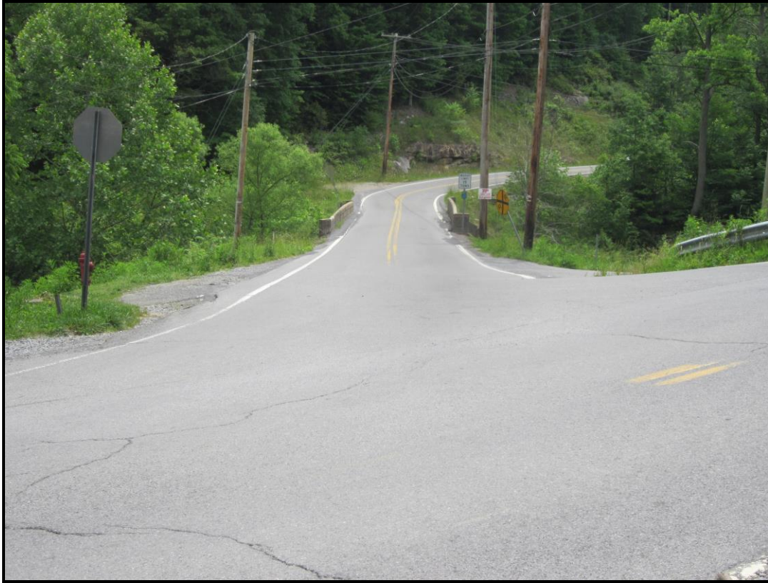
Milam Arch Bridge – West Approach, taken from County Rt 1. View SE (WVDOH 6-12-2017).
