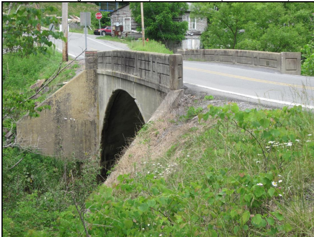
Milam Arch Bridge – South (Downstream) Elevation & East Approach. View NW (WVDOH 6-12-2017).
