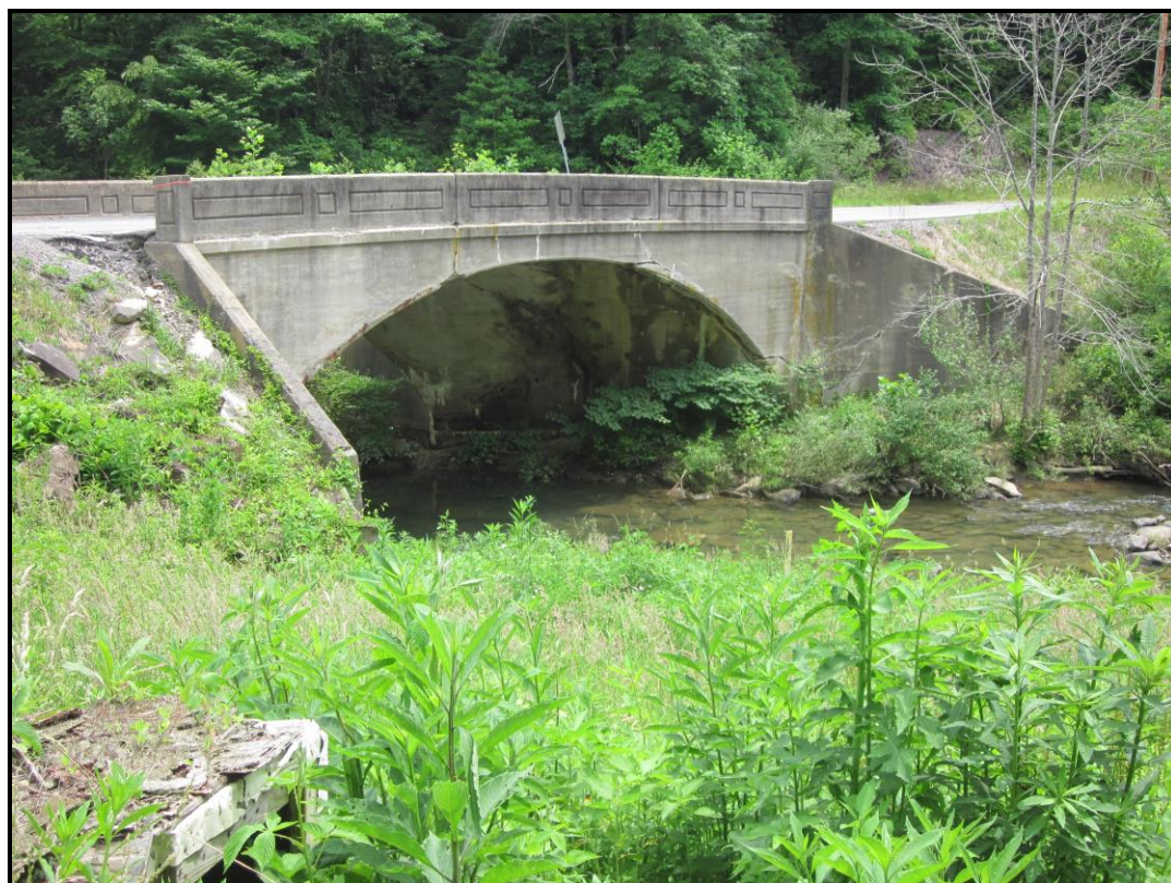
Milam Arch Bridge – South (Downstream) Elevation. View NE (WVDOH 6-12-2017).
