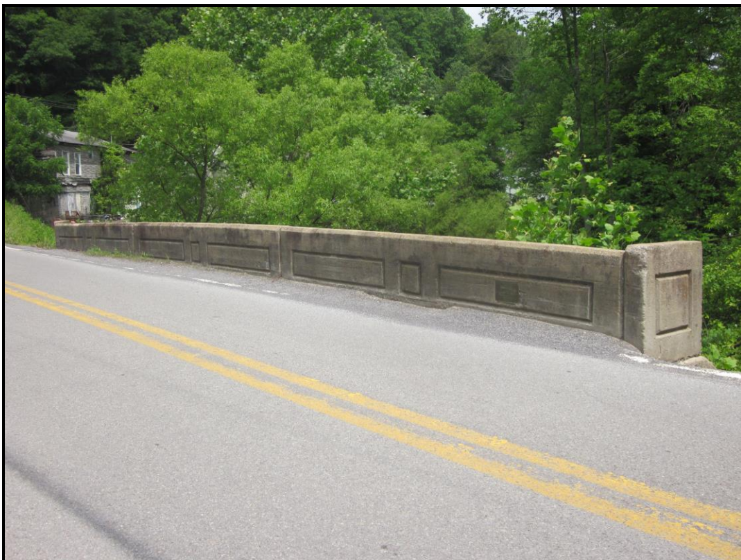
Milam Arch Bridge – North Parapet Railing. View NW (WVDOH 6-12-2017).
