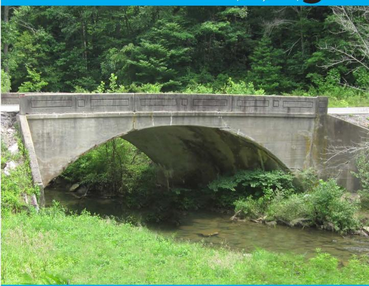
**Location:** County Route 5, east of County Route 1, spanning Laurel Fork **Type:** Reinforced Concrete Closed Spandrel Elliptical Arch Span
