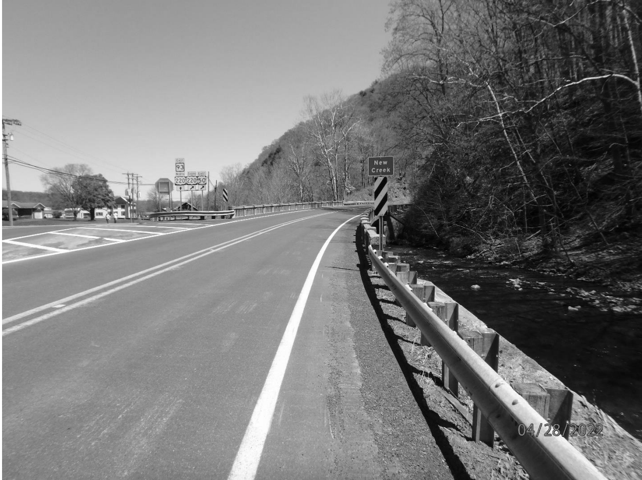
Photo #4 New Creek Bridge Mineral County US Route 50, spanning New Creek Looking east at New Creek Bridge
