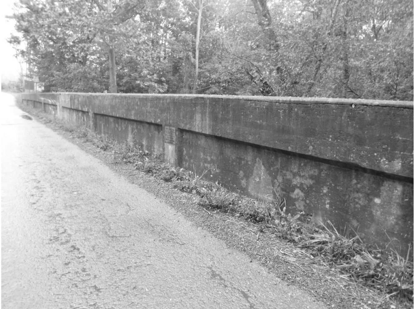
Photo #3 Pallet Factory Bridge Morgan County County Route 13, spanning Sleepy Creek View of parapet wall with bridge plaque in the center
