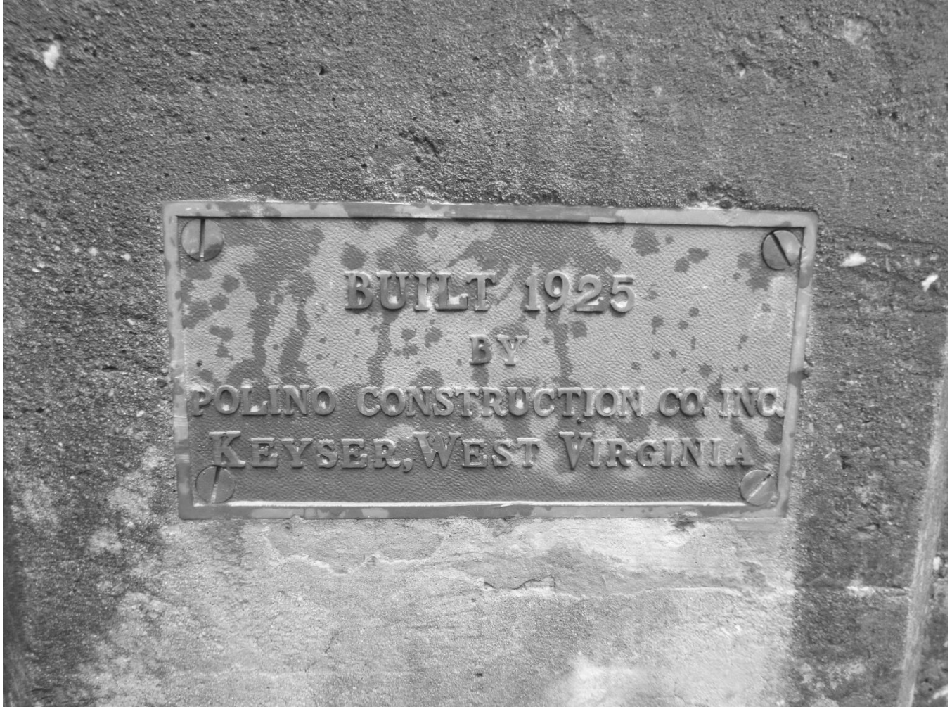
Photo #5 Pallet Factory Bridge Morgan County County Route 13, spanning Sleepy Creek Bridge builder plaque
