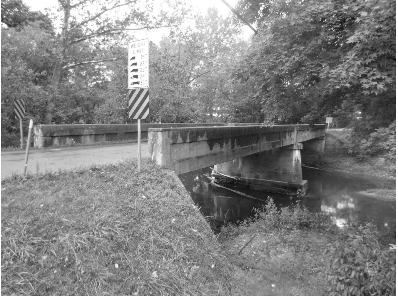
Photo #4 Pallet Factory Bridge Morgan County County Route 13, spanning Sleepy Creek Looking upstream at Pallet Factory Bridge
