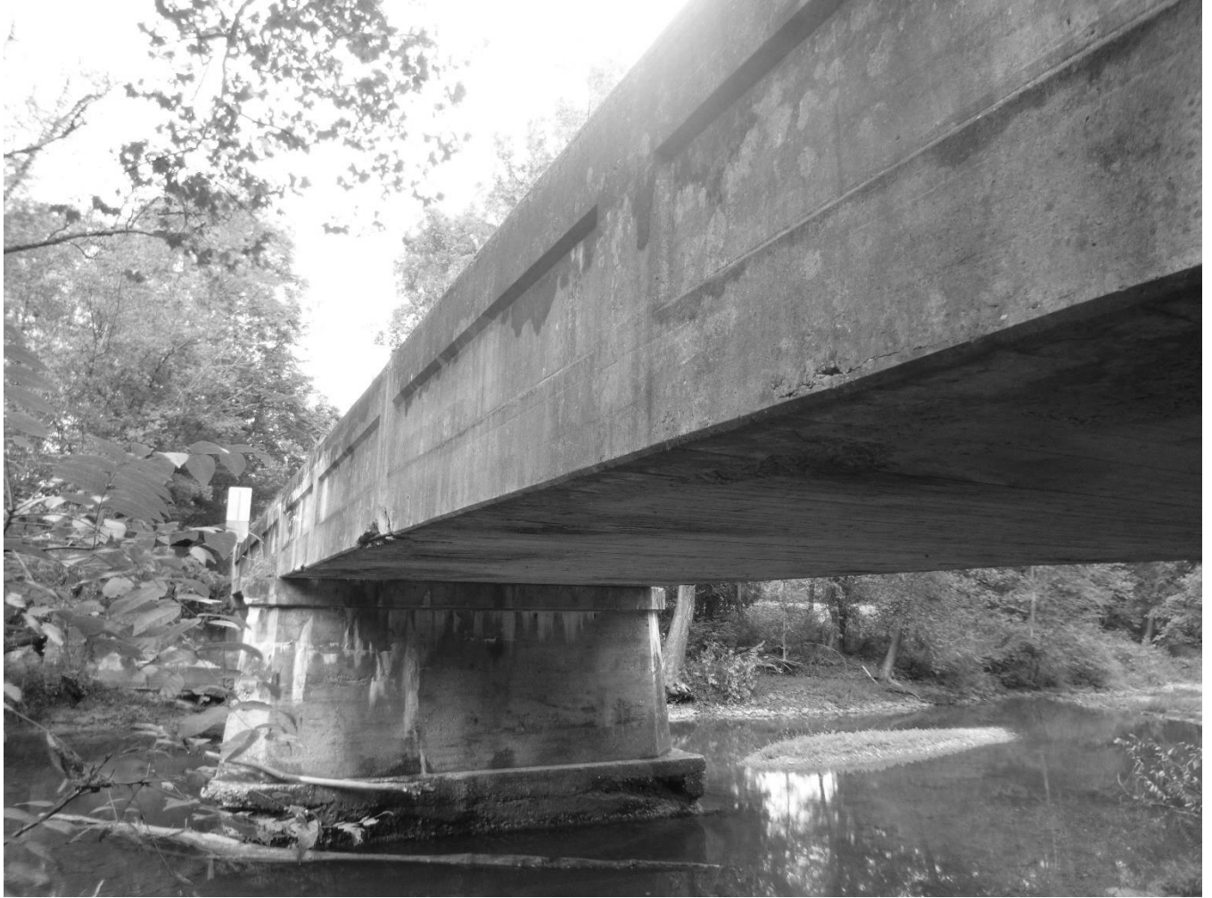
Photo #8 Pallet Factory Morgan County County Route 13, spanning Sleepy Creek Downstream view showing pier and superstructure
