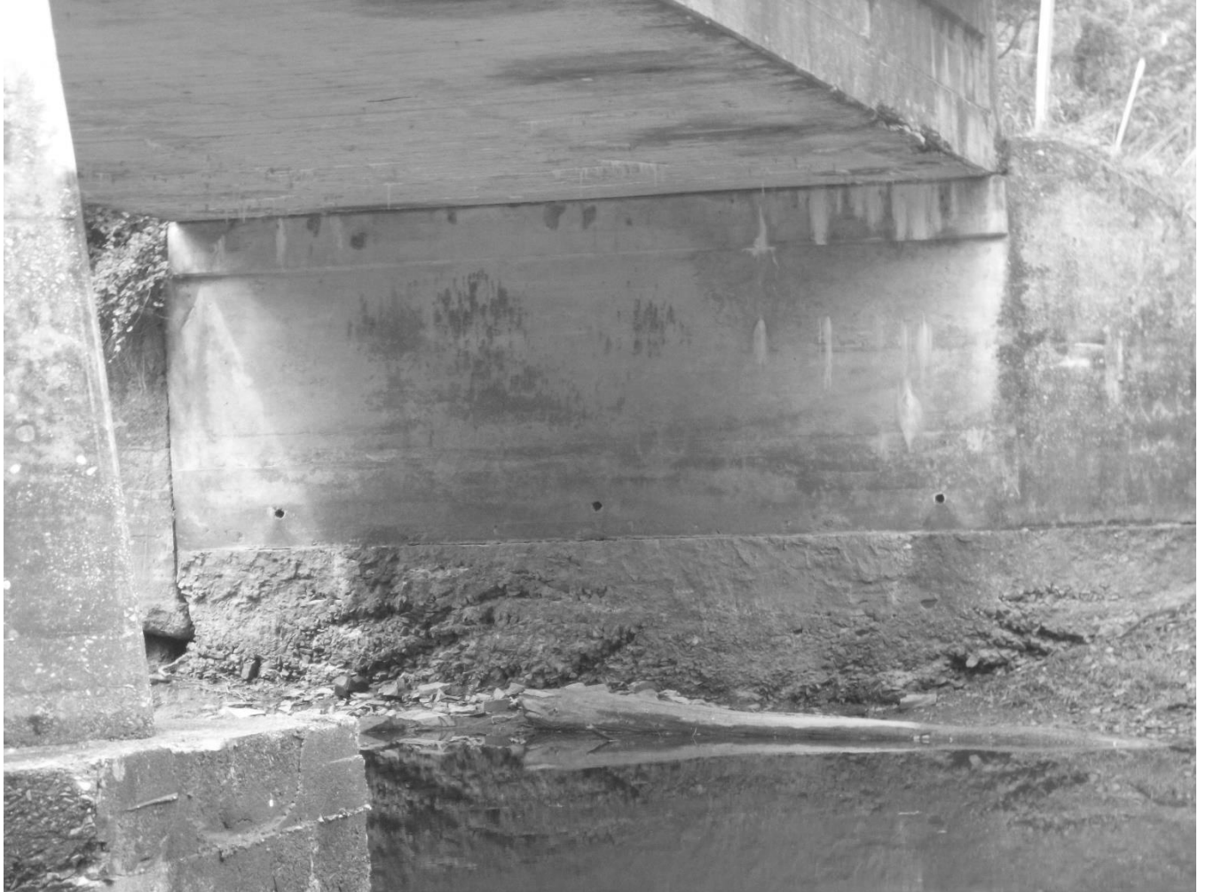
Photo #7 Pallet Factory Bridge Morgan County County Route 13 View of abutment and underside of bridge
