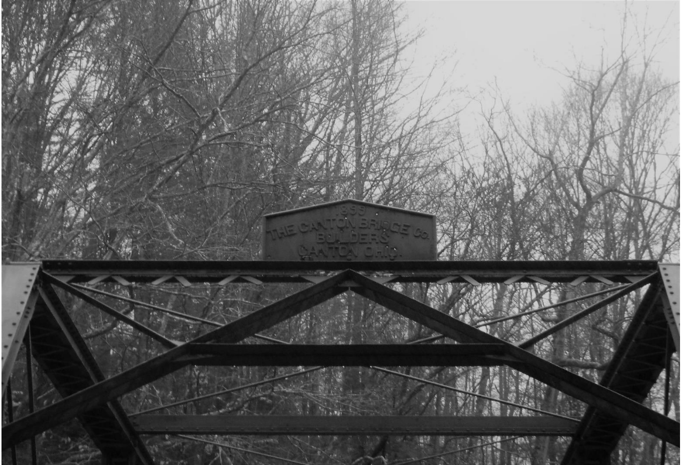
Photo #3 Pocatalico River Road Truss Roane County County Route 34, spanning the Pocatalico River Bridge builder plaque.
