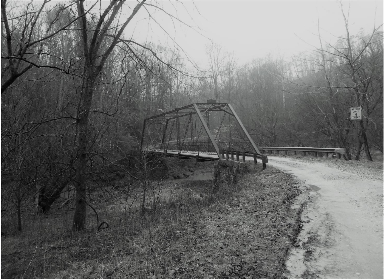
Photo #1 Pocatalico River Road Truss Roane County County Route 34, spanning the Pocatalico River View southwest toward Pocatalico River Road Truss Bridge.
