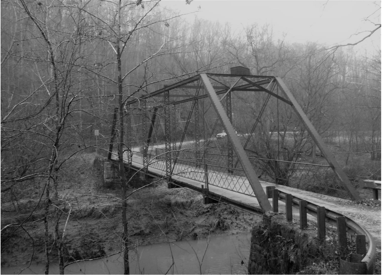
Photo #4 Pocatalico River Road Truss Roane County County Route 34, spanning the Pocatalico River View southwest toward Pocatalico River Road Truss Bridge.
