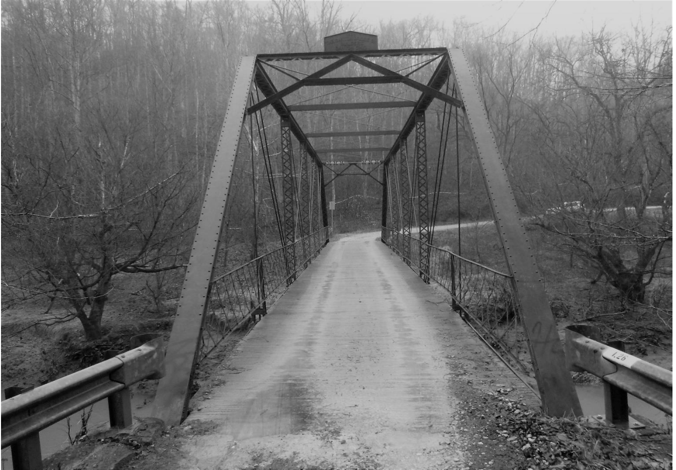
Photo #2 Pocatalico River Road Truss Roane County County Route 34, spanning the Pocatalico River View south toward Pocatalico River Road Truss Bridge.
