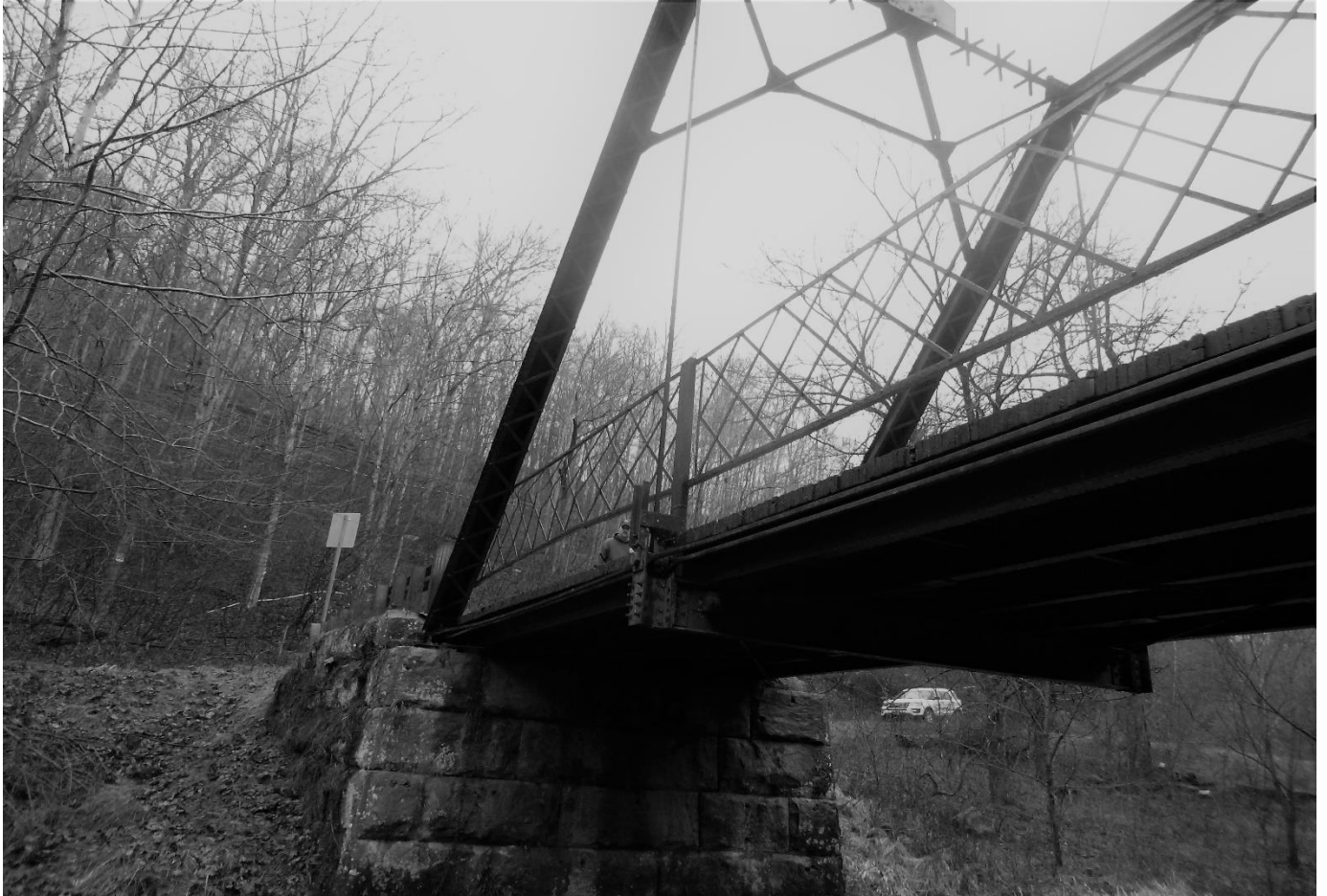
Photo #5 Pocatalico River Road Truss Roane County County Route 34, spanning the Pocatalico River View of the abutments, substructure, and parapets.
