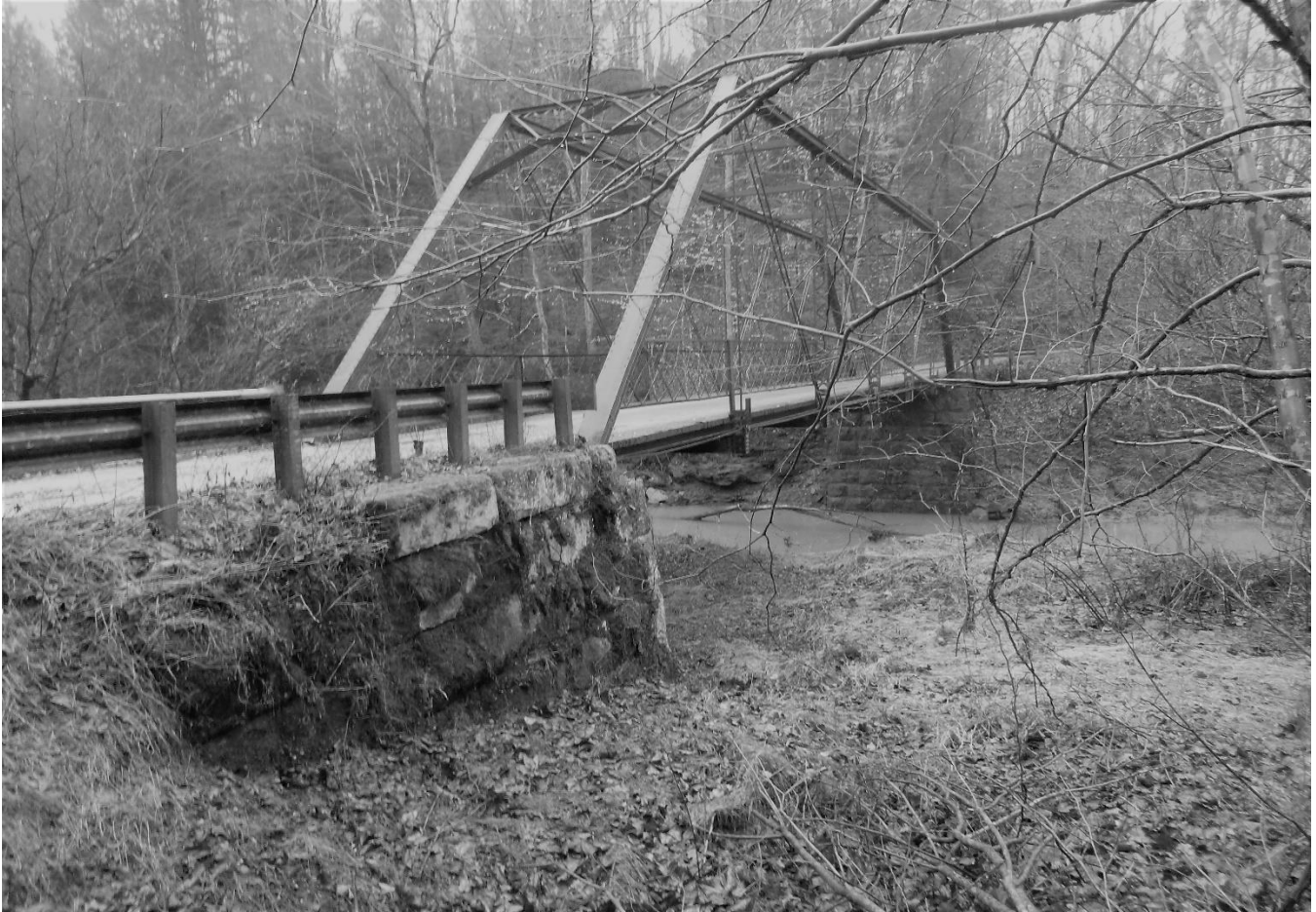
Photo #6 Pocatalico River Road Truss Roane County County Route 34, spanning the Pocatalico River View southeast toward Pocatalico River Road Truss Bridge.
