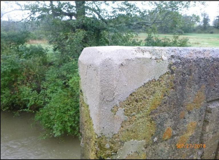
11. Repair to north parapet corner of east abutment. (Photo: WVDOH September 2018)
