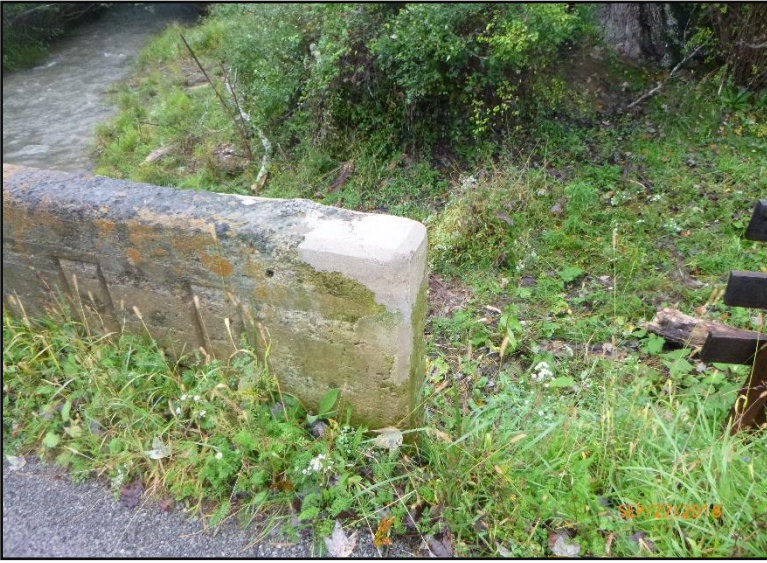
9. Repair to north parapet corner of west abutment. (Photo: WVDOH September 2018)
