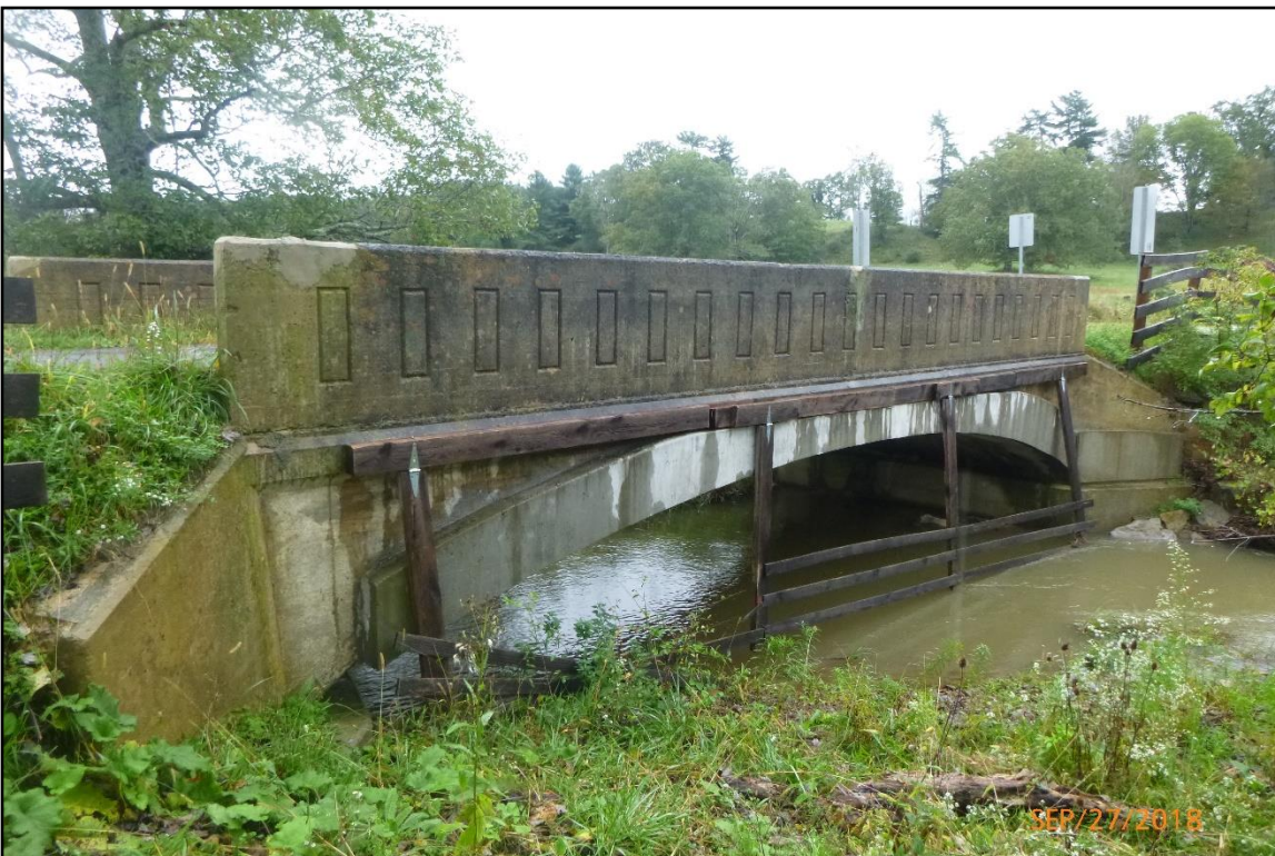
Elevation view, downstream (west) side. (Photo WVDOH, September 2018)
