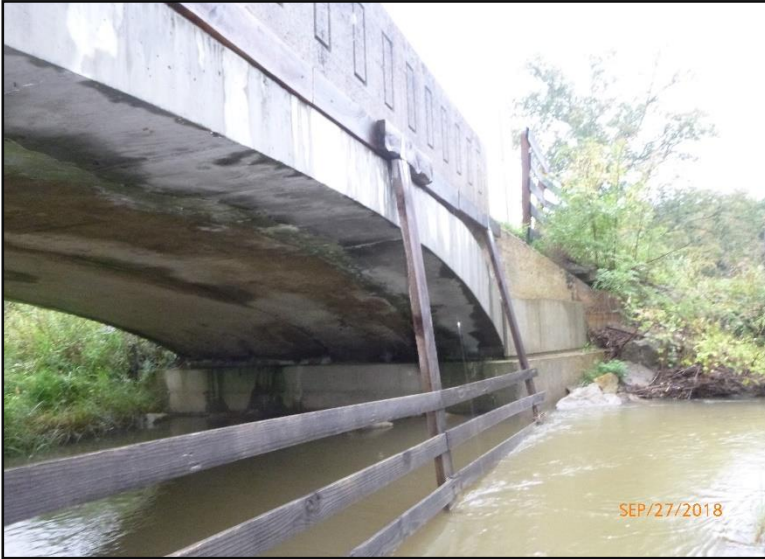
5. View of south abutment, showing alterations, including collar around the abutment, repairs to the arch ring, and wooden cattle guard. (Photo: WVDOH September 2018)
