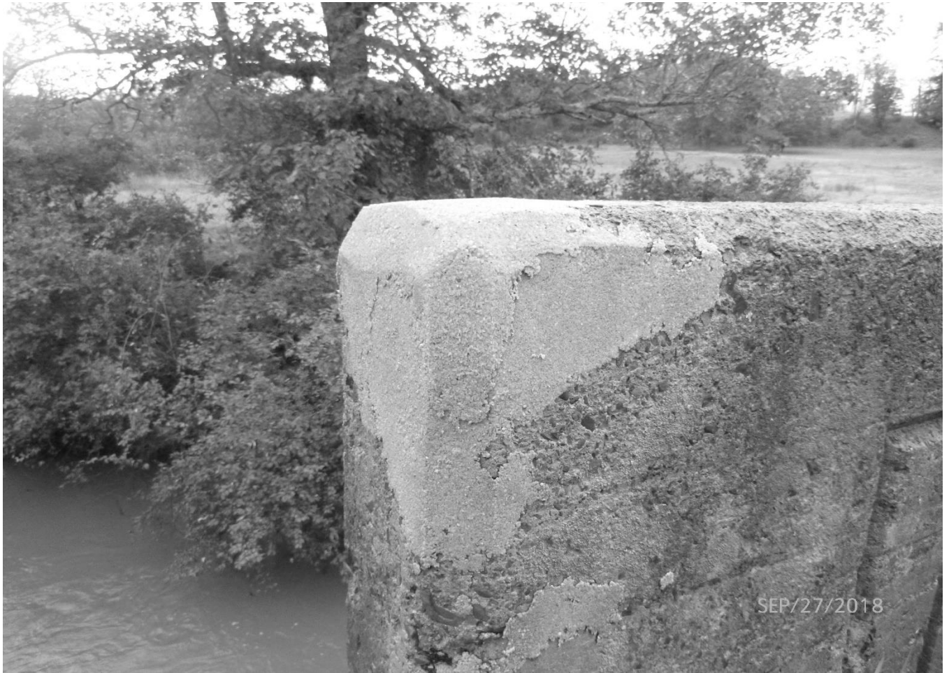
Photo 11 Saulsbury Run Arch Bridge Pocahontas County County Route 4/1 spanning Saulsbury Run Repair to north parapet corner of east abutment
