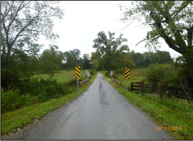
1. North approach to bridge, view south. (Photo: WVDOH September 2018)
