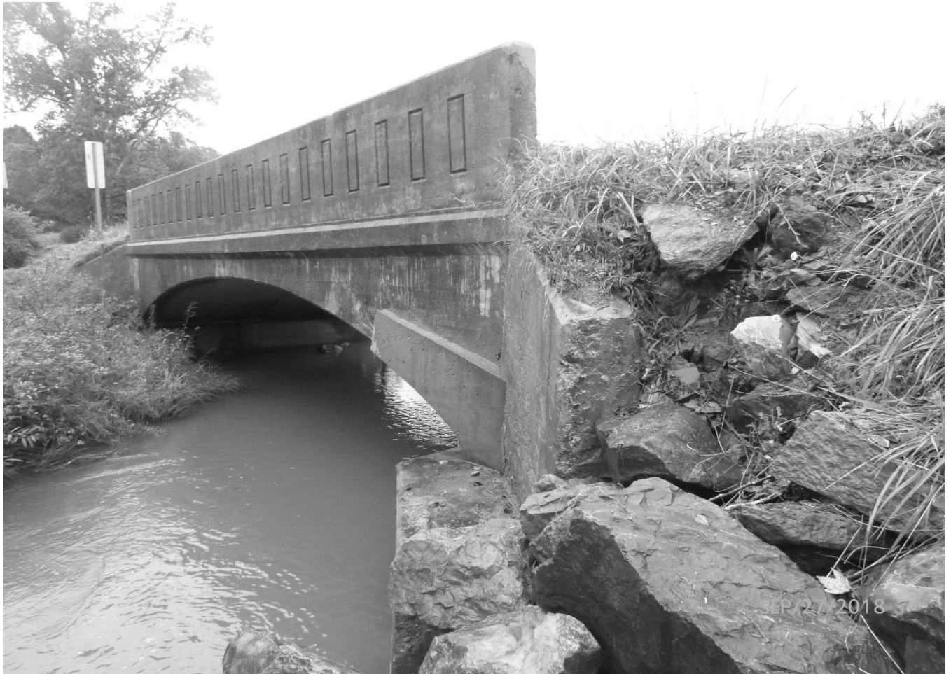
Photo 3 Saulsbury Run Arch Bridge Pocahontas County County Route 4/1 spanning Saulsbury Run Upstream elevation
