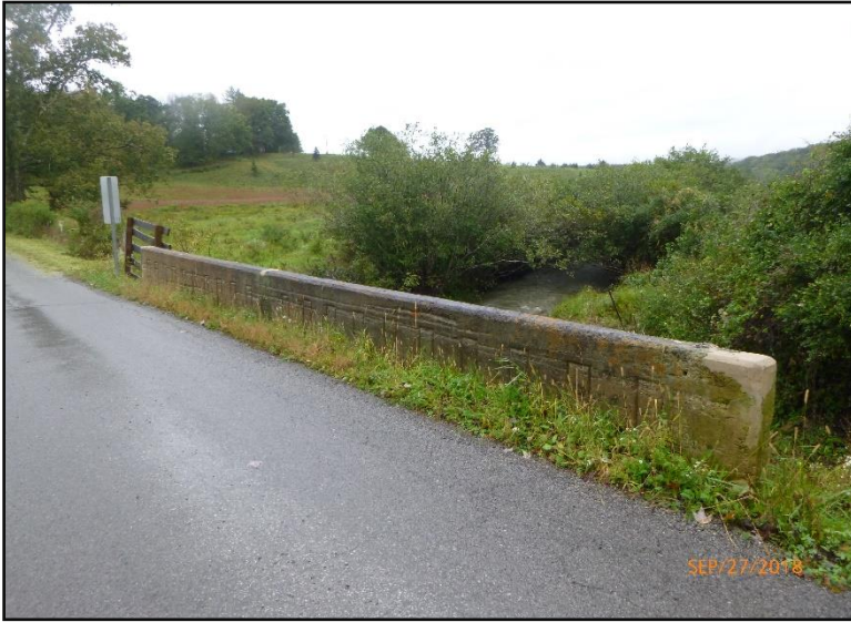
13. West parapet. (Photo: WVDOH September 2018)
