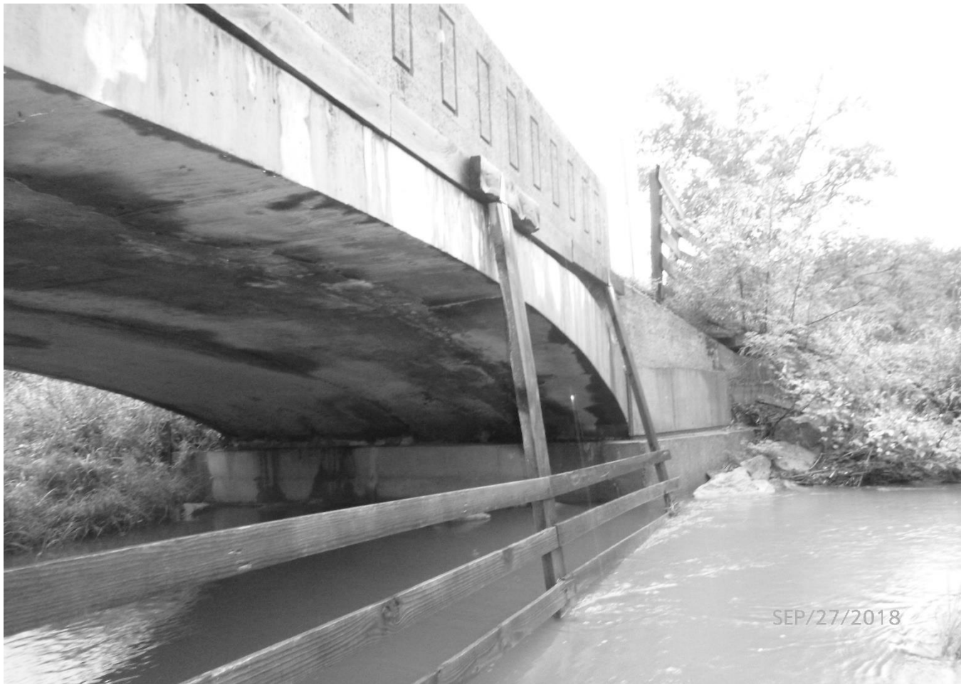
Photo 5 Saulsbury Run Arch Bridge Pocahontas County County Route 4/1 spanning Saulsbury Run View of south abutment, showing alterations, including collar around the abutment, repairs to the arch ring, and wooden cattle guard
