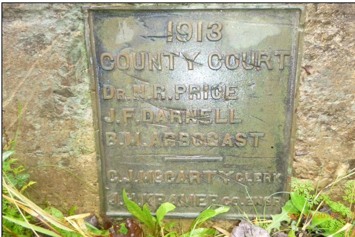
Detail: bridge plaque (Photo WVDOH, September 2018)
