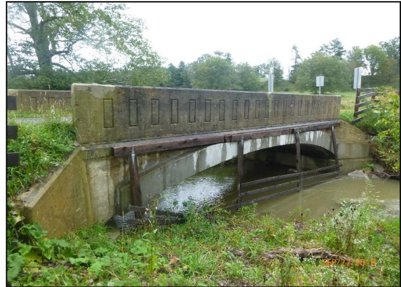
4. Downstream elevation. (Photo: WVDOH September 2018)
