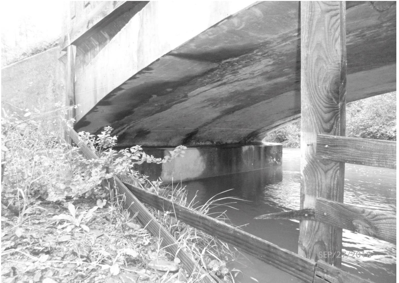
Photo 6 Saulsbury Run Arch Bridge Pocahontas County County Route 4/1 spanning Saulsbury Run View of north abutment
