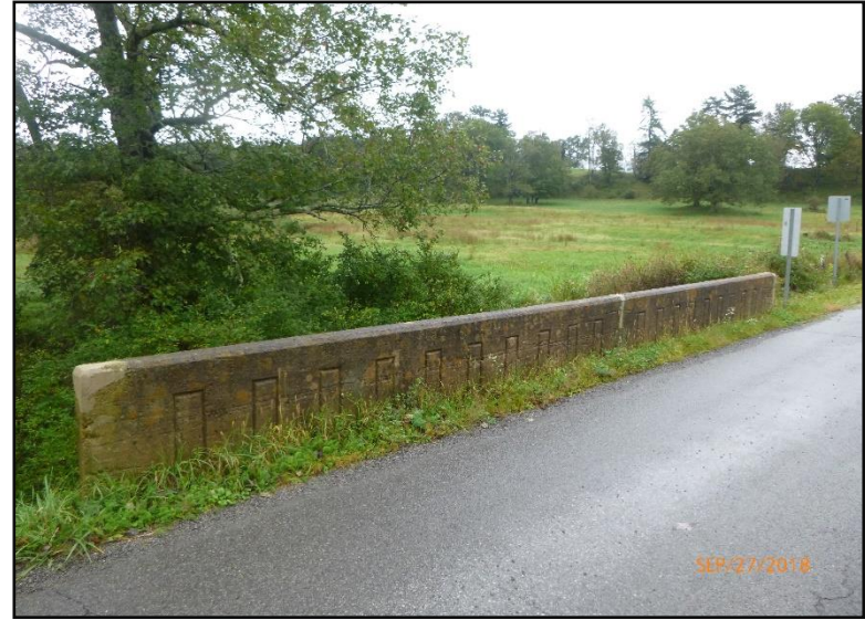
14. East parapet. (Photo: WVDOH September 2018)
