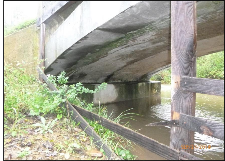
6. View of north abutment. (Photo: WVDOH September 2018)
