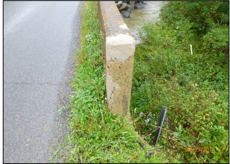
12. Repair to south parapet corner of east abutment. (Photo: WVDOH September 2018)
