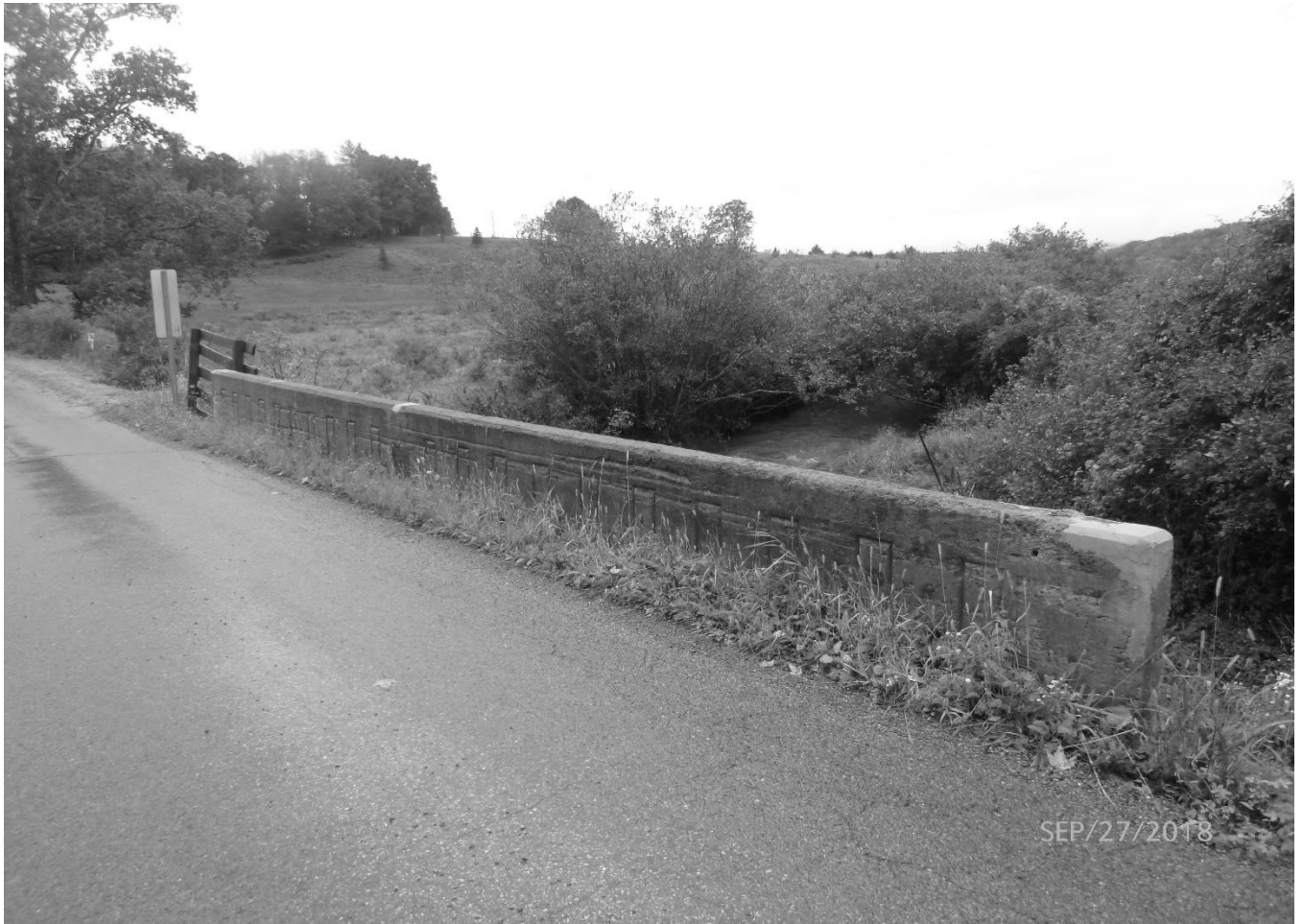
Photo 13 Saulsbury Run Arch Bridge Pocahontas County County Route 4/1 spanning Saulsbury Run West parapet
