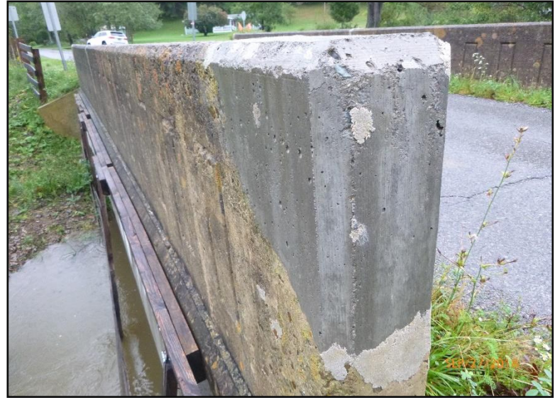
10. Repair to south parapet corner of west abutment. (Photo: WVDOH September 2018)
