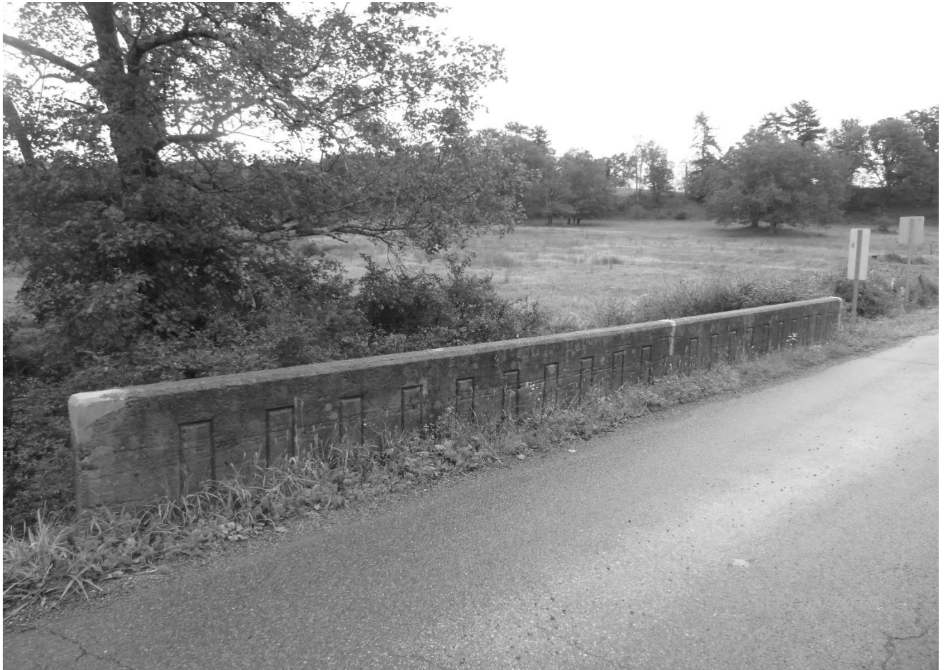
Photo 14 Saulsbury Run Arch Bridge Pocahontas County County Route 4/1 spanning Saulsbury Run East parapet
