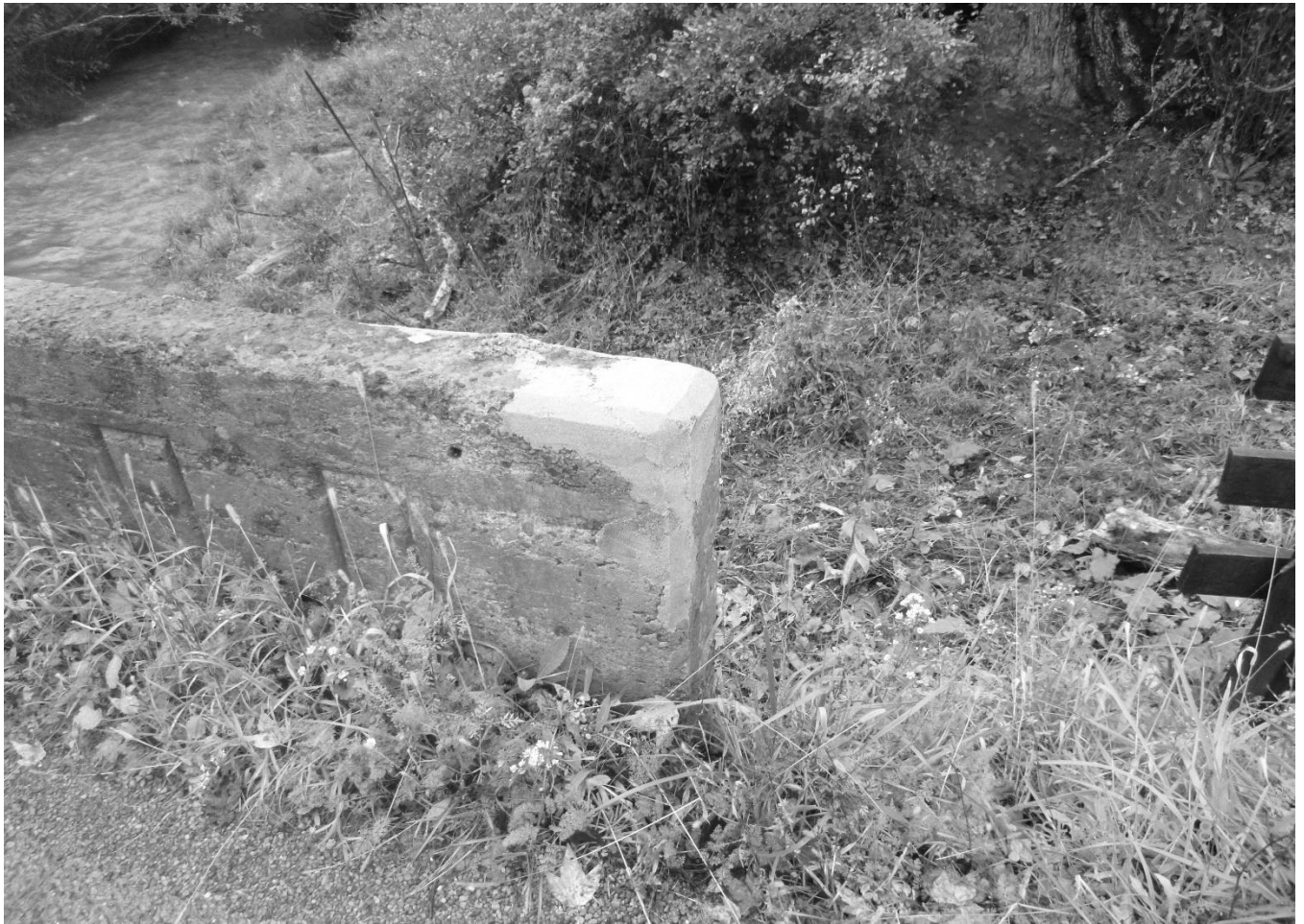
Photo 9 Saulsbury Run Arch Bridge Pocahontas County County Route 4/1 spanning Saulsbury Run Repair to north parapet corner of west abutment
