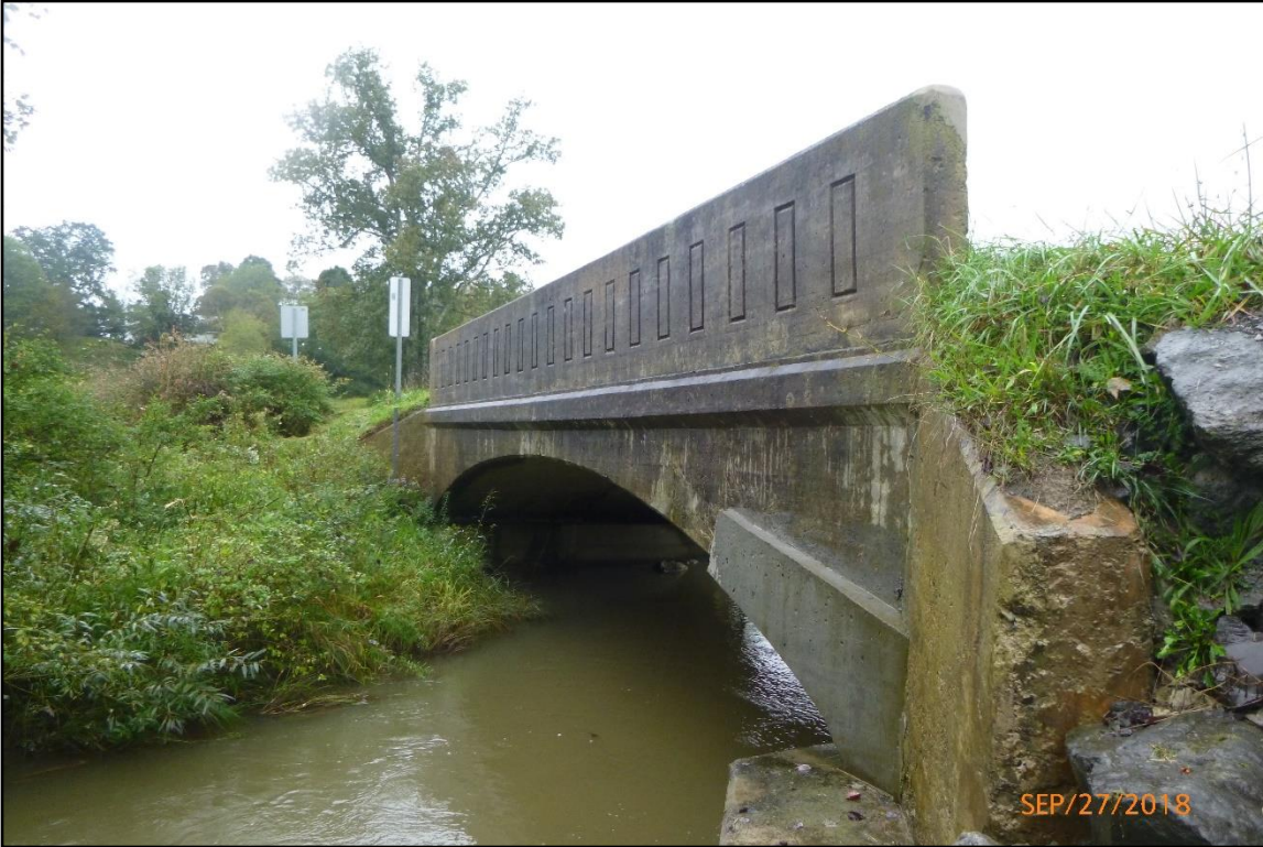
Elevation view, upstream (east) side. (Photo WVDOH, September 2018)
