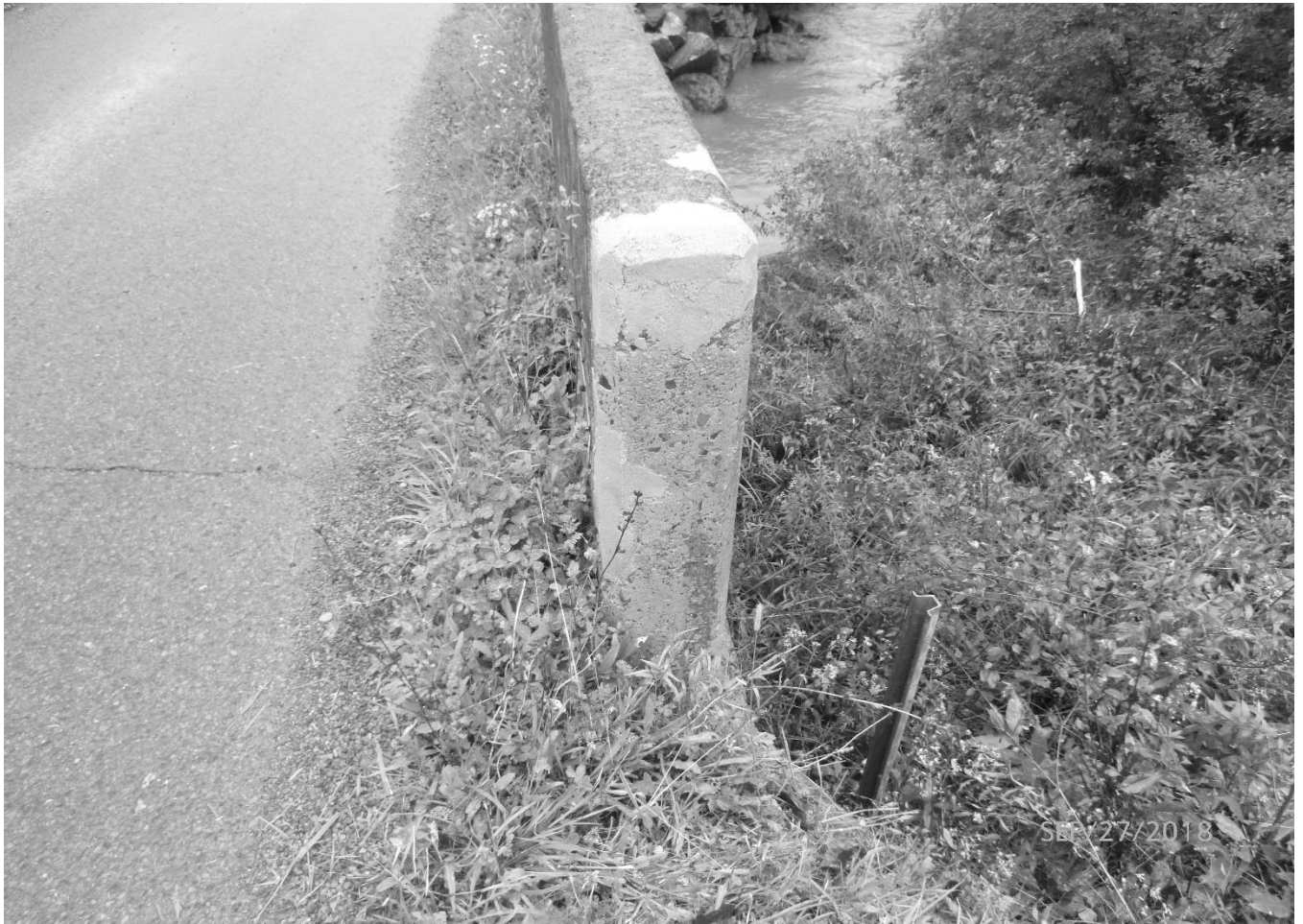
Photo 12 Saulsbury Run Arch Bridge Pocahontas County County Route 4/1 spanning Saulsbury Run Repair to south parapet corner of east abutment
