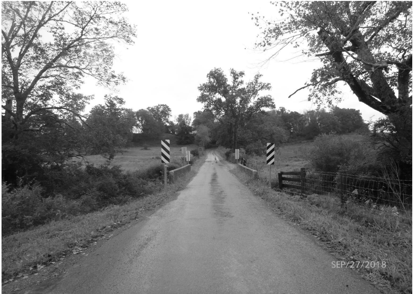
Photo 1 Saulsbury Run Arch Bridge Pocahontas County County Route 4/1 spanning Saulsbury Run North approach to bridge, view south
