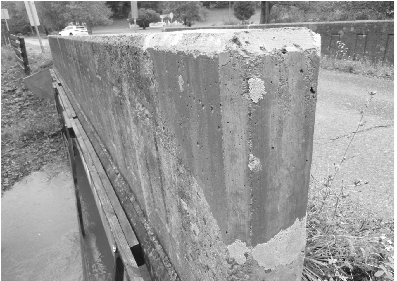
Photo 10 Saulsbury Run Arch Bridge Pocahontas County County Route 4/1 spanning Saulsbury Run Repair to south parapet corner of west abutment
