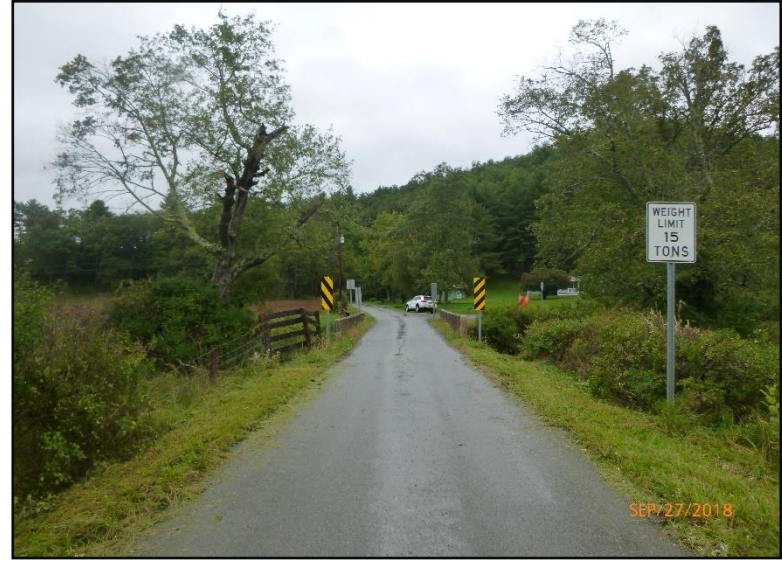
2. South approach to bridge, view north. (Photo: WVDOH September 2018)
