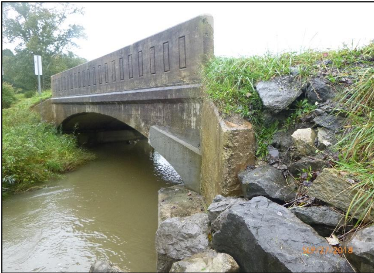
3. Upstream elevation. (Photo: WVDOH September 2018)
