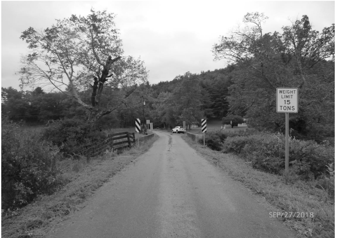
Photo 2 Saulsbury Run Arch Bridge Pocahontas County County Route 4/1 spanning Saulsbury Run South approach to bridge, view north
