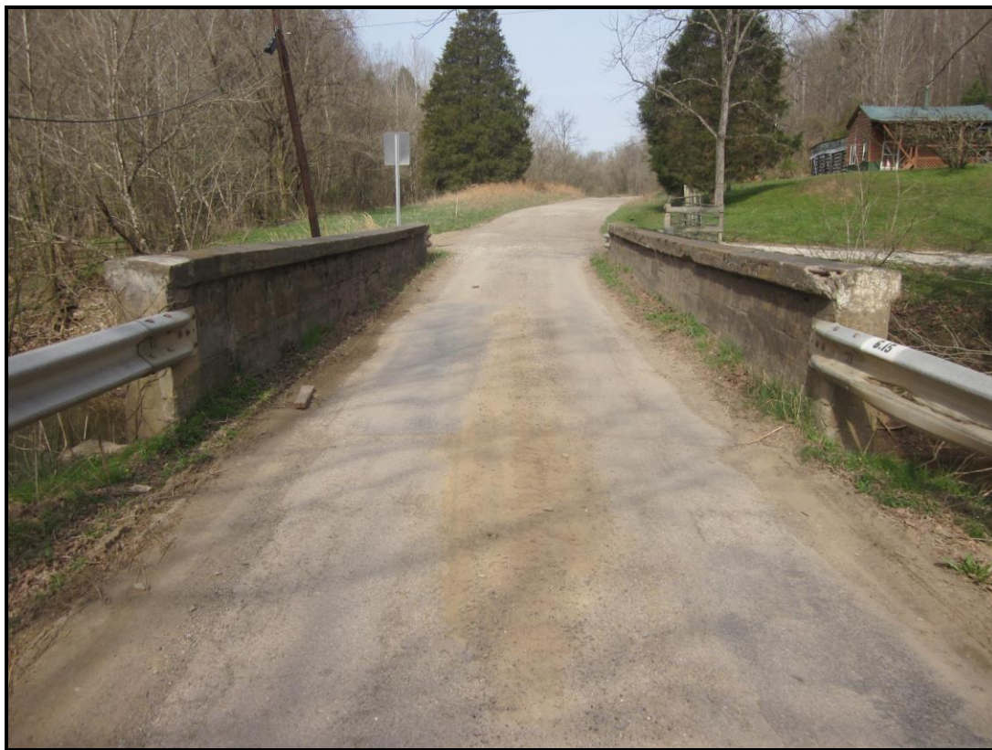
East Approach. View West (WVDOH 4-4-2019)
