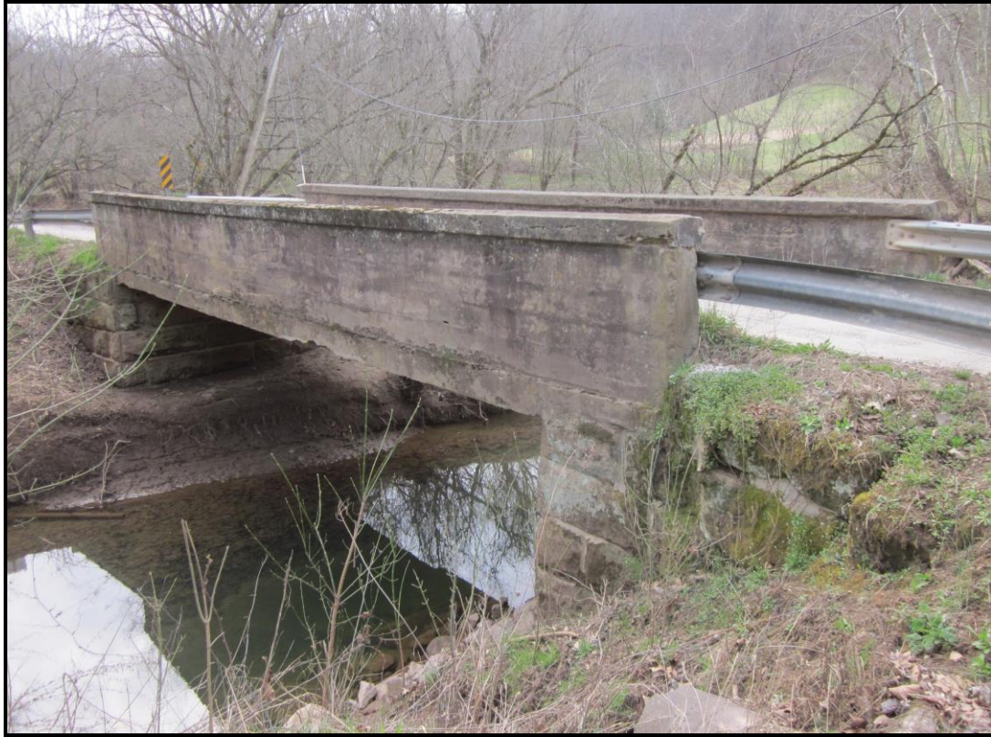
North (Upstream) Elevation. View SE (WVDOH 4-4-2019)
