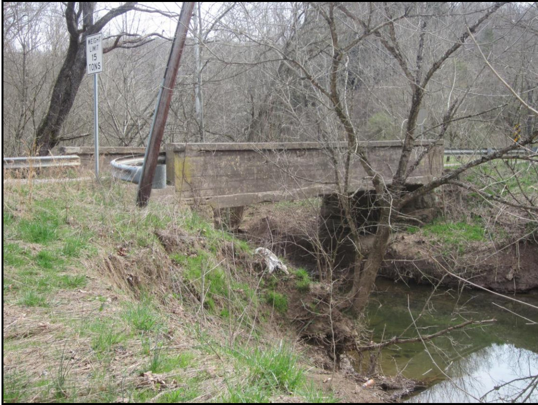
South (Downstream) Elevation. View NE (WVDOH 4-4-2019)
