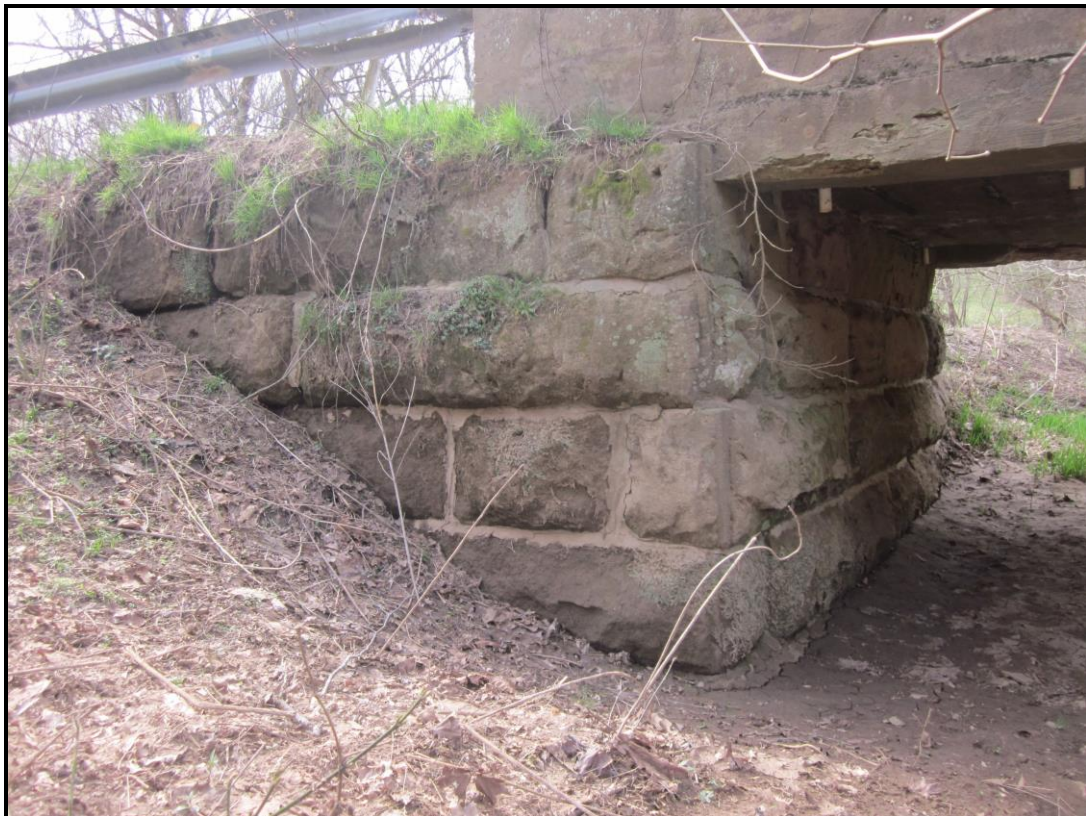
East Abutment. View SE (WVDOH 4-4-2019)
