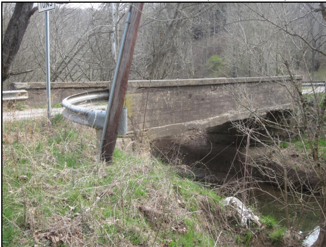
South (Downstream) Elevation. View NE (WVDOH 4-4-2019)
