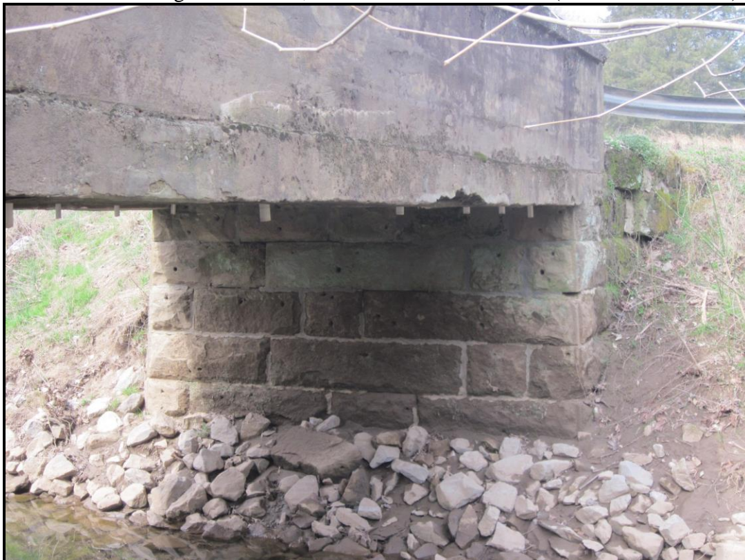
West Abutment. View ESE (WVDOH 4-4-2019)
