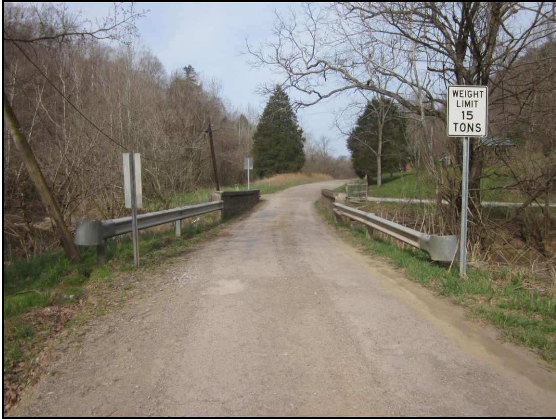
East Approach. View West (WVDOH 4-4-2019)
