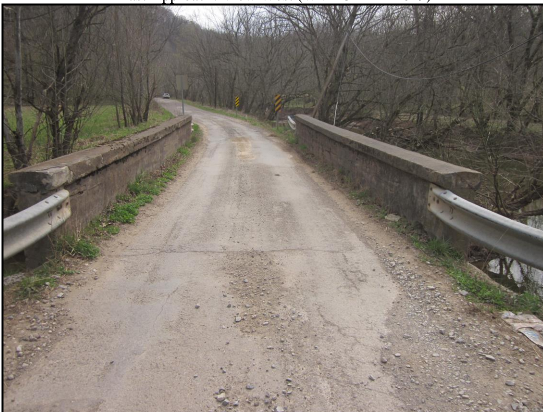
West Approach. View East (WVDOH 4-4-2019)
