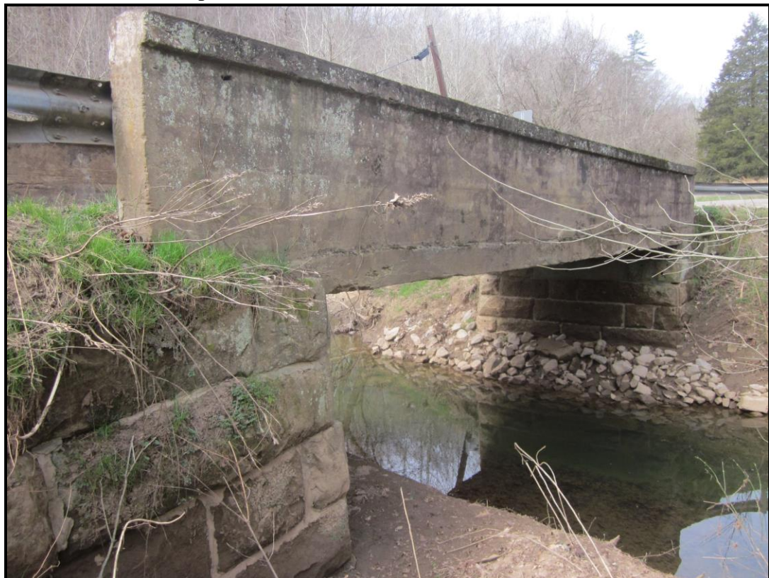
North (Upstream) Elevation. View SW (WVDOH 4-4-2019)
