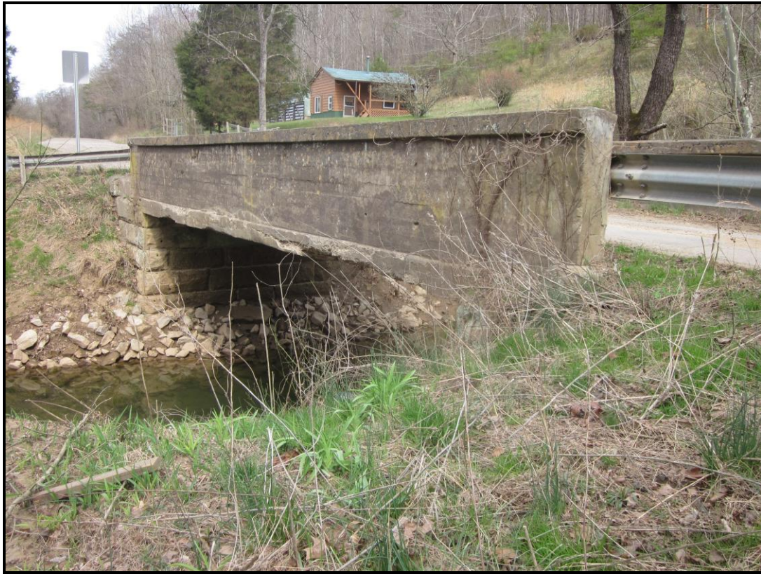
South (Downstream) Elevation. View NW (WVDOH 4-4-2019)
