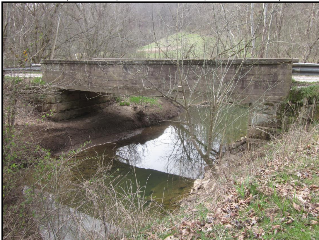
North (Upstream) Elevation. View South (WVDOH 4-4-2019)
