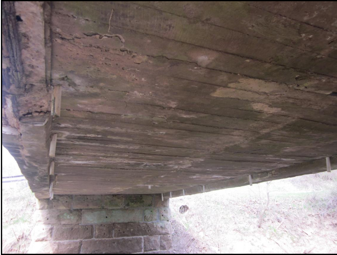
Underside of Bridge. View ENE, taken from East Abutment (WVDOH 4-4-2019)
