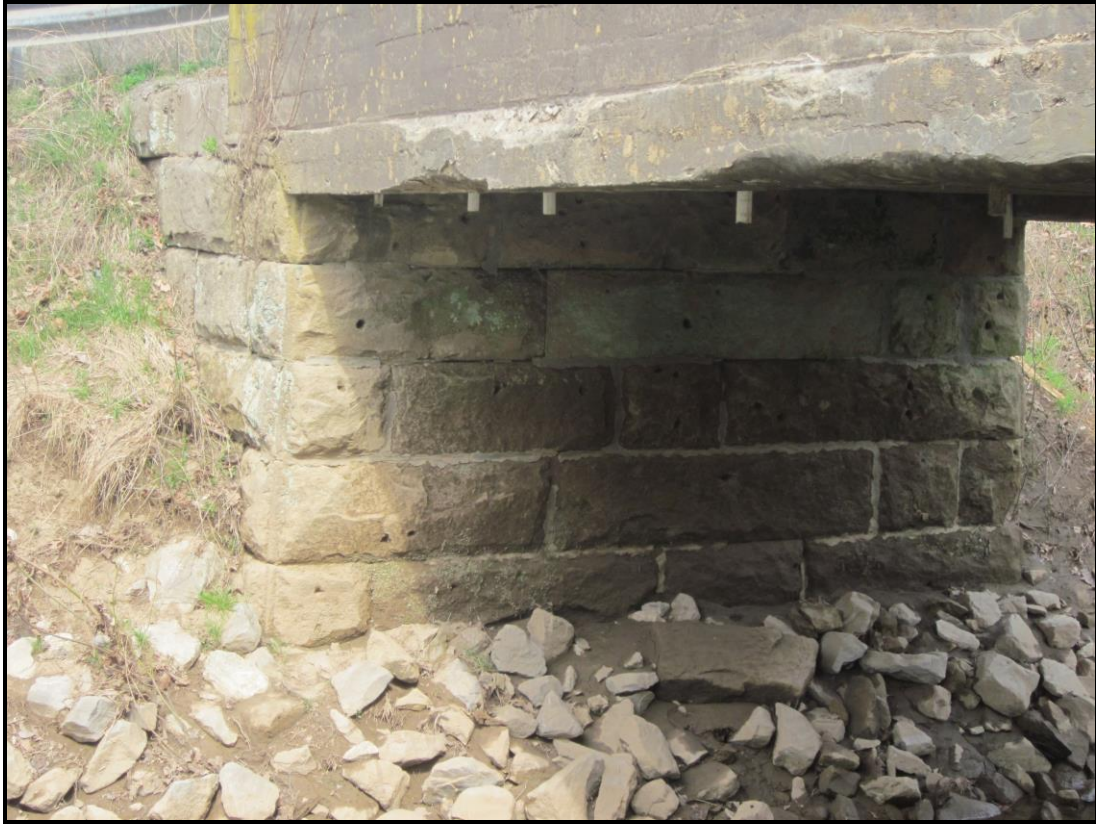
West Abutment. View NW (WVDOH 4-4-2019)
