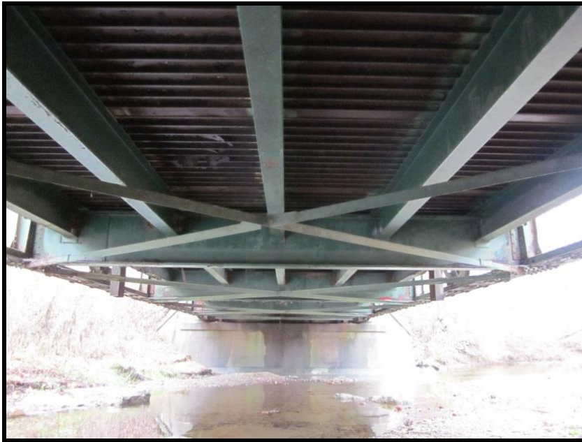
17. Underside of Bridge Decking, highlighting floorbeams, stringers and crossed lateral bracing. View South/Southeast
