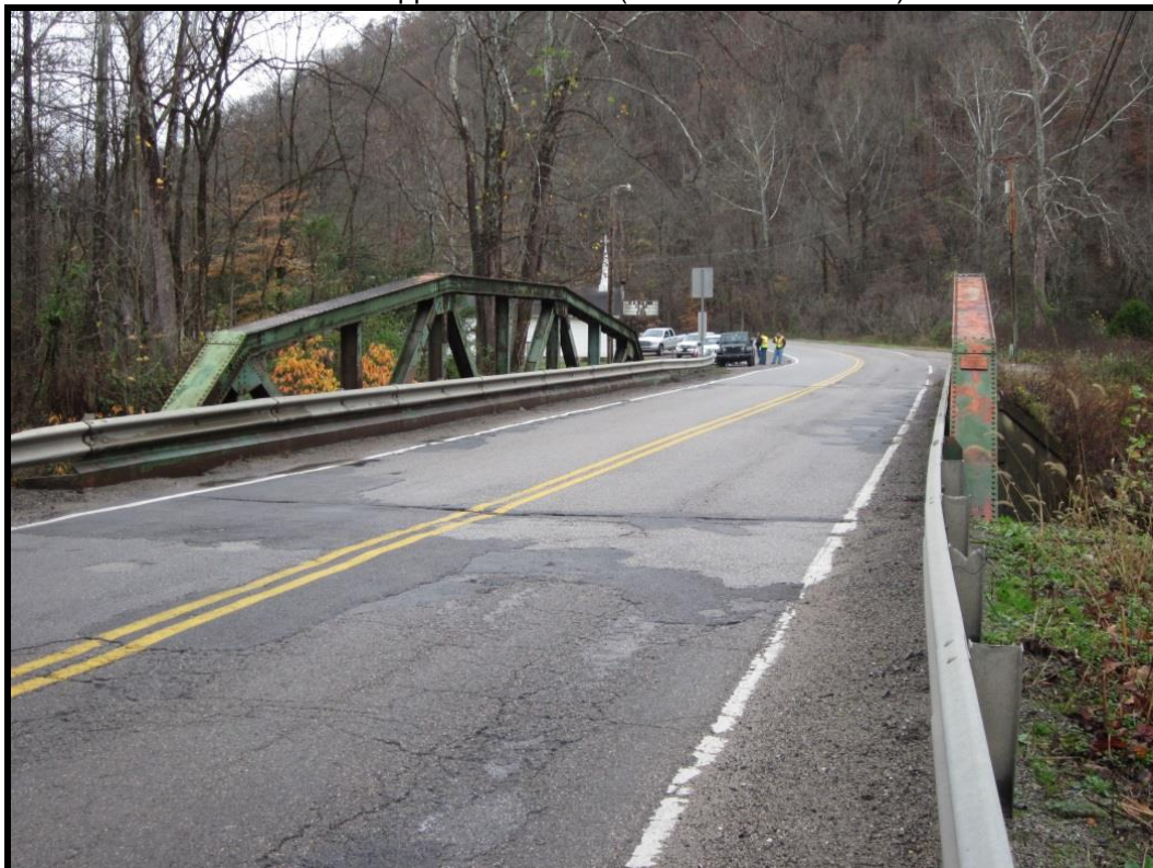
South Approach. View NW (WVDOH 11-10-2015)
