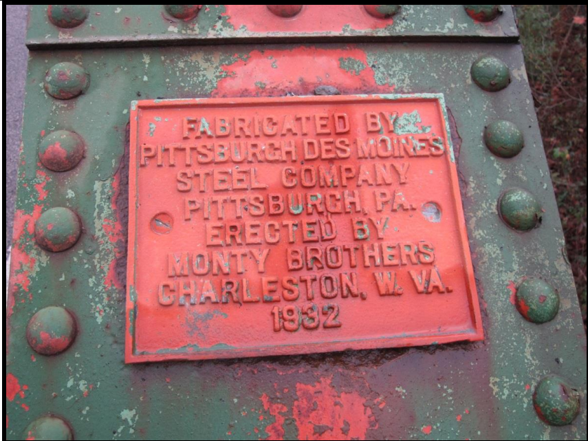
23. Bridge Builders' Plaque at South End Post of East Truss. View North
