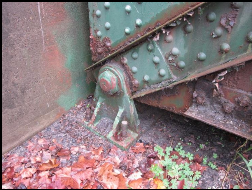
21. Typical Truss Expansion Bearing Connection to Abutment Bridge Seat; View is on North End of West Truss. View Northeast
