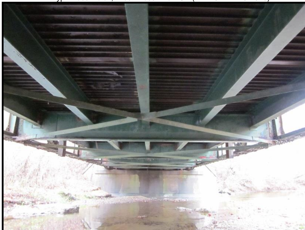
Underside of Bridge Decking, highlighting floorbeams, stringers and crossed lateral bracing. View S/SE (WVDOH 11-10-2015)
