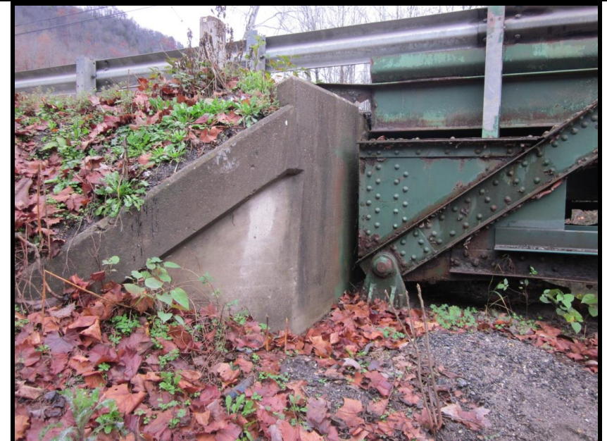
20. Typ. Abutment & Truss/Deck End Connection. View is of North Abutment and West Truss. View East
