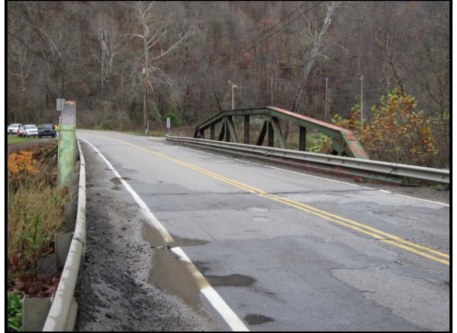
14. South Approach. View Northeast
