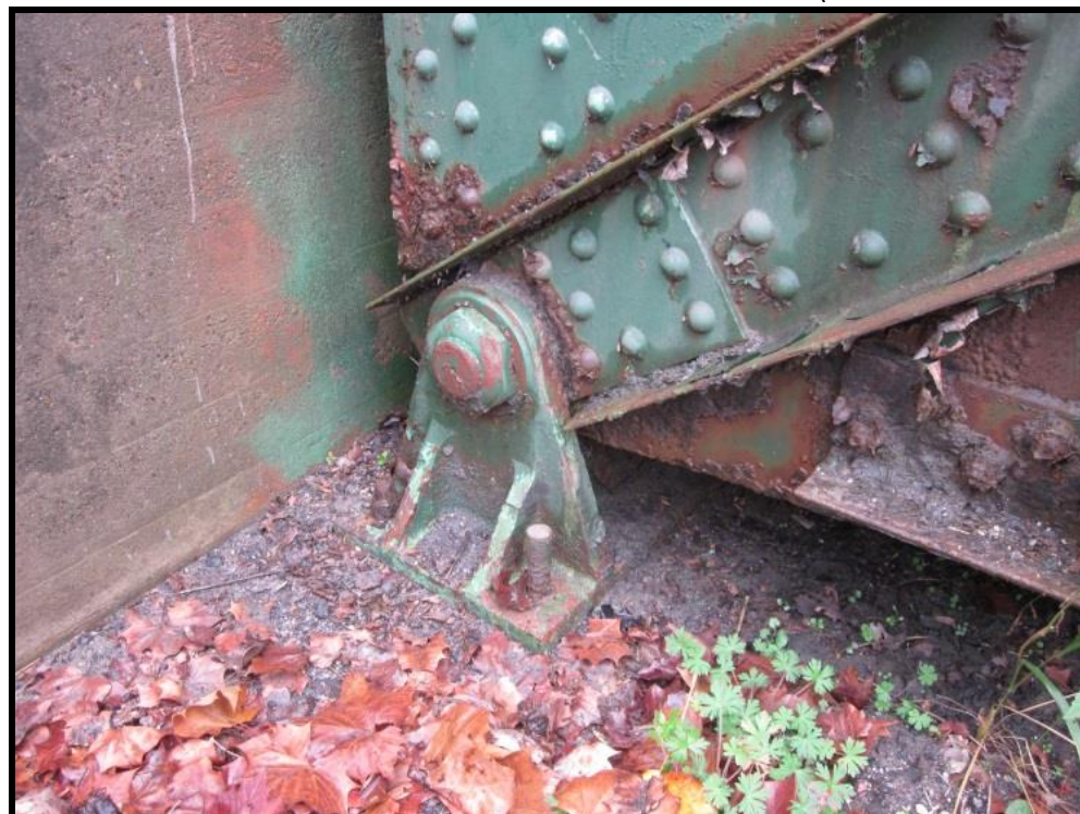
Typical Truss Expansion Bearing connection to Abutment Bridge Seat; view is of north end of West Truss. View NE (WVDOH 11-10-2015)
