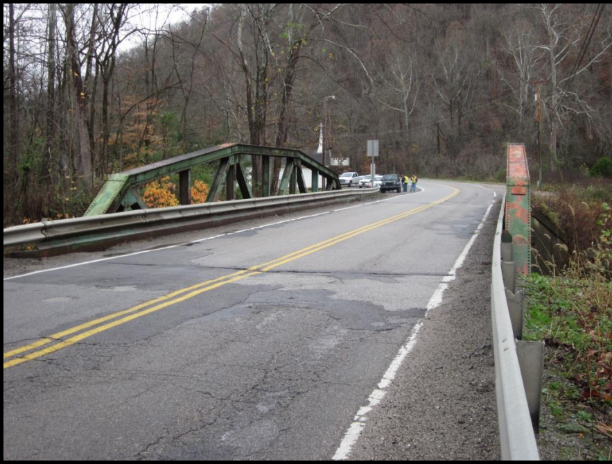
13. South Approach. View Northwest
