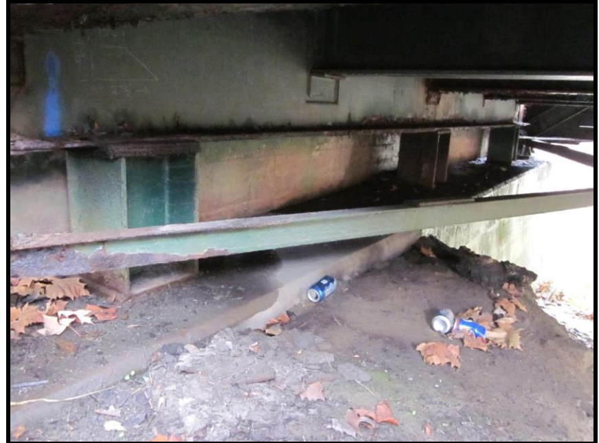
22. Typical End Floorbeam Support Posts at Bridge Seat; View is of North Abutment. View Northeast
