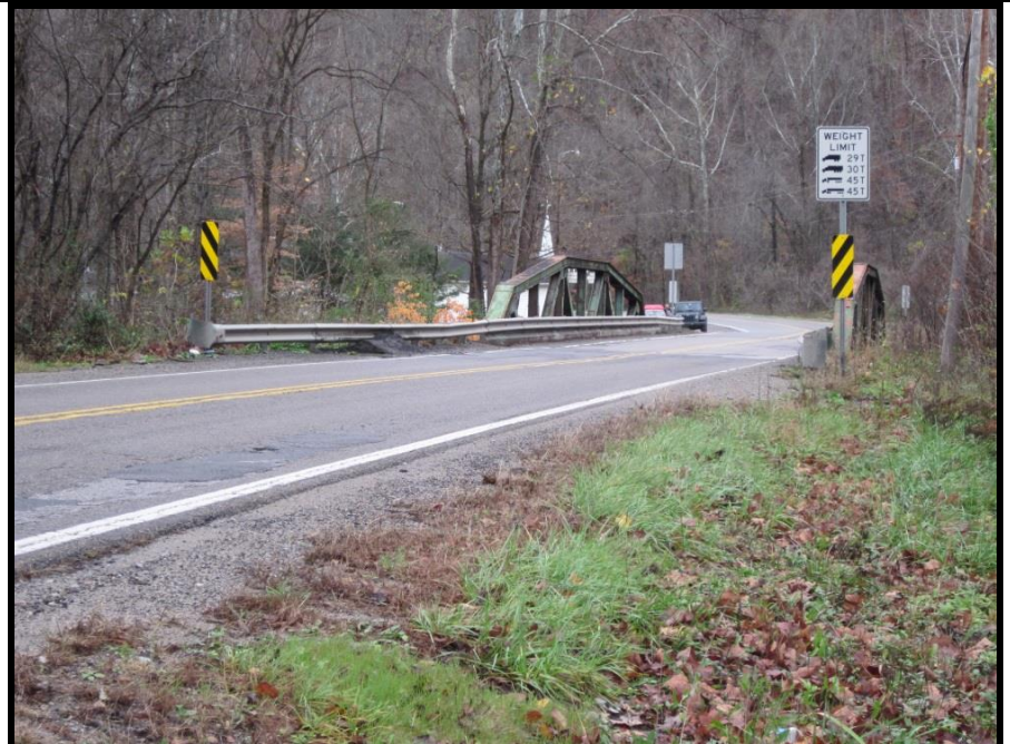
12. South Approach. View Northwest
