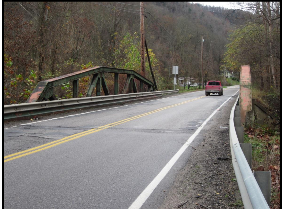
8. North Approach. View Southeast
