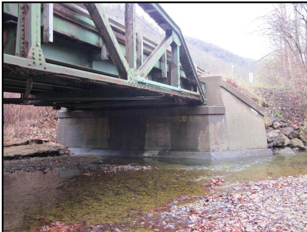
South Abutment. View SE (WVDOH 11-10-2015)
