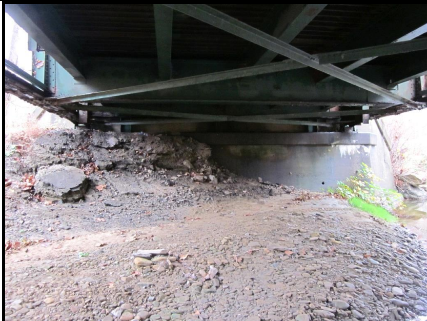
19. North Abutment. View North/Northwest
