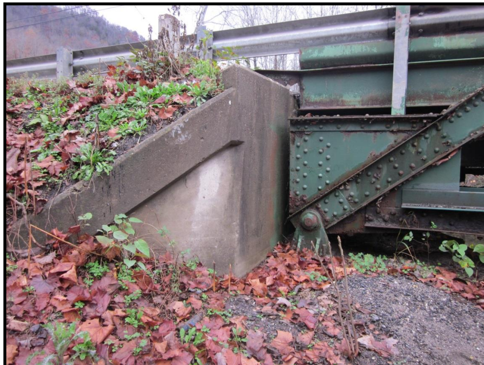
Typ. Abutment & Truss/Deck End Connection. View is of the North Abutment and West Side Truss. View E (WVDOH 11-10-2015)
