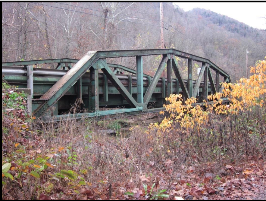
3. West (Downstream) Elevation. View Southeast
