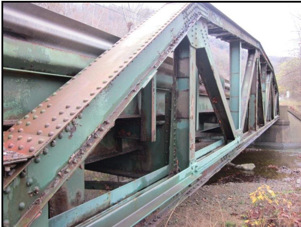
Typ. Truss Detail; West Truss. View SE (WVDOH 11-10-2015)
