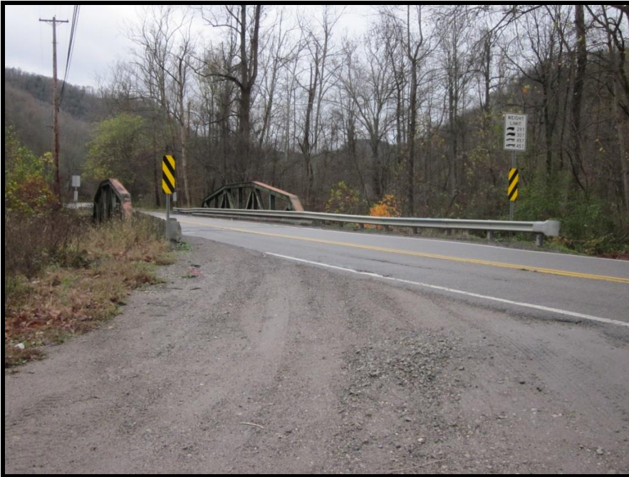
9. North Approach. View Southwest
