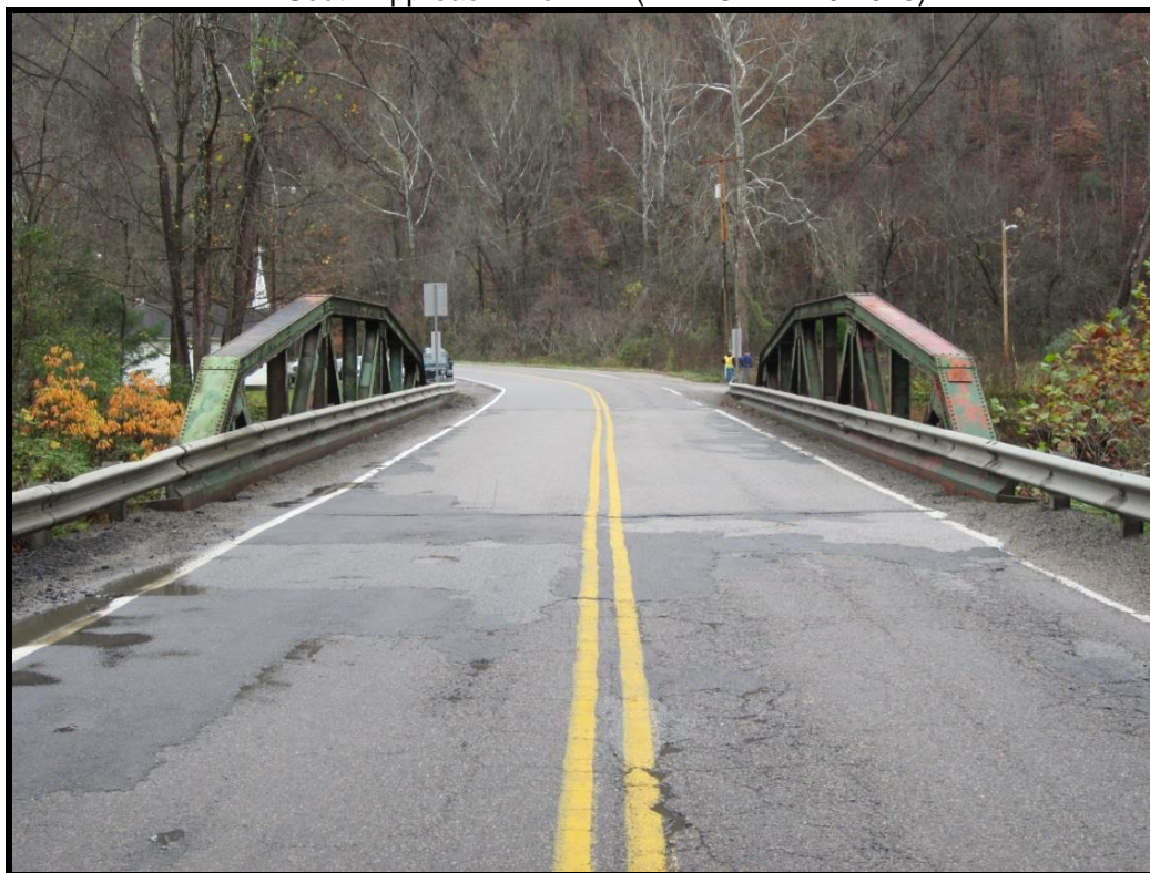
South Approach. View N (WVDOH 11-10-2015)
