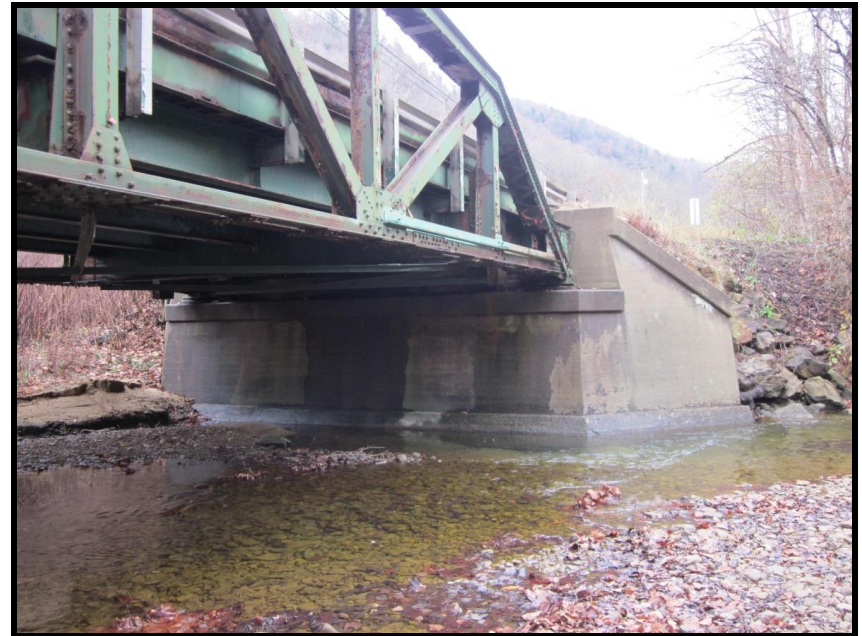
18. South Abutment. View Southeast
