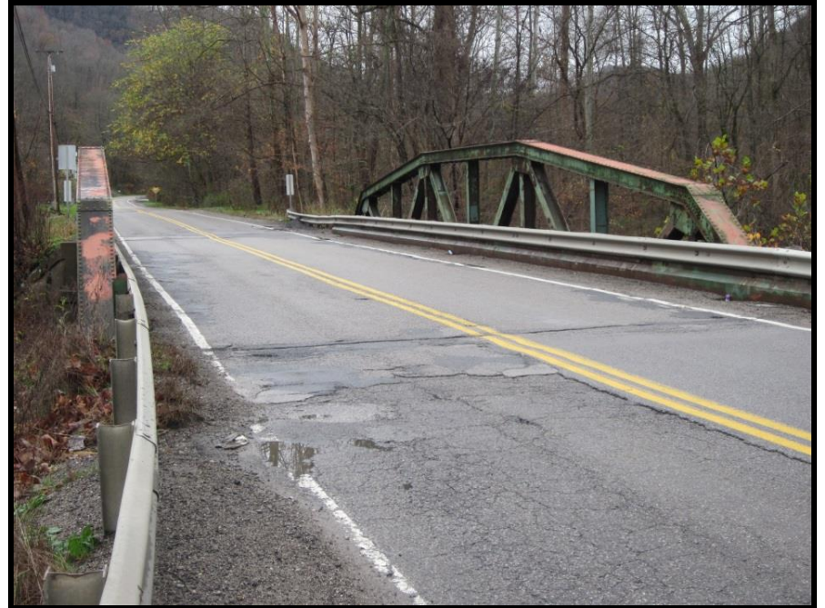
10. North Approach. View Southwest
