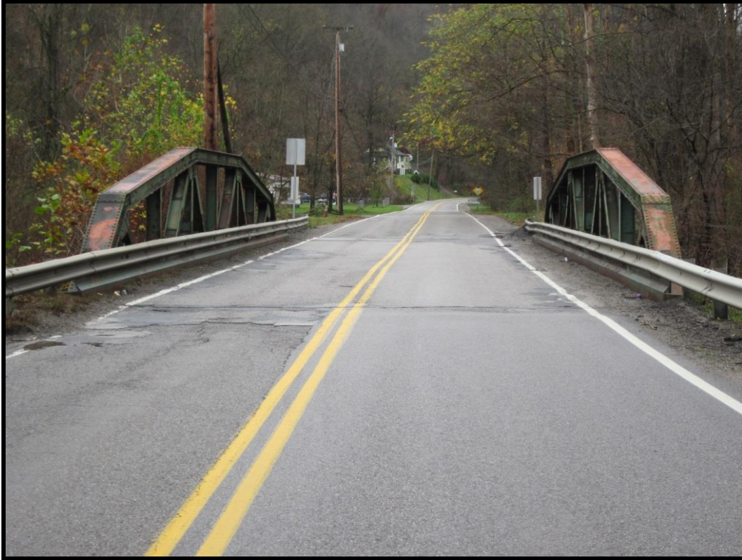
North Approach. View S (WVDOH 11-10-2015)
