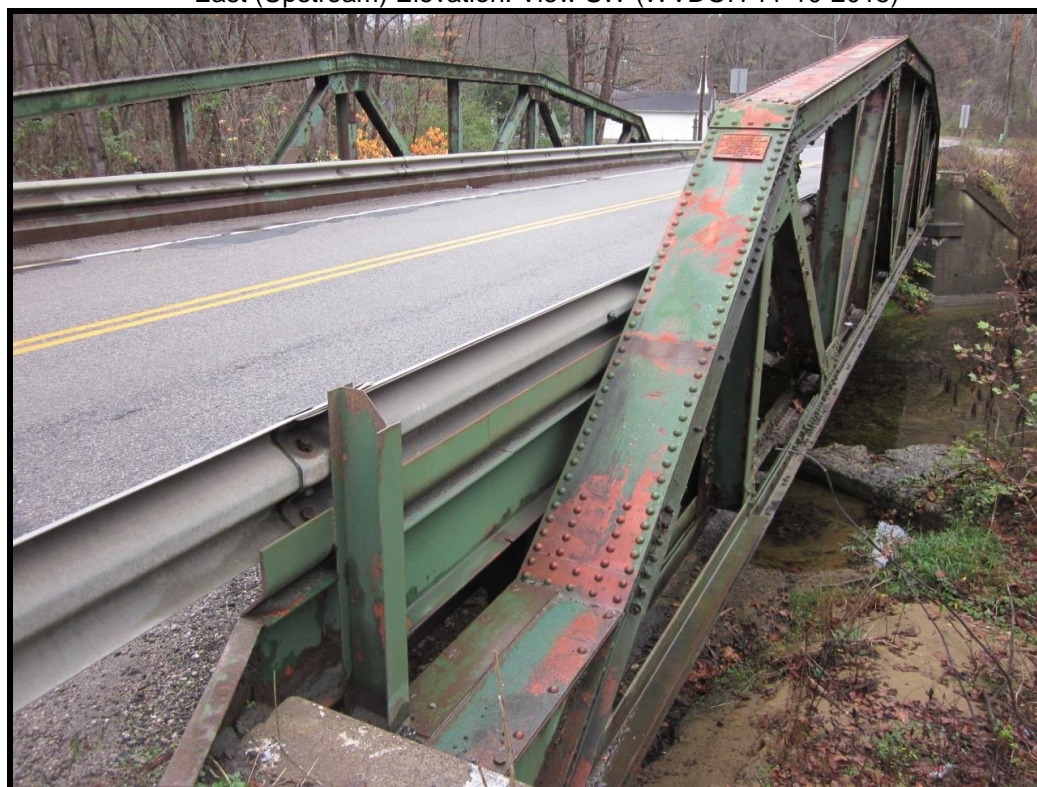
East Truss with Builder's Plaque. View NW (WVDOH 11-10-2015)
