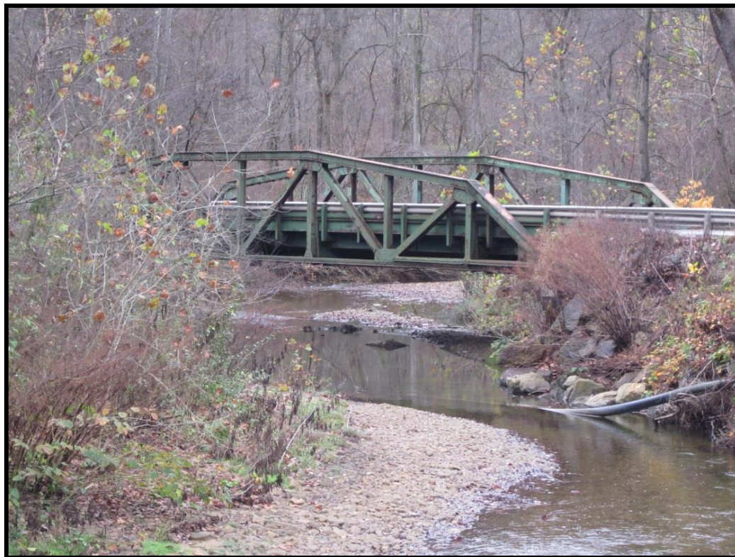
East (Upstream) Elevation. View SW (WVDOH 11-10-2015)
