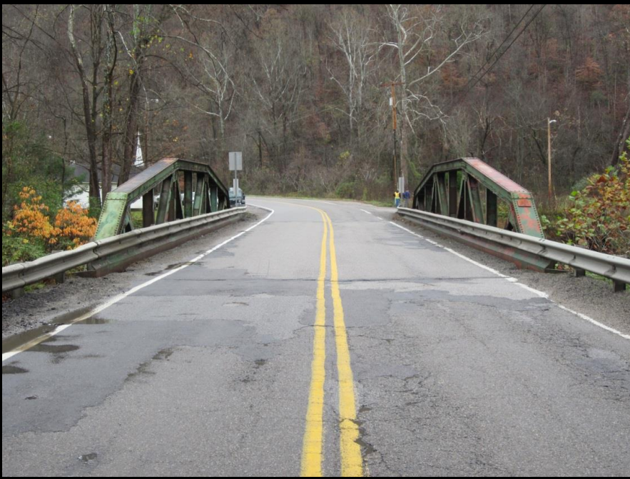
15. South Approach. View North
