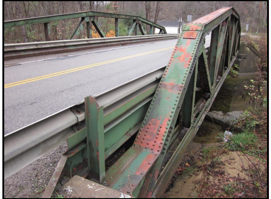
6. East Truss with Builders' Plaque. View Northwest
