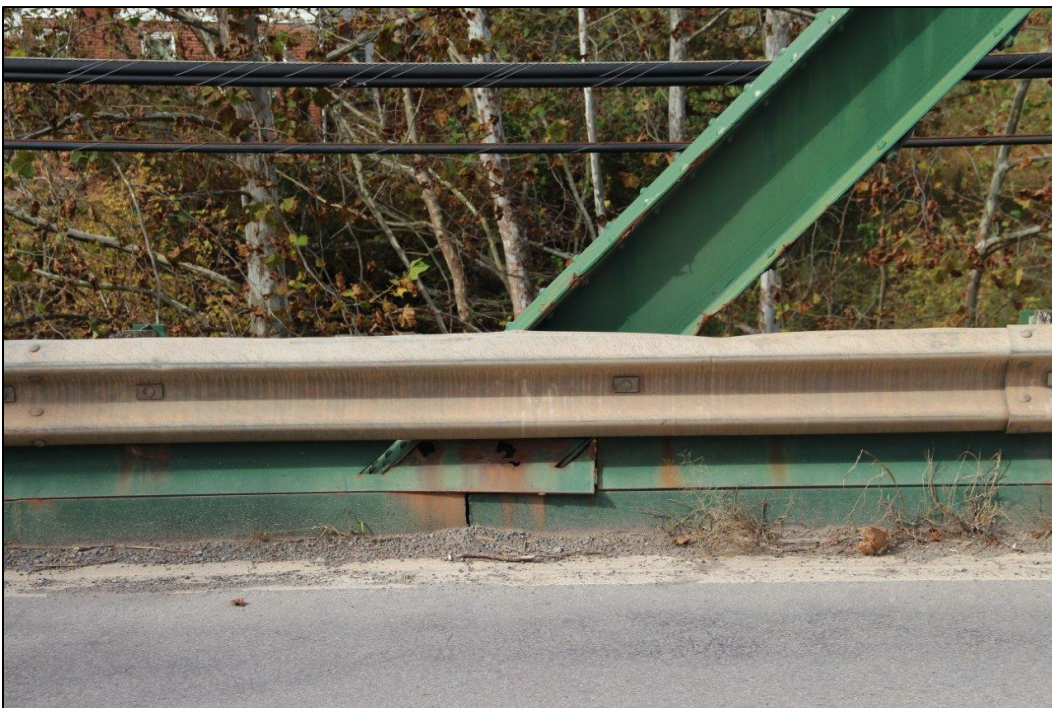
Photo 20. DETAIL OF GUARDRAIL AND SPLASHGUARD, FACING NORTHWEST (WV_Gilmer County_Glenville Truss Bridge_0020).
