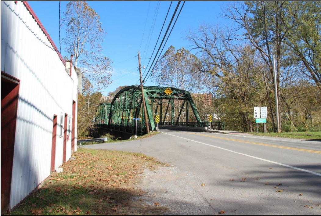
Photo 1. BRIDGE IN CONTEXT SHOWING SOUTHWEST APPROACH OF BRIDGE, FACING NORTHEAST (WV_Gilmer County_Glenville Truss Bridge_0001).
