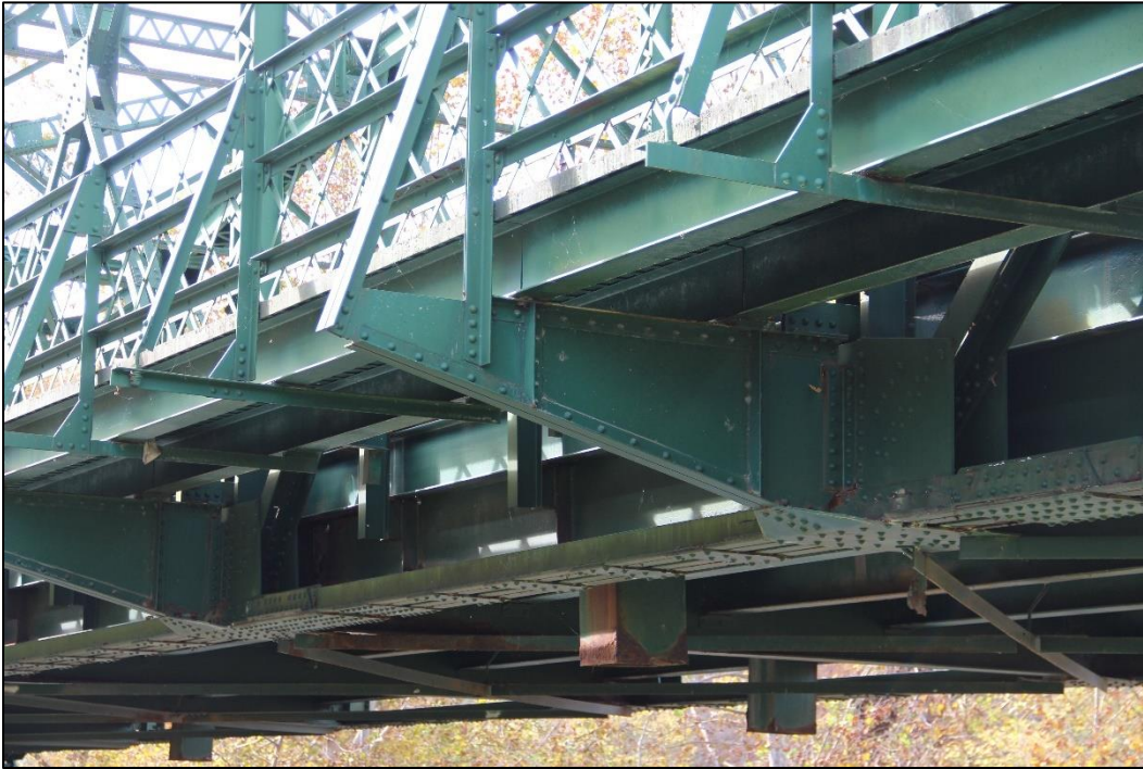
Photo 29. DETAIL OF SIDEWALK BRACKETS AND BEAMS, SOUTHEAST ELEVATION OF SPAN 2 (NORTHEAST), FACING WEST (WV_Gilmer County_Glenville Truss Bridge_0029).
