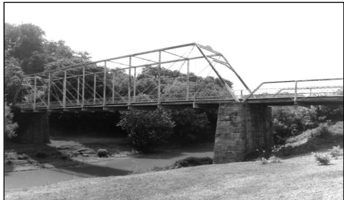
Figure 1. Undated photo of the 1885 Glenville Bridge. (Gilmer County Historical Society.)
