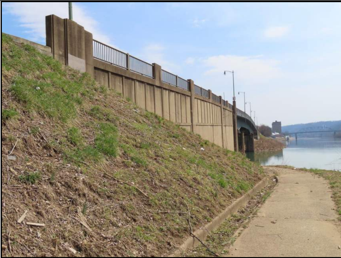
Return-type Wingwall at West Abutment, south/downstream side. View SE (WVDOH 3-13-2025)
