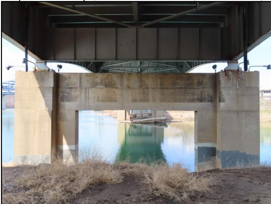
Substructure – Typ. Pier. View is of East Pier. View NW (WVDOH 3-13-2025)
