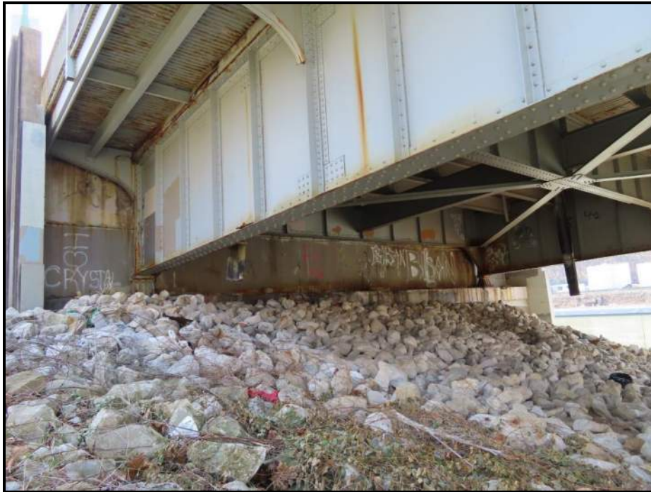
East Abutment. View SE (WVDOH 3-13-2025)
