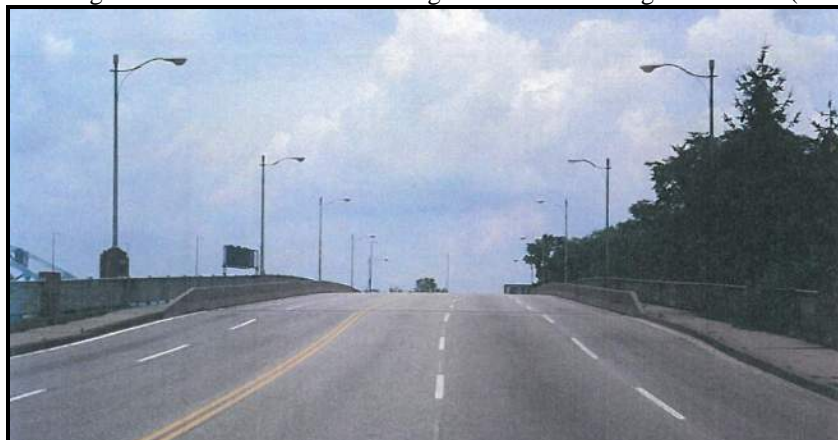
1994 Image of Bridge. Lampposts include light fixtures (luminaire, arms/braces) estimated to have been installed ca. 1980. These fixtures were replaced with the current lamps/arms ca. 2008-10. (Image from 1994 WVDOH bridge inspection report)
