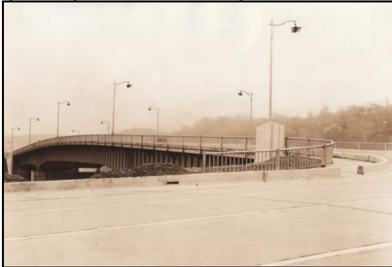
View of North/Upstream side of Bridge, ca. 1939. Taken from West End of Bridge, on former Columbia Blvd, now the entrance to the Union Square Office complex. Image depicts the original light fixtures on the bridge.
