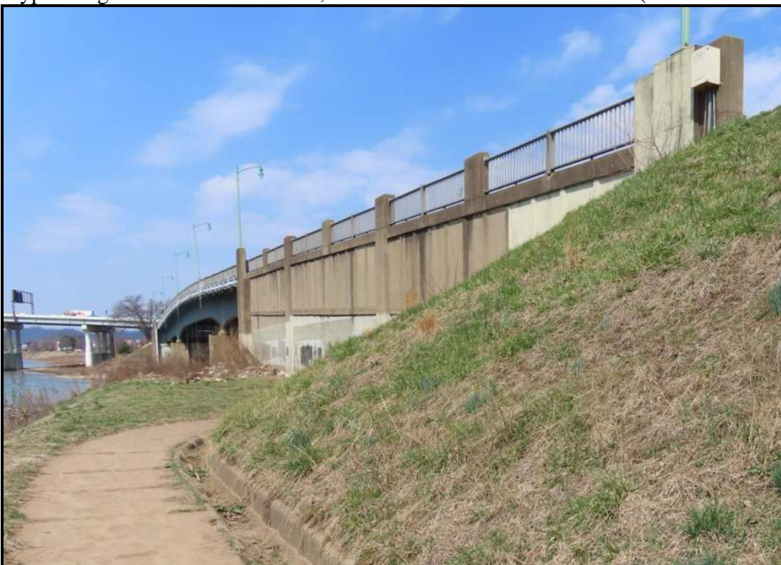
Return-type Wingwall at East Abutment, south/downstream side. View NW (WVDOH 3-13-2025)
