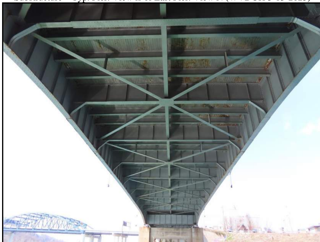
Superstructure – Main/Center Span, Underside of Deck. View NW (WVDOH 3-13-2025)
