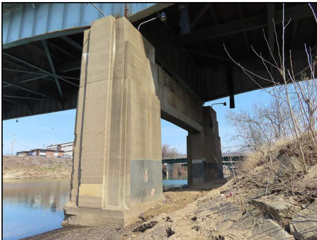
Substructure – Typ. Pier. View is of East Pier. View N (WVDOH 3-13-2025)
