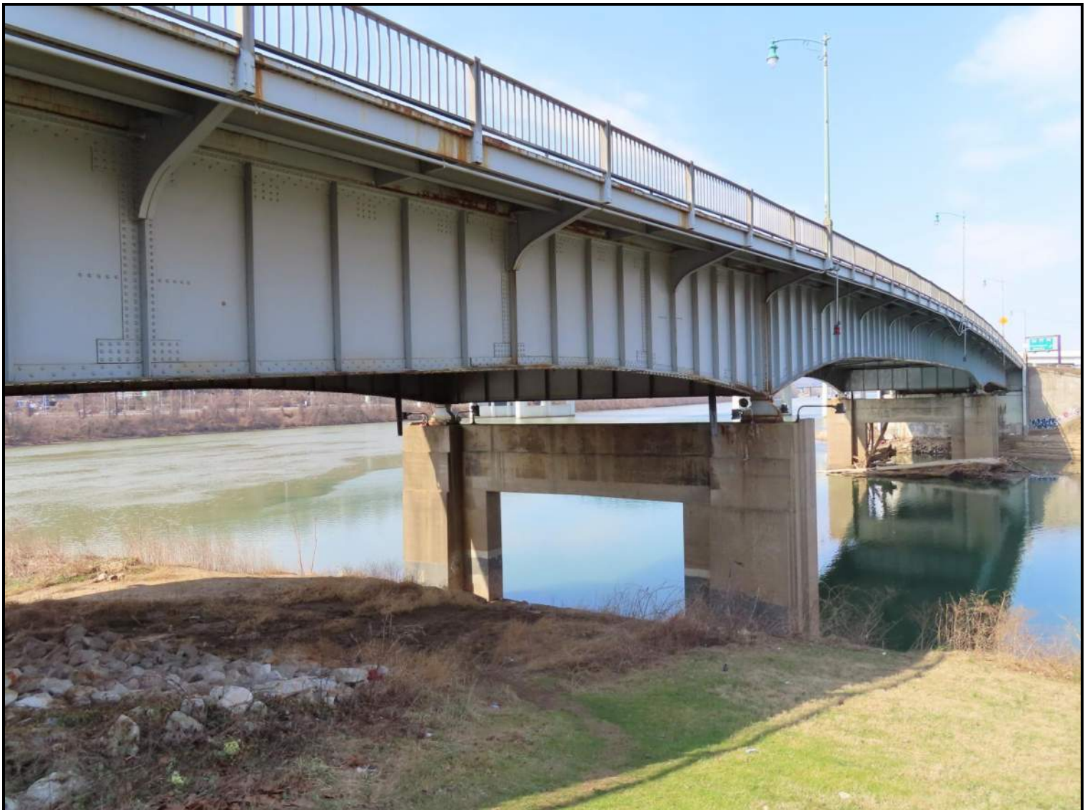
North/Upstream Elevation. View WNW, taken from Courtyard Hotel property (WVDOH 3-13-2025).
