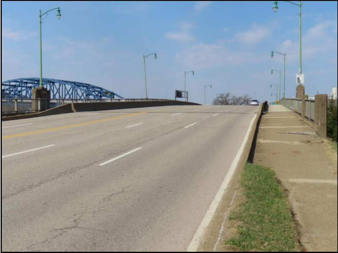
East Approach, taken from north/upstream side. View NW (WVDOH 3-13-2025)
