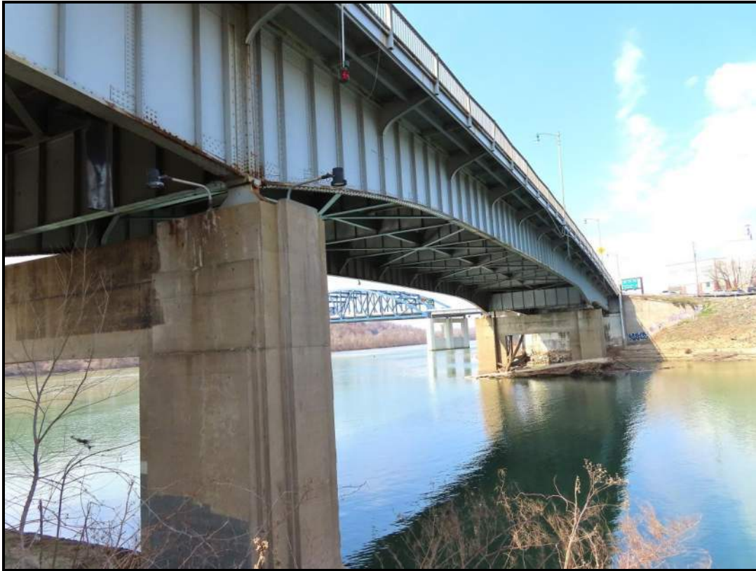
North/Upstream Elevation & Underside of Main Span. View NW. (WVDOH 3-13-2025)
