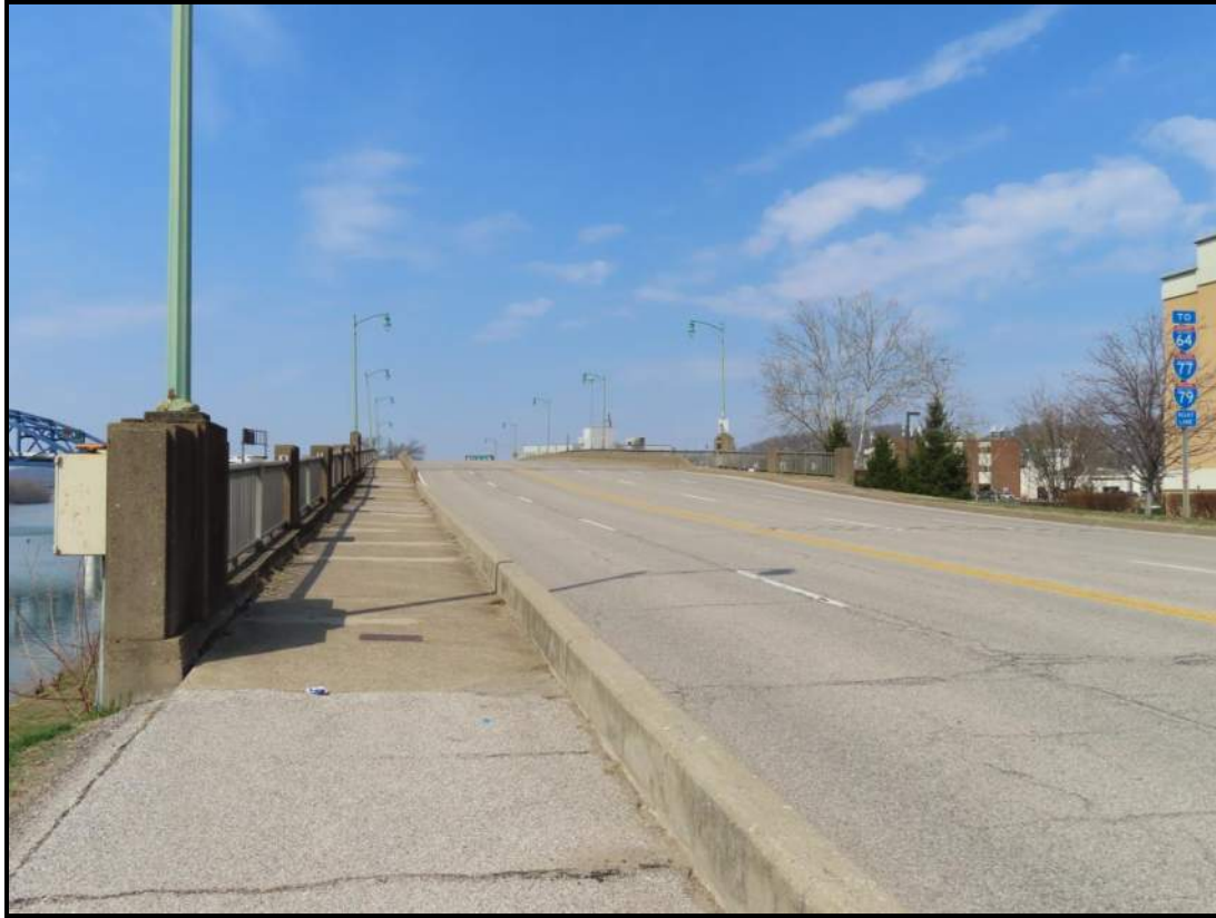
East Approach. View NW, taken from south/downstream side (WVDOH 3-13-2025)
