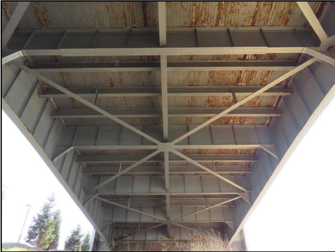
Superstructure - East Span, Underside of Deck. View SE (WVDOH 3-13-2025)
