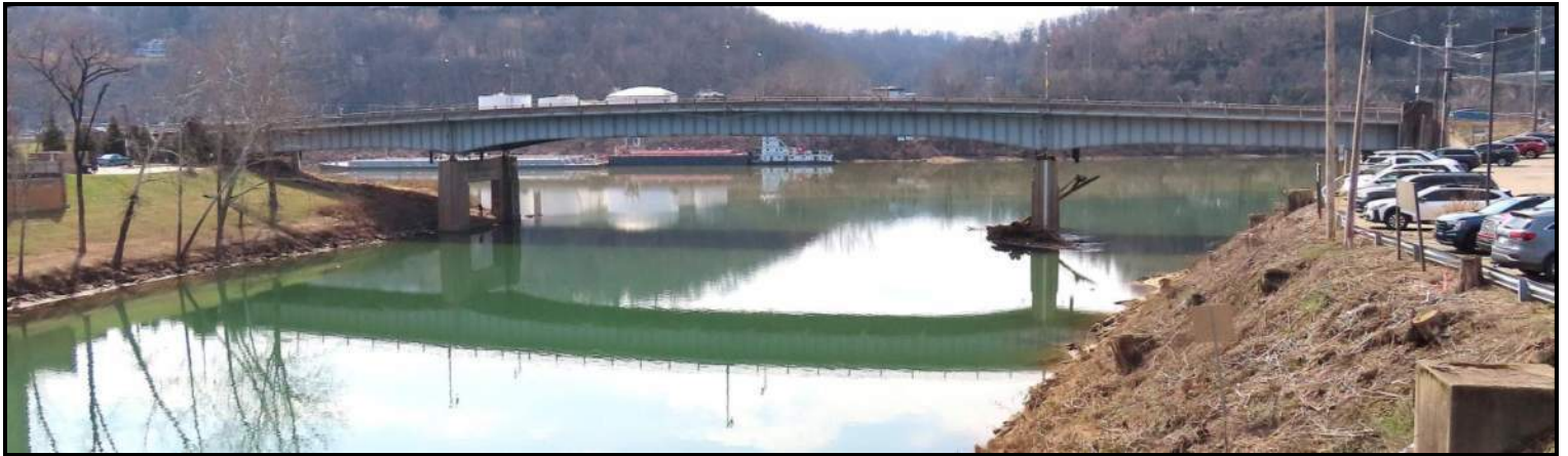
Kanawha Blvd Bridge – North/Upstream Elevation. View SW, taken from west end of Virginia St Bridge (WVDOH 3-13-2025).
