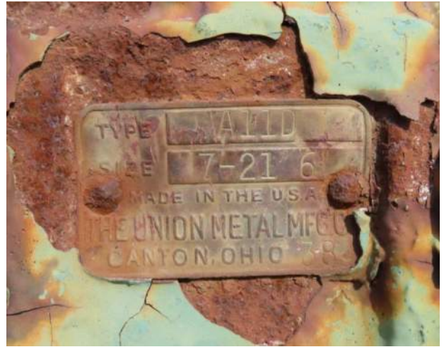
Manufacturer's tag at Base of Lamppost (Fluted Pole) on Bridge (WVDOH 3-13-2025)
