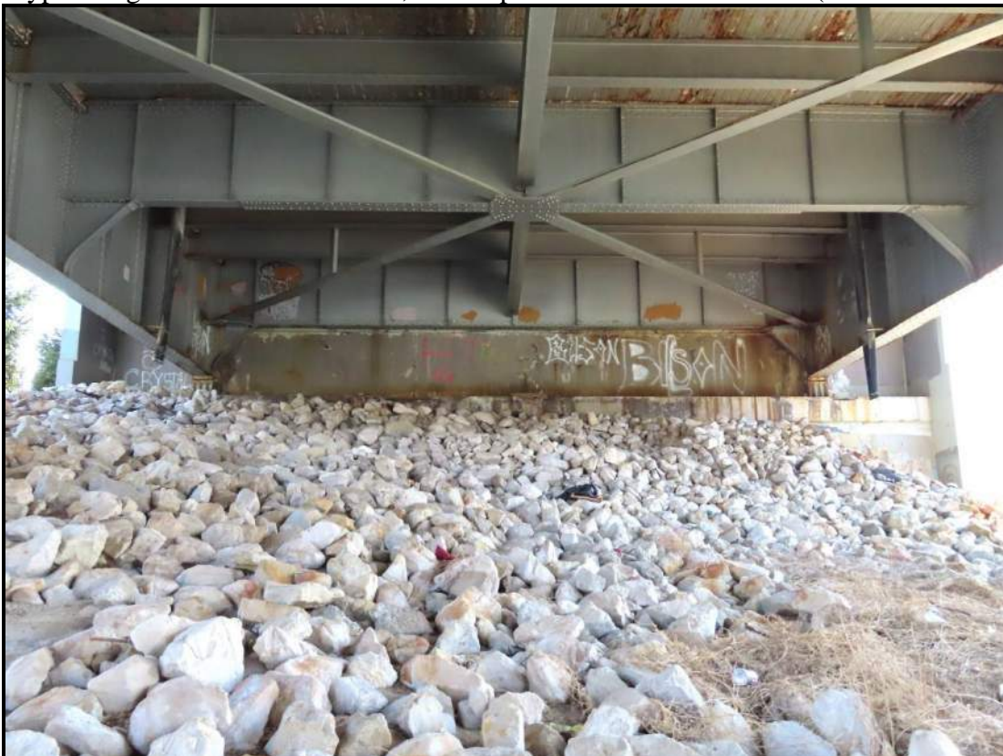
East Abutment. View SE (WVDOH 3-13-2025)
