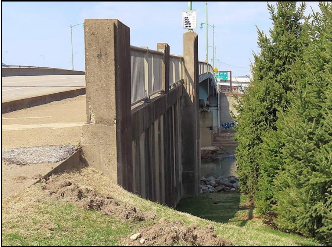
Return-type Wingwall at East Abutment, north/upstream side. View WNW (WVDOH 3-13-2025).
