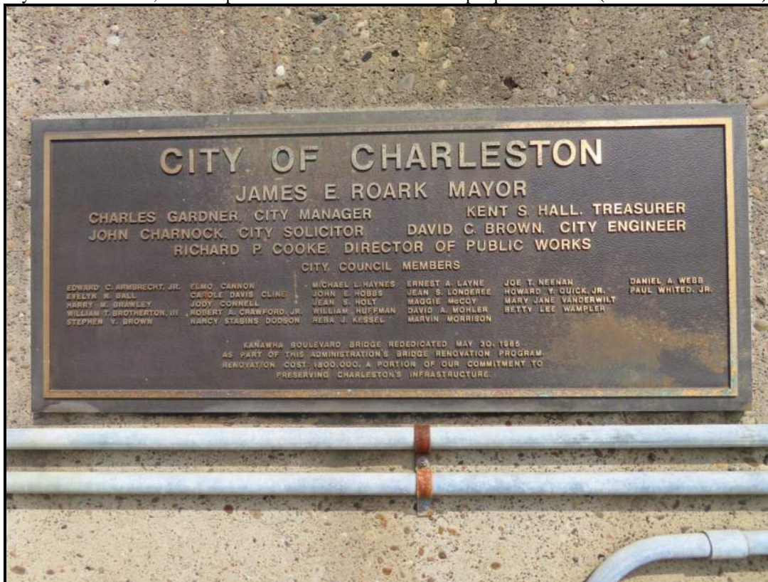
Plaque on both West End Pylons (WVDOH 3-13-2025)
