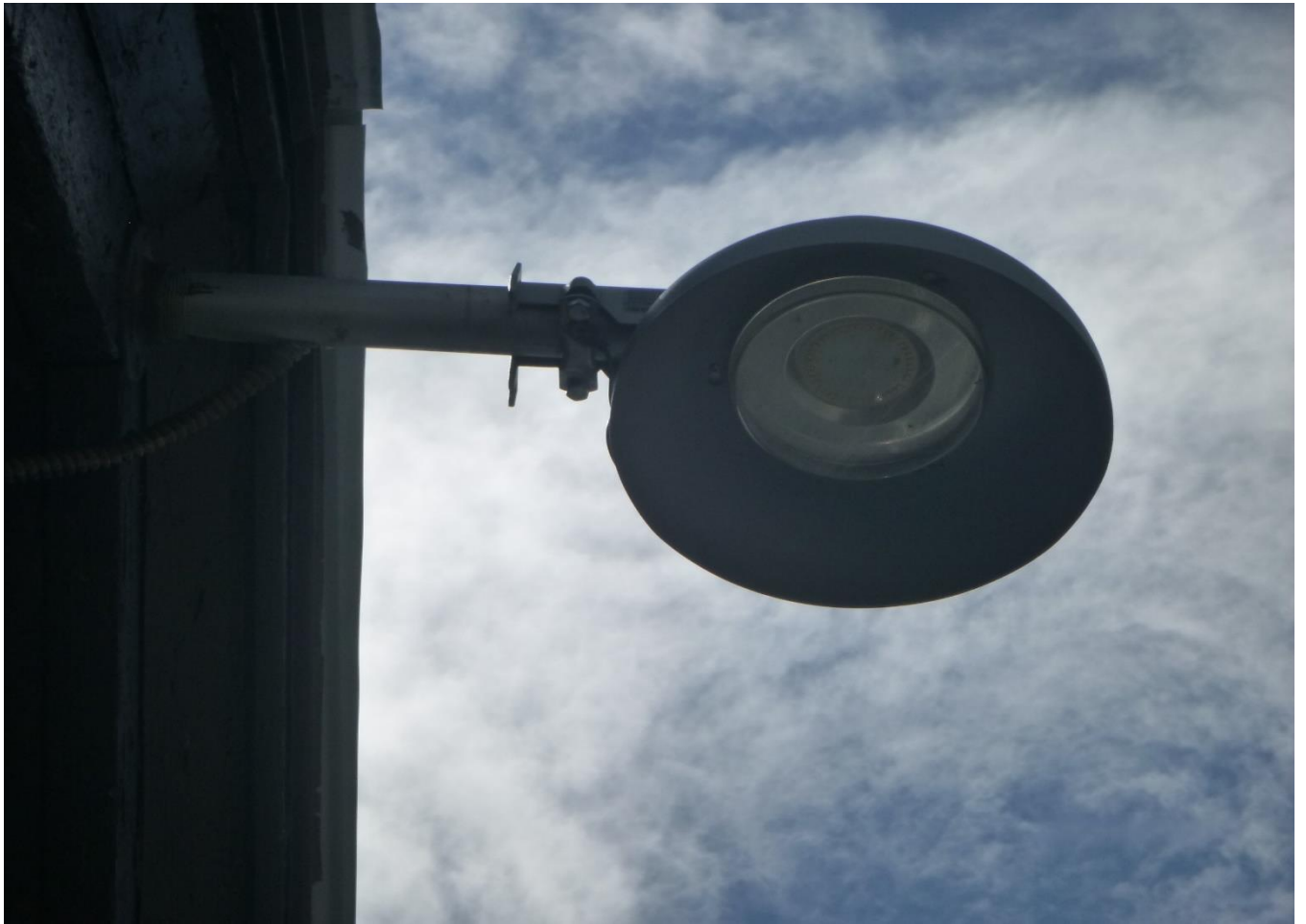
Photo 10 Barbour County Maintenance HQ Shed Barbour County State Route 119 Detail of lighting attached to west elevation
