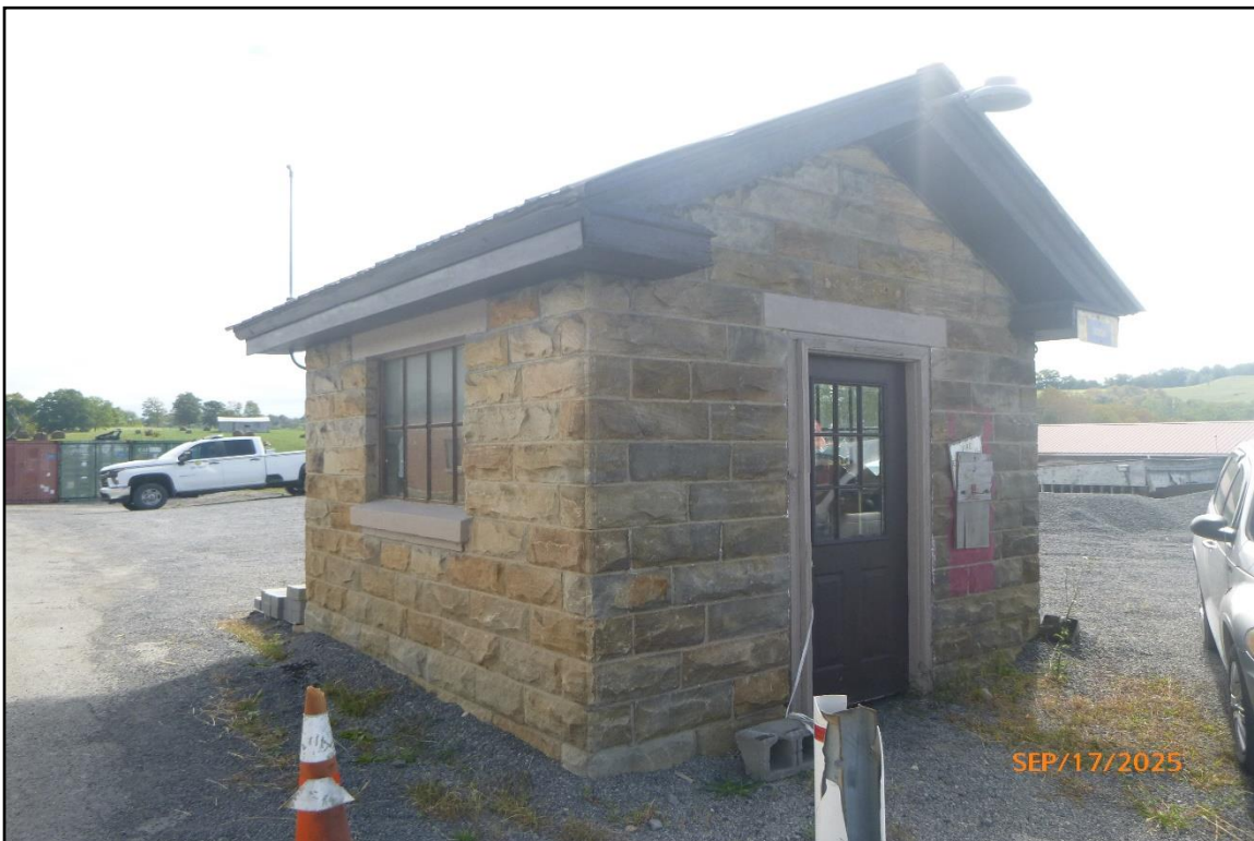
Former gas house located south of garage building, west (façade) and north elevation.
