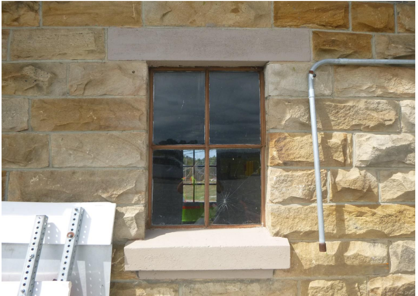
Photo 8 Barbour County Maintenance HQ Shed Barbour County State Route 119 Detail of steel window and concrete sill and lintel on east elevation
