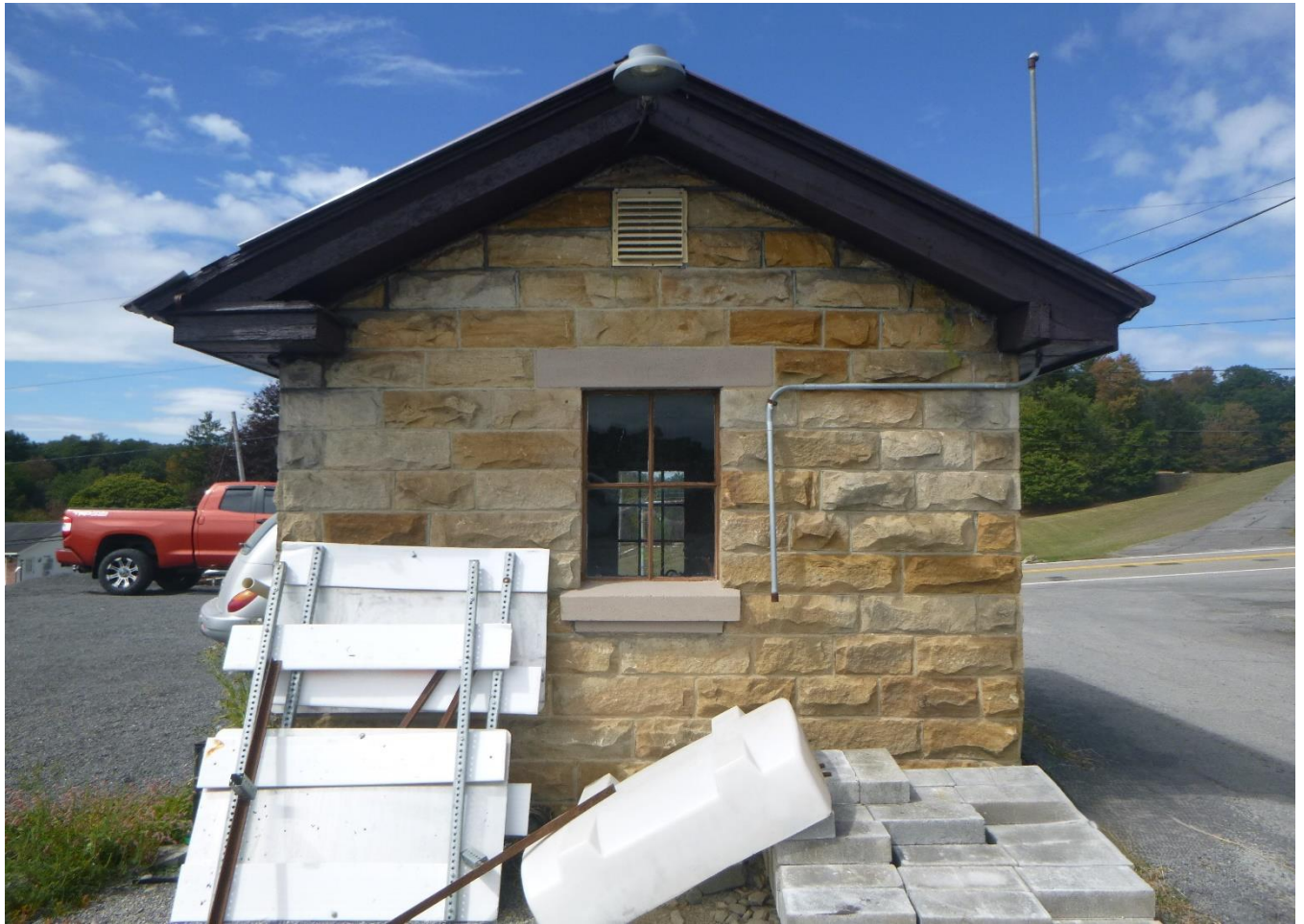
Photo 3 Barbour County Maintenance HQ Shed Barbour County State Route 119 East elevation of storage shed
