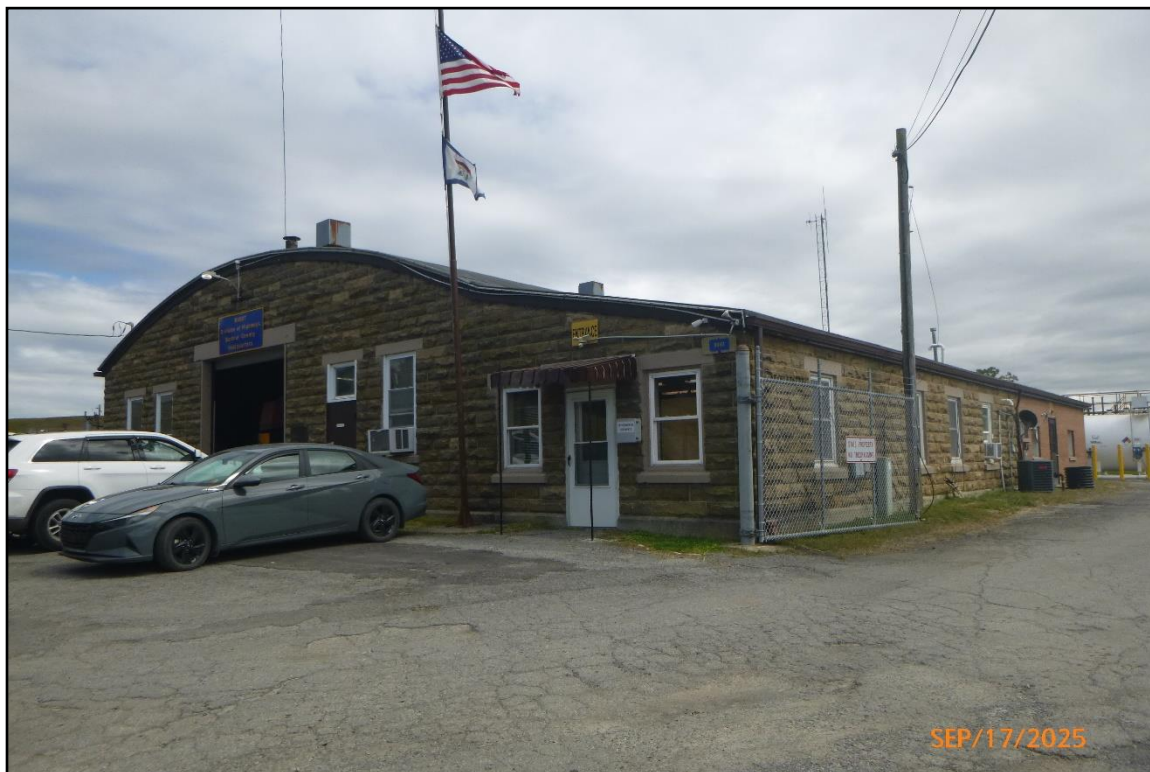
South and west elevation view of BCMH garage and office building.
