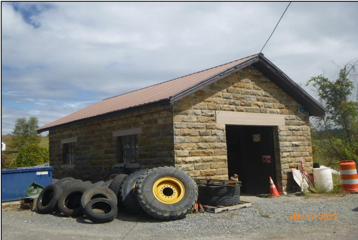
Storage building, west and south elevations.
