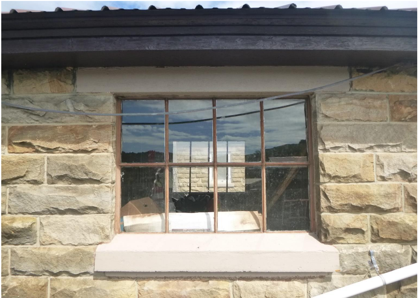
Photo 7 Barbour County Maintenance HQ Shed Barbour County State Route 119 Detail of steel window and concrete sill and lintel on south elevation
