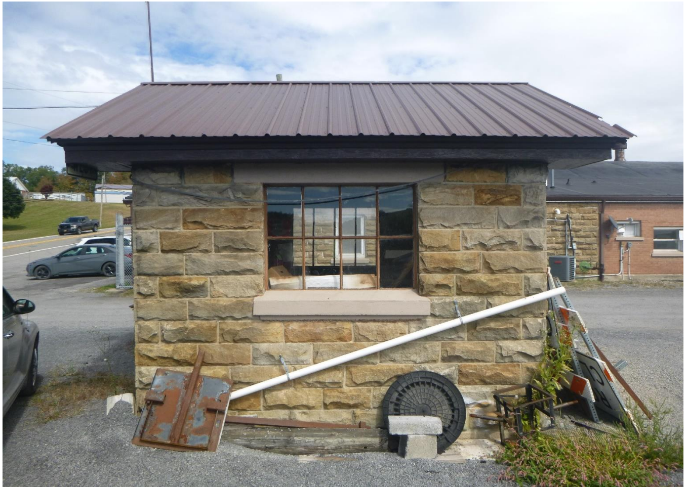
Photo 4 Barbour County Maintenance HQ Shed Barbour County State Route 119 South elevation of storage shed
