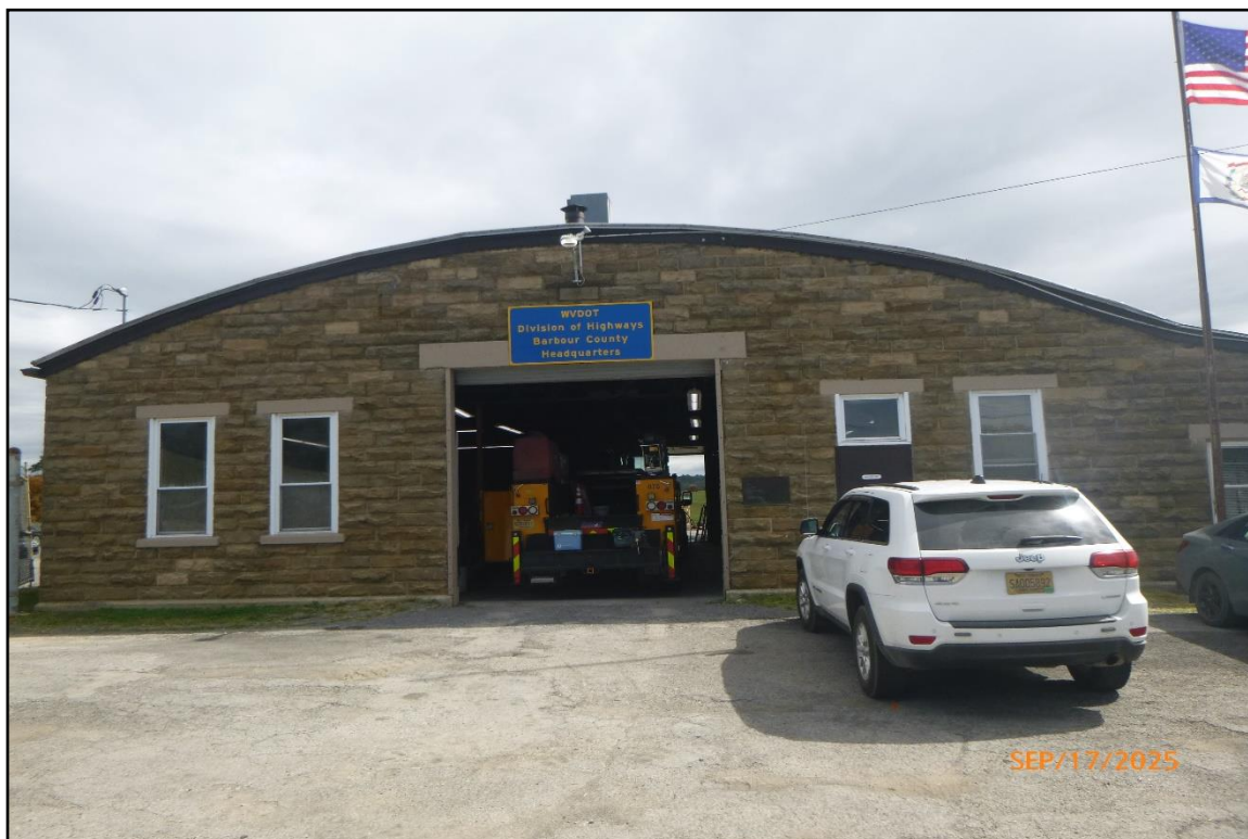
Façade (west elevation) of BCMH garage and office building.
