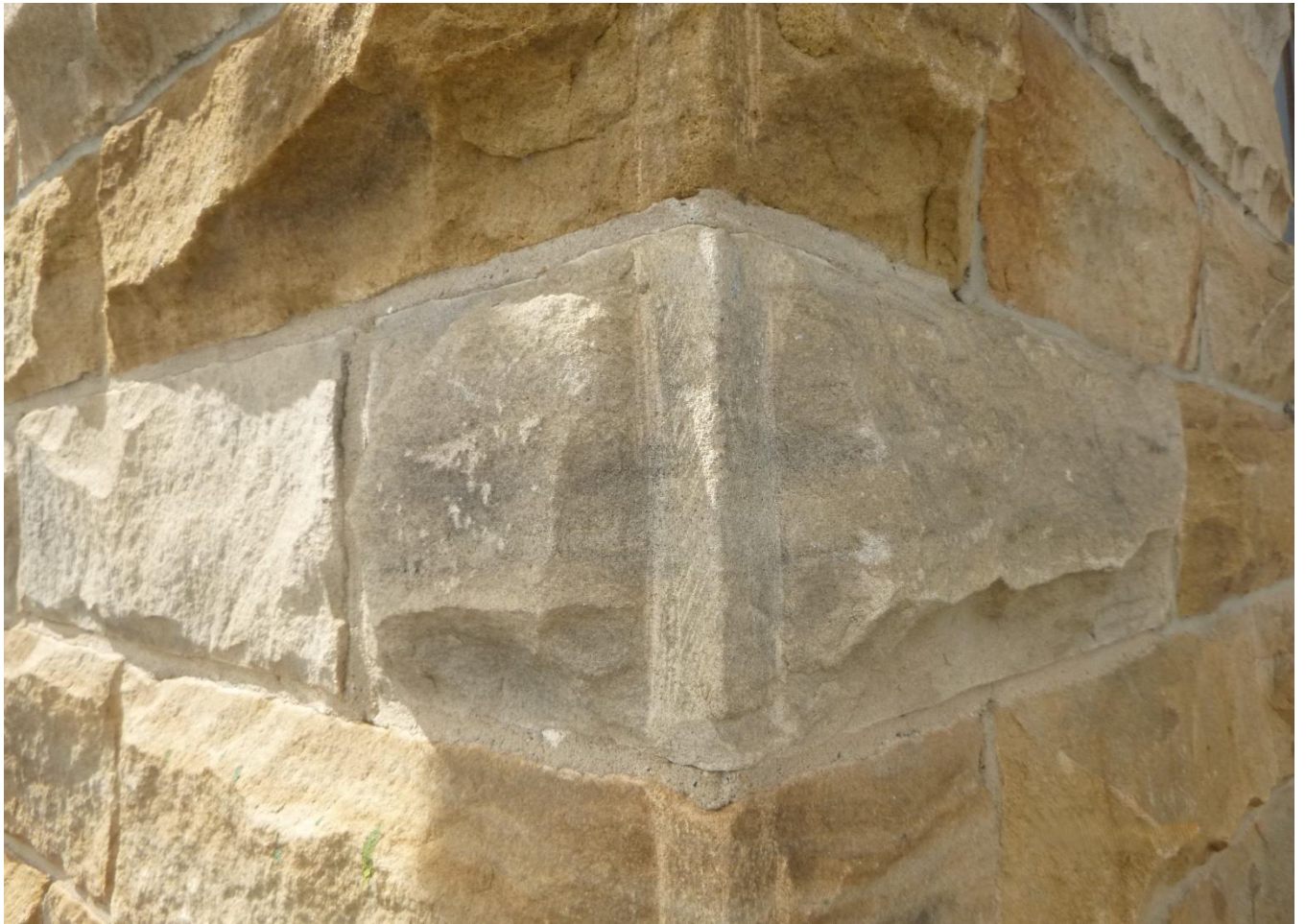
Photo 9 Barbour County Maintenance HQ Shed Barbour County State Route 119 Detail of stone masonry corner
