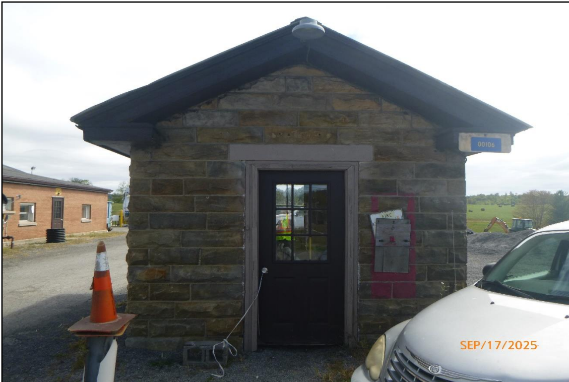
West elevation (façade) of former gas house.
