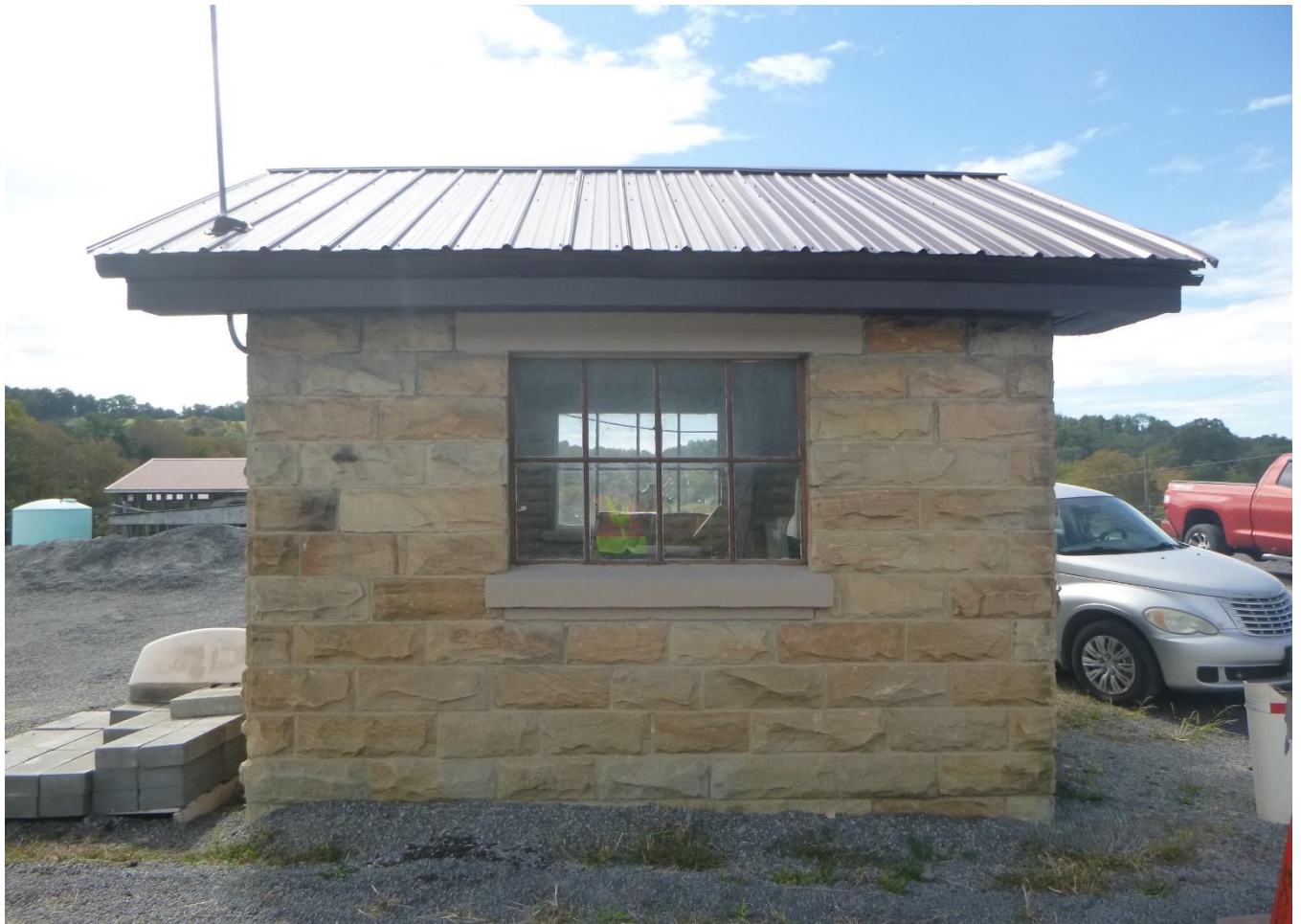
Photo 2 Barbour County Maintenance HQ Shed Barbour County State Route 119 North elevation of storage shed
