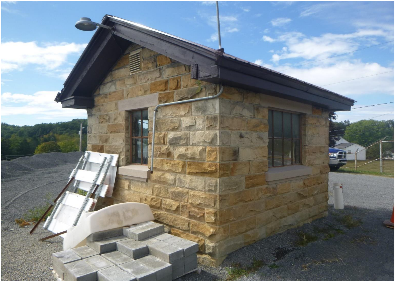
Photo 6 Barbour County Maintenance HQ Shed Barbour County State Route 119 Three-quarter view of shed, view southwest
