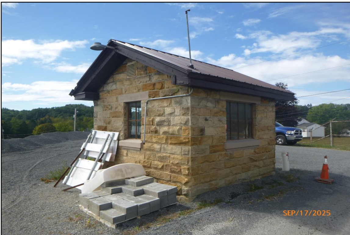
Former gas house, north and east elevations.
