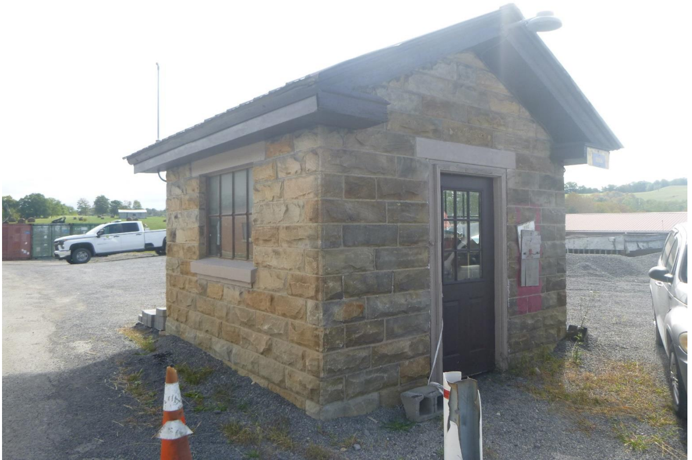
Photo 5 Barbour County Maintenance HQ Shed Barbour County State Route 119 Three-quarter view of shed, view southeast
