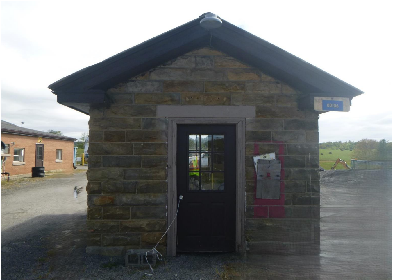
Photo 1 Barbour County Maintenance HQ Shed Barbour County State Route 119 Façade (west elevation) of storage shed
