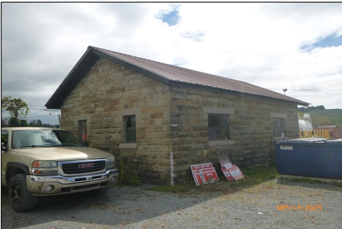
Storage building, north and west elevations.
